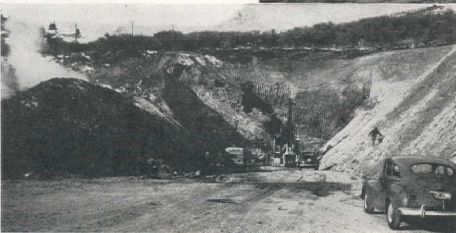
EAST PORTAL CUT , on the Livingston side of Bozeman Pass, in which the grading is complete, left. Early stage of the same excavation showing the equipment in action, above. The bulldozer was especially useful to blade pit free of frozen ruts, thus facilitating efficient truck movement.
