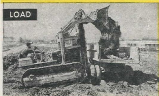
Traxcavator excavating and loading for barracks foundations at an army camp, Indianapolis, Ind.
