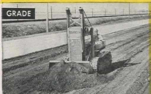
Traxcavator grading between lanes on U. S. Highway 30, near Valparaiso, Indiana.
