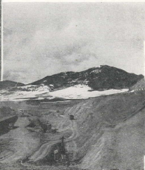
BOZEMAN TUNNEL west portal approach cut showing the excavation nearly complete, left. Power shovels loading five cu. yd. trucks from separate benches of the same cut during early stage of construction, below. Approach excavations consisted of 165,000 cu. yd. of common excavation and 130,000 cu. yd. of solid rock removal.
