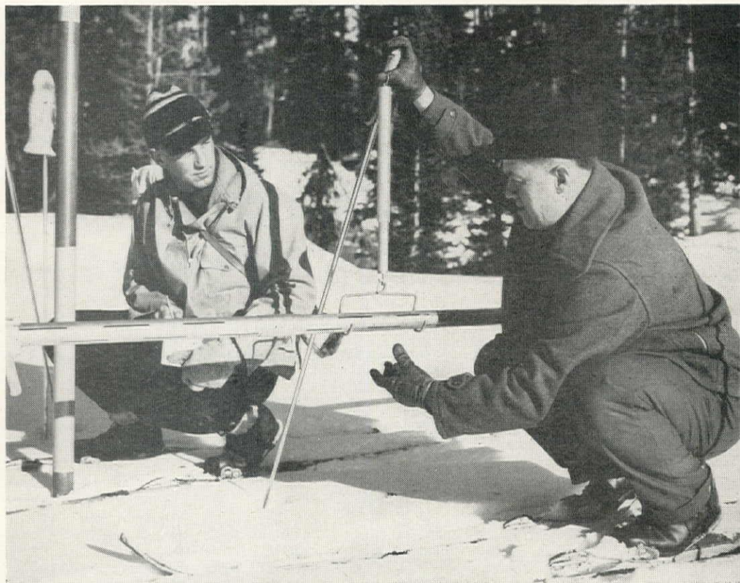
SOIL CONSERVATION SERVICE men take measurements of snowpack as basis for 1945 stream runoff forecast. R. A. WORK, of the Service at Medford, Ore., left, and A. E. KENWORTHY, forest ranger at Anthony Lake, Ore. Snow-sampling apparatus includes tube with vision slits, hand scale with holding cradle, and marker pole.
