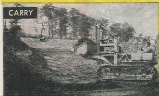
Traxcavator preparing right-of-way for a cross-country pipe line in Illinois.
