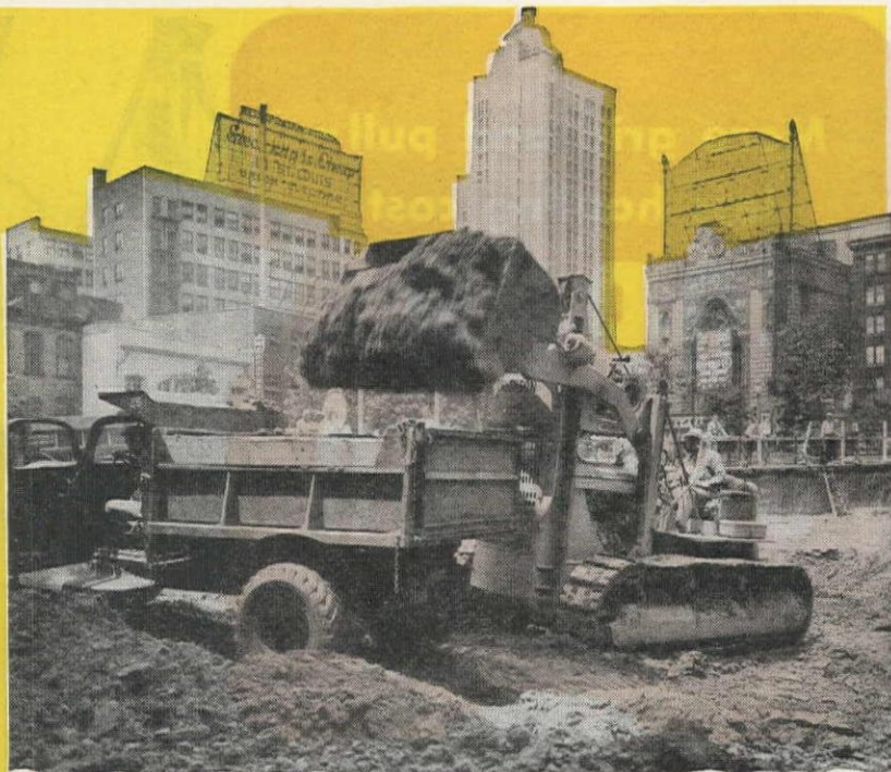
Traxcavator digging up old street surfacing in a Virginia town.
