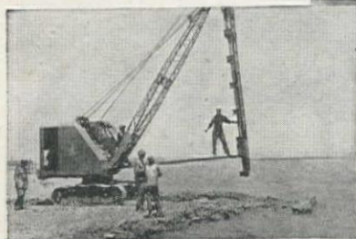
Osgood "20" driving piles for a landing pier in North Africa.
