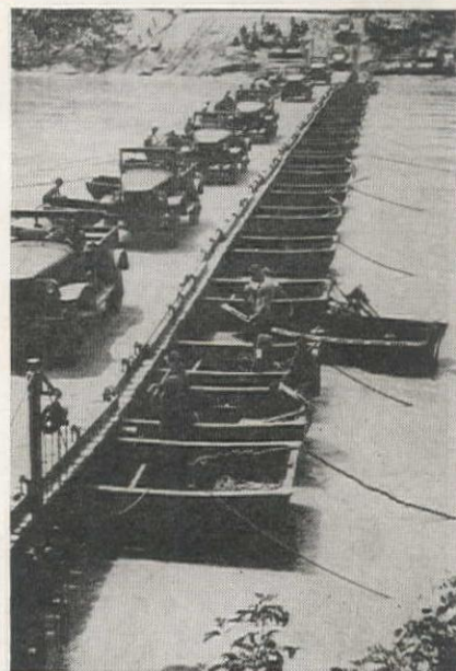
MILITARY VEHICLES using a modern ponton bridge during operations in the Italian campaign. Boats can be put into place by outboard motors in quick order, and deck, cut of standardized timbers, attached in short space of time.
