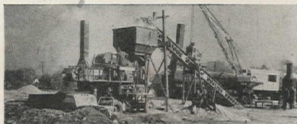
For Intermediate Mixes— The B-G Mixer Is Teamed Up With a Dual Drum Dryer
