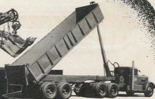
Steward & Nuss, Fresno, operate such Fruehauf Dump Trailers. Capacity 25 tons.
