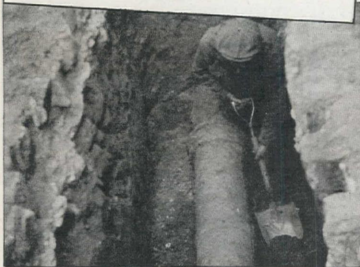
[Here is America's oldest cast iron water main, now in its 124th year of continuous service in the water distribution system of the city of Philadelphia.]
