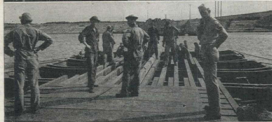
CONSTRUCTION OPERATIONS on a modern ponton bridge. Top, "balk" or bridge stringers, held in place with clamps, while 5-ponton section is moved into place. Bottom, timber balk being laid on top of a span of pontoons, with the deck planking, which is called "chess" on top of it. Overall width of the planked roadway is 15 ft.
