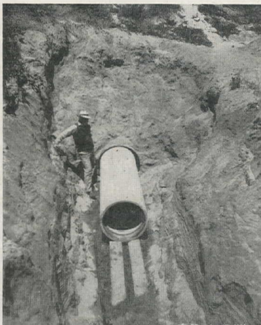
Inserting the 24" Concrete Cylinder Pipe Through Casing
