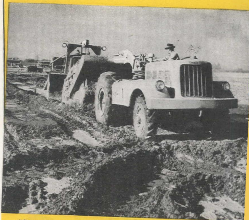
"Caterpillar" Diesel DW-10 Tractor with 8.5-yard scraper being pushdozer loaded with "Caterpillar" D8 Tractor on a muddy Army airport in California.
