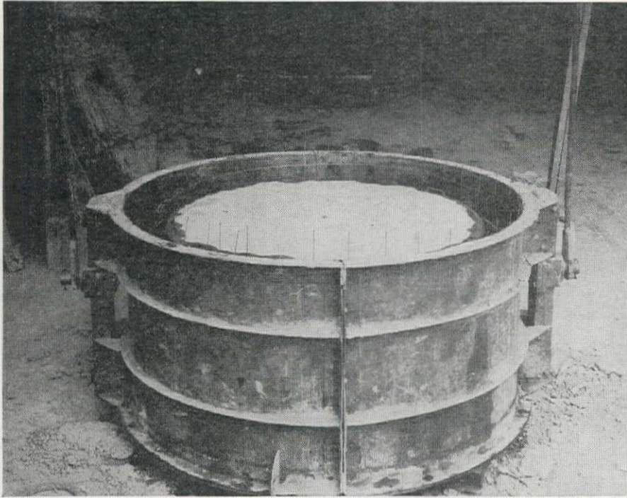
STEEL PLATE MOLD for 500-gal. tank with welded steel mesh reinforcement in place in preparation for pouring. Tank is poured bottom side up and immediately turned over (note trunnions) on clamped pallet to permit concrete to settle toward floor.
