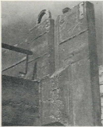
LIFTING LOOP on precast forms for tremie concrete slab showing strut-tie connected to side wall of form.
