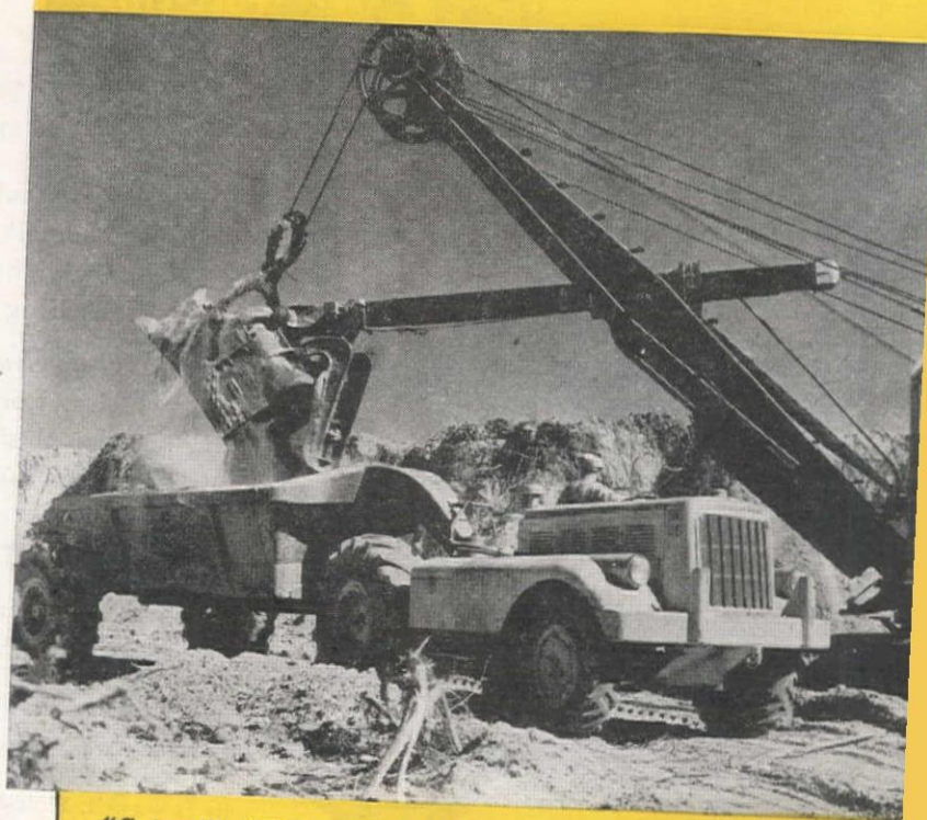
"Caterpillar" Diesel DW-10 Tractor and 8.3-yard W-10 Wagon hauling from shovel on a railroad job in Maryland.
