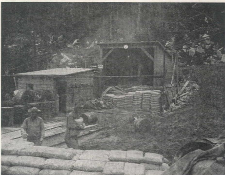
A 50-TON MINE HOIST rigged up by Seabees at the top of a 750-ft. inclined railway used for supply of equipment, materials, and supplies to an Alaskan coast defense project. Seabees practice jobs they knew in civilian life, at same time ready to fight.
