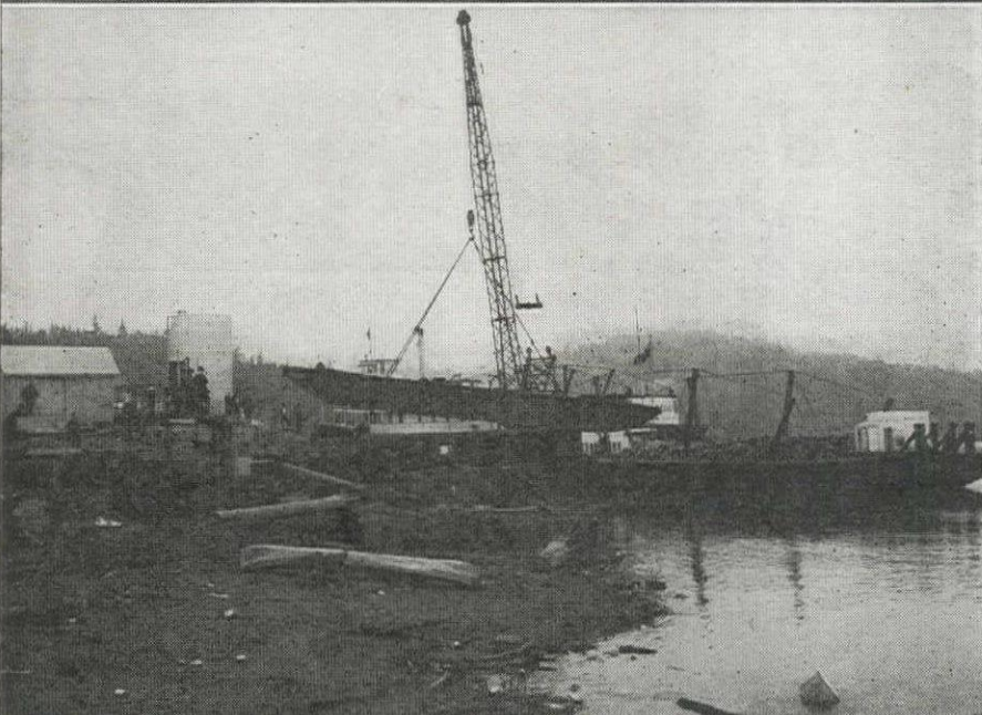
DURING THE SUMMER of 1942, materials for the Canol pipeline were hauled by water from Waterways on the Athabaska River to Canol camp on the Mackenzie. Barges used in this voyage were constructed in a shipyard at Waterways (upper). Between Fitzgerald and Fort Smith, it was necessary to portage around 16 mi. of rapids. Barges were lifted bodily out of the water (bottom), pulled across portage road by tractor (middle).
