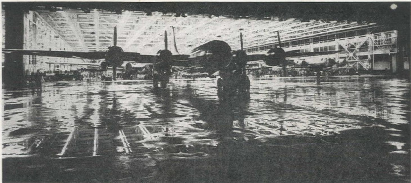
NIGHT VIEW of a completed B-29 ready to be moved through one of the 300-ft. door openings of the Renton, Wash. plant of the Boeing Aircraft Co., to the flying field outside. The complete operation of opening a set of doors requires 2 min.
