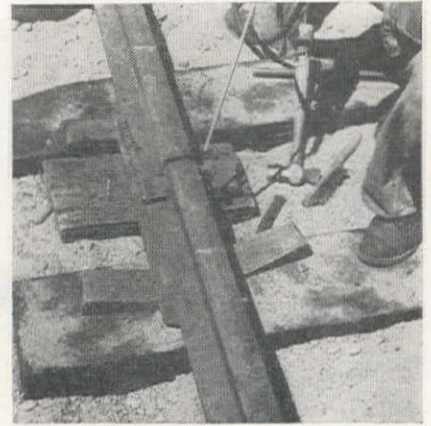
BASE PLATE is wedged up to rails after tops of rails are lined up. Welds are peened and brushed to remove scale.
