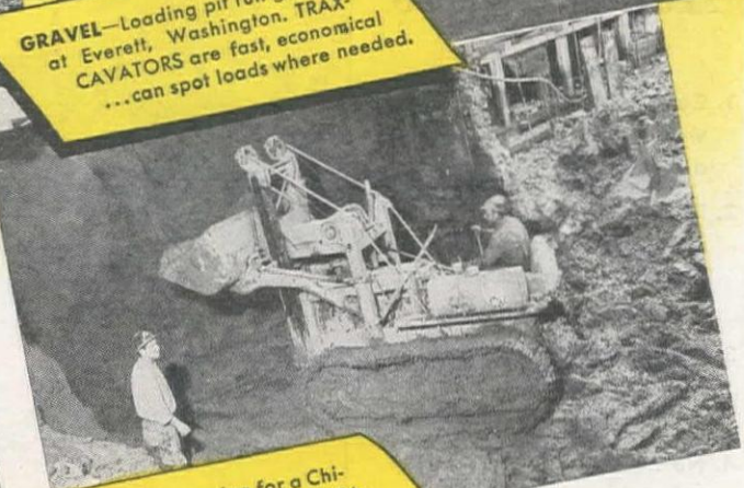
SUBWAY —Excavating for a Chicago subway station. TRAXCAVATORS get high production even in awkward, close quarters.
