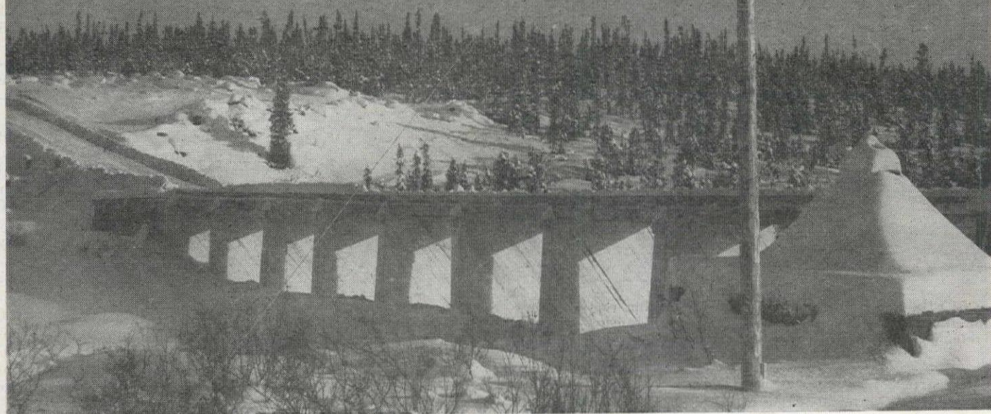
BRIDGE OVER the Macmillan River on Canol Road is blanketed with snow. Telephone line will be used in operation of pipeline. Piling covered with sheathing for winter protection.
