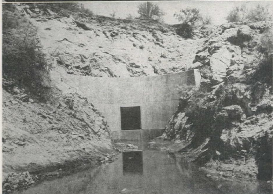
PLYWOOD FORMS (upper) being built for curved intake section. Intake gate tower, 108 ft. high will surmount this opening. Outlet rectangular section (lower) is 7x8 ft. Transition from 12-ft. diam. arch section of main tunnel is made in last 23 ft.
