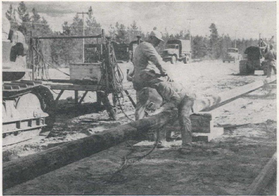
WELDING CREW working on 6 in. line from Whitehorse along the Alaska Highway. Tractors pull sleds carrying portable welding machines. Equipped with side booms, they raise and lower the line from blocks to facilitate underside welding.
