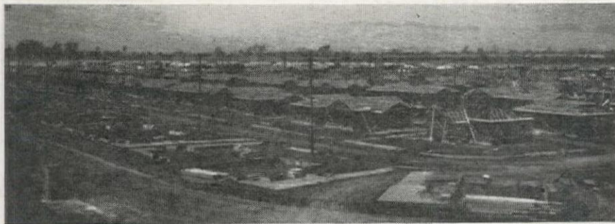
HOUSES in various sections are seen to be in the same stage of construction. Crews have certain types of work to do, follow each other up and down the rows of houses. The village is to consist of 1329 homes and a complete business and civic center.
