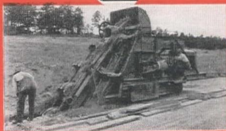
Sewer extension with a Model 160.
