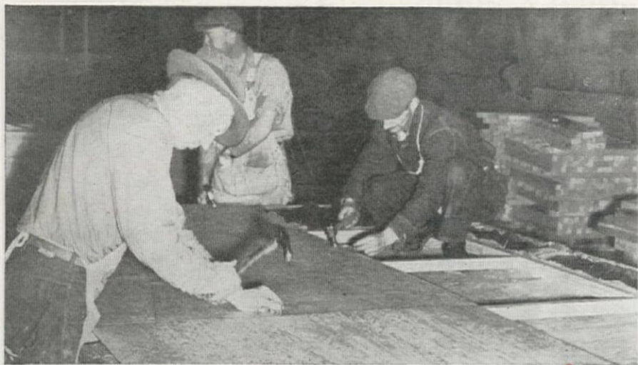
CARPENTERS BUILD wall panels on benches in sub-assembly building. Outside wall panels are insulated and wired before application of final plywood finish surface.
