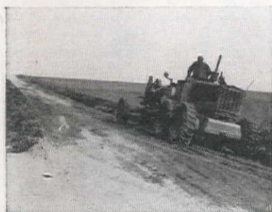
"Caterpillar" Motor Grader cleans out ditches.
