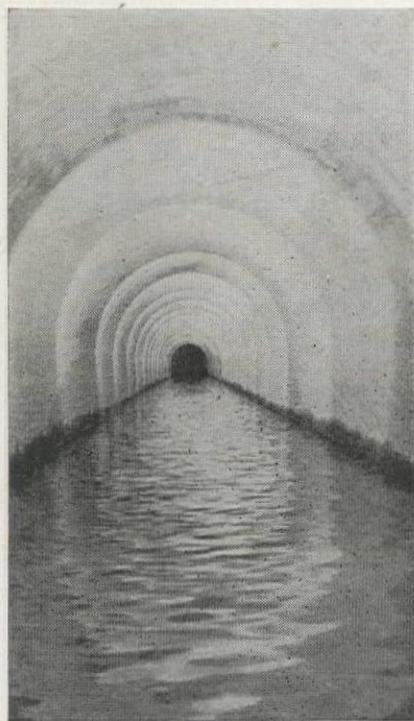
THE TUNNEL after being cleaned and lined. Original alignment was good and walls had suffered little disintegration.
