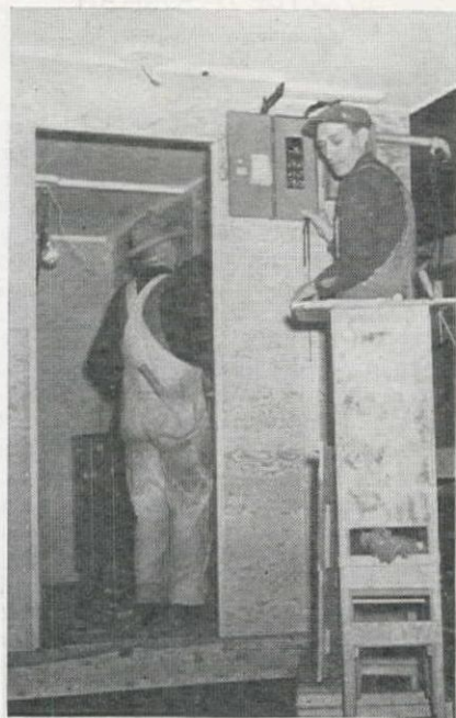
ELECTRICIANS in final assembly, connect panel wires and install pre-assembled switch and meter units. Wiring for modern electric appliances is installed in sub-assembly building while panels are being fabricated.
