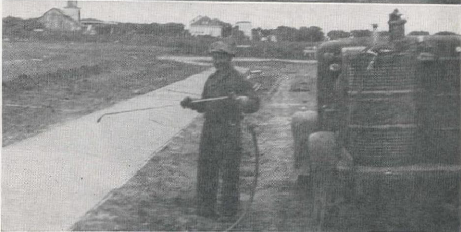
A TRACTOR (upper) pulls a machine, built on the job, to grade and roll the ground in preparation for pouring concrete sidewalks and rounded curbs. Concrete is mixed (middle) in Mixermobile machine and transported to each job in three-wheeled buggies. In order to prevent the evaporation of moisture from the freshly poured concrete, a paraffin seal-coat is sprayed (lower) on concrete surfaces as soon as they are finished.
