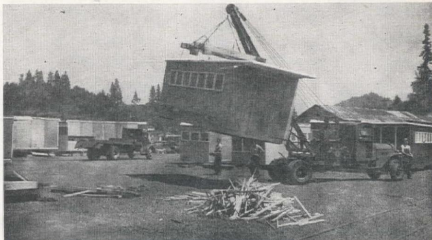
POWER EQUIPMENT solves heavy lifting problem. "Cherry picker" mobile derrick lifts two-bedroom house to be loaded on truck in background and taken to building site. Prefabricated sections in this storage yard will be assembled into housing units.
