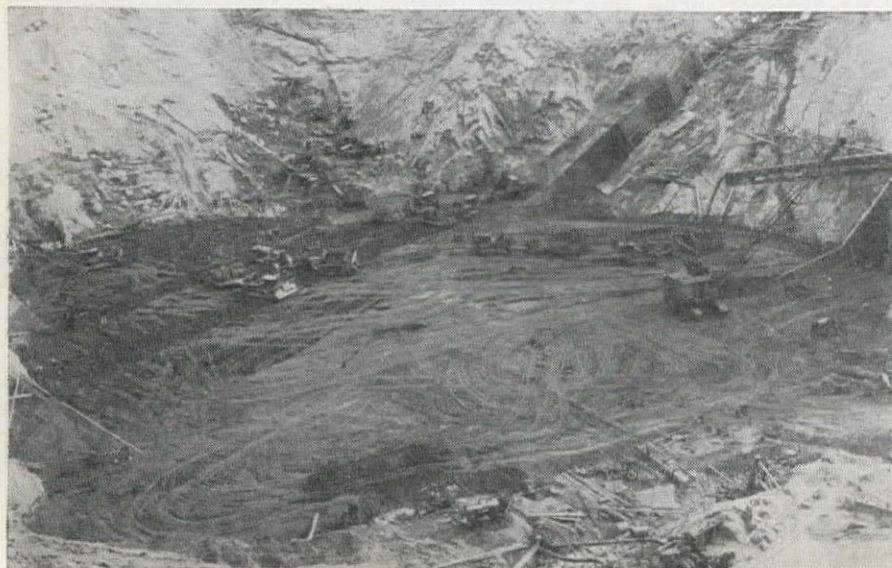
BACKFILLING OF CUT-OFF trench in progress about 30 ft. above the bottom of the excavation. Material discharging from the conveyor belt is from Dixie pit, located 1\frac{1}{2} mi. downstream and 1,200 ft. above the dam. Concrete cut-off walls are visible.
