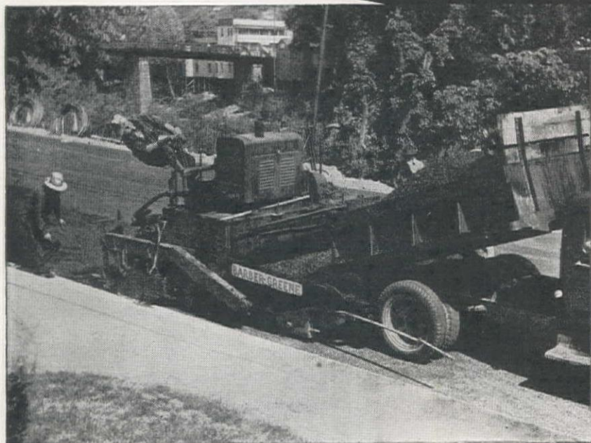
Left: B-G Asphalt Finisher laying top course even with top edge of gutter.
