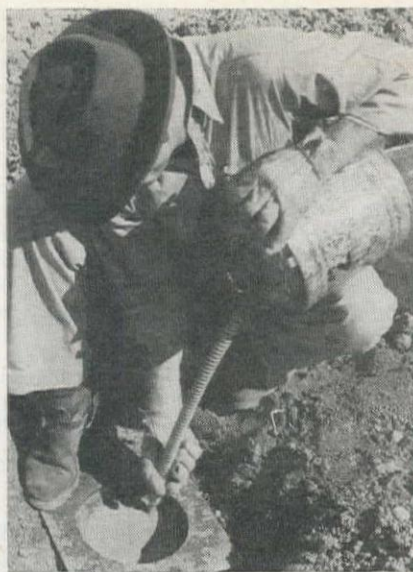
SOIL TECHNICIAN taking a density test in the compacted embankment. Sand of known density is being used to determine the volume of the hole from which a sample has been taken. Sufficient tests are made to insure control of moisture and compaction in the rolled earth embankment.
