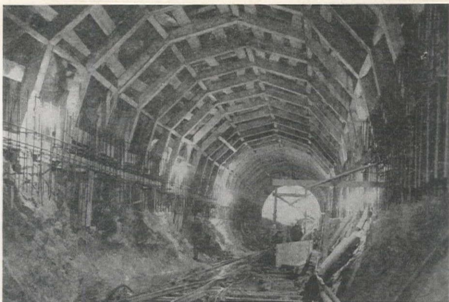
BECAUSE OF THE STEEL shortage, timber supports were placed in the downstream section of the 24-ft. tunnel. This framework supported the excavated tunnel until the reinforced concrete lining was poured. The finished inside diameter is 20 ft.
