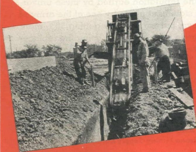
Top: "Digging Wheel" Buckeye trenching for steam mains at a Naval Base. Center: Model 12 Buckeye trenching for telephone cable near airport. Above: Fast, compact "boom type" Model 410 digs trench for water main in Michigan. Left: Model 120 "boom type" Buckeye trenching for drainage, sewage, water, gas, steam and electric cable at new Veterans' Hospital, Hines, Illinois.
