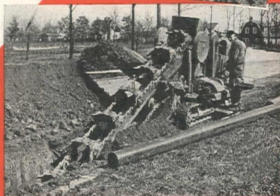
Top: "Digging Wheel" Buckeye trenching for steam mains at a Naval Base. Center: Model 12 Buckeye trenching for telephone cable near airport. Above: Fast, compact "boom type" Model 410 digs trench for water main in Michigan. Left: Model 120 "boom type" Buckeye trenching for drainage, sewage, water, gas, steam and electric cable at new Veterans' Hospital, Hines, Illinois.
