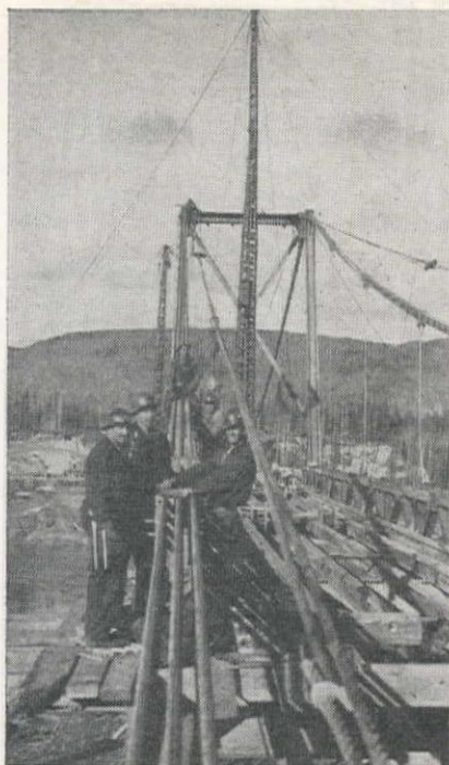
CABLE ERECTION on the Liard River suspension span. The main span is 543 ft. long, towers 94 ft. high. Open style, 12-strand, 2 \frac{1}{8} -in. cables were used.
