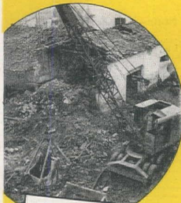
In Italy, a Lorain scoops up debris from a bombed building to clear the way for the advance.
