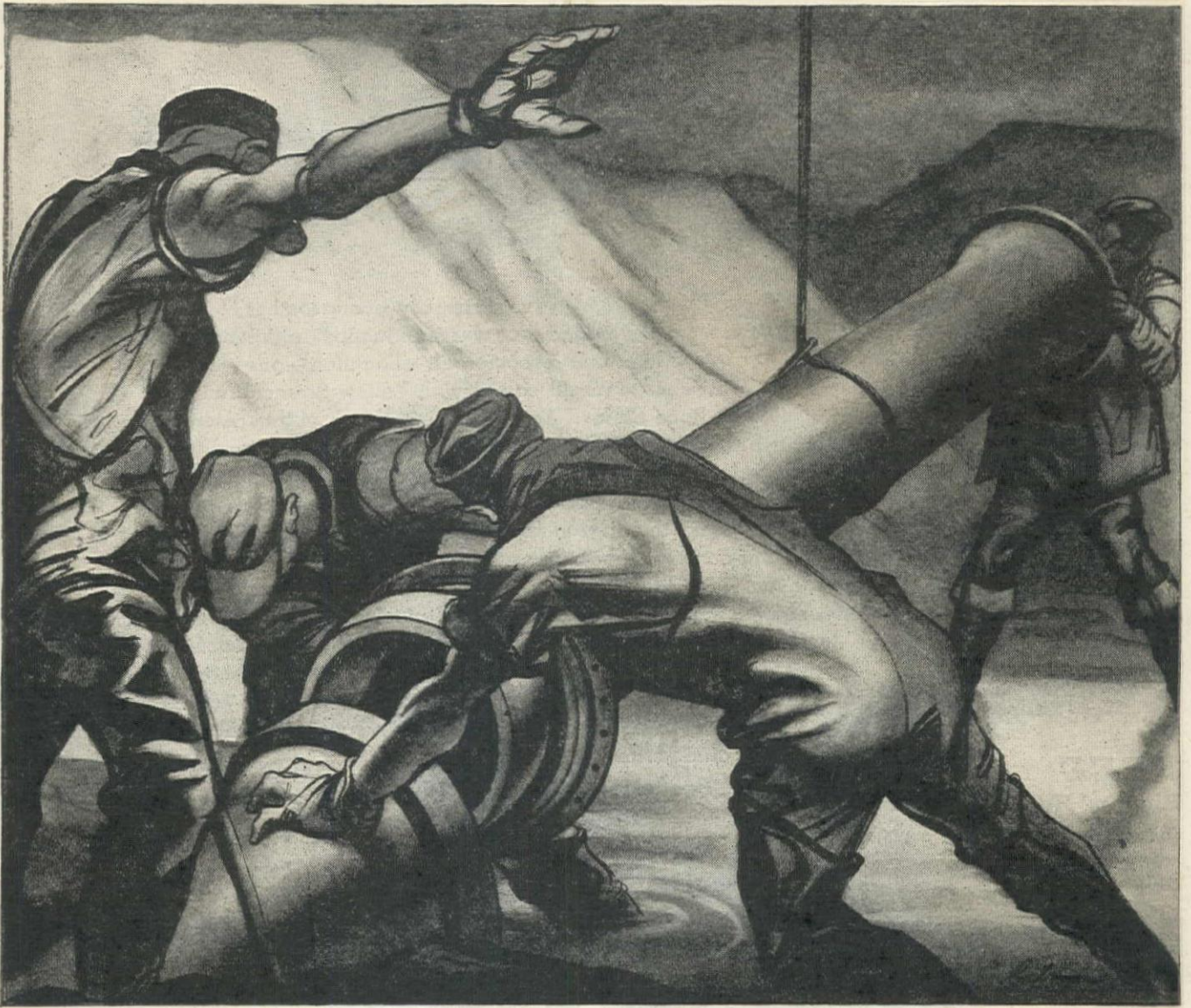
Installing "Usiflex" flexible joint cast iron pipe for submarine crossing. Drawn by Rico Lebrun for U. S. Pipe & Foundry Co.
