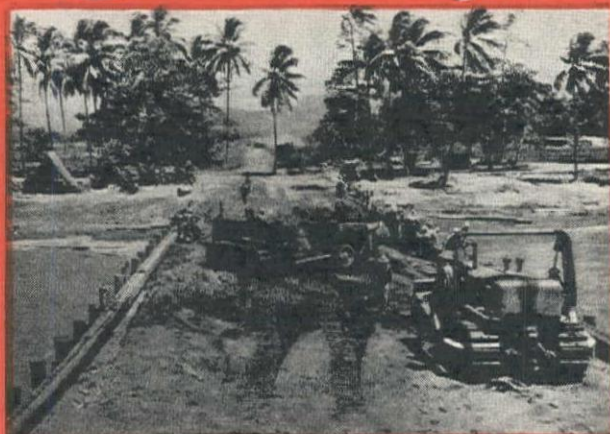
Baker Bulldozer on Allis-Chalmers tractor spreading, leveling and compacting sand on jetty for unloading supply ships; South Pacific.
