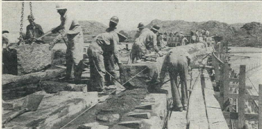
MASONRY PLACING at Altus Dam. TOP , the beds of the granite facing were reduced by a surfacing machine to obtain a 2-in. joint; surfacing time varied from 5 to 15 min. CENTER , the blocks were set by crane after thorough cleaning. BOTTOM , wooden wedges were placed so as to assure proper joint thickness. The back side of block was supported on spalls, an excess deposit of mortar assured well-filled joint.
