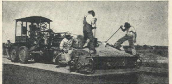
Left—Loading Spreader with chips from truck. Spreader remains hitched to grader.
