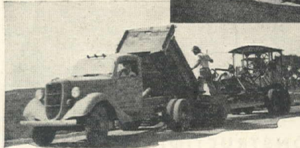
Right—Grader-powered Spreader applying chips in seal coating operation.
