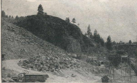
Basaltic cliff near Spokane, Wash., into which the Standard Asphalt Paving Company has tunneled to place Atlas free-flowing explosives in a "single T coyote hole."
