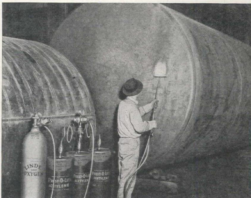
Above an operator is using an Oxweld flame-priming blow-pipe to prepare a large tank for a lasting paint job. The acetylene is from three manifolded Prest-O-Lite cylinders.
