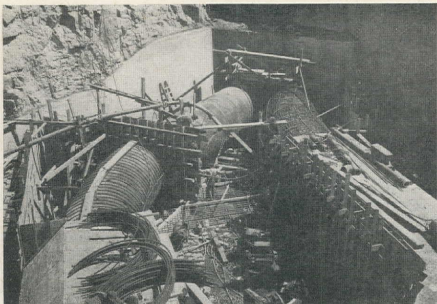
CONCRETE ENCASEMENT of penstocks below tunnel portal. Because much of this work was done in periods of very low temperature, artificial heating with steam pipes, salamanders and electric heaters, was resorted to to prevent temperature stresses.
