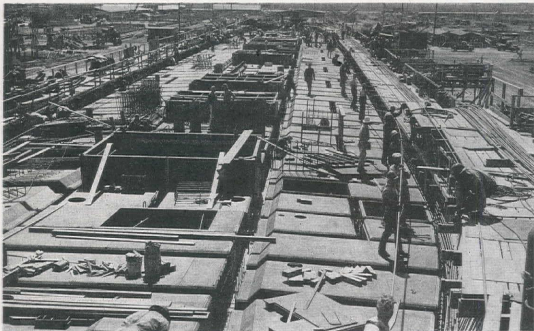
DECK FORMS in place for the third and final pour on a concrete ship at Belair yard, South San Francisco, Calif. Workmen are placing one of the 350-ft. reinforcing bars for the gunwales of the vessel.
