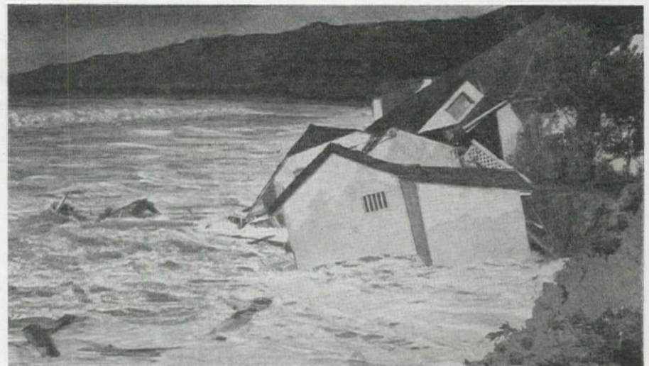
BEACH COTTAGES undermined at Sandyland, Calif., as a result of beach erosion attributable to building of breakwater at Santa Barbara 9 mi. west, and stopping of sand flow.
