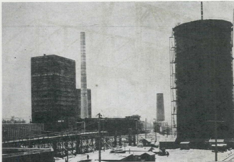
A GAS HOLDER (right) for by-product gases at the Geneva Works plant, and a partial view of the coke manufacturing plant, with coal charging structure in the center and banks of coke ovens extending in each direction and quenching tower at the end.
