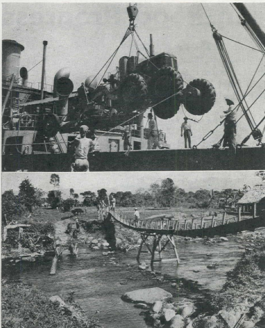
TRANSPORTATION of equipment was one of the most serious handicaps faced by builders of the Pan American Highway. Above, road building equipment being unloaded from transport at Corinto, Nicaragua; below, native footbridge over Mermoso River near San Isidro, Costa Rica, vehicles being obliged to ford. Oxen are hauling timber for new bridge.
