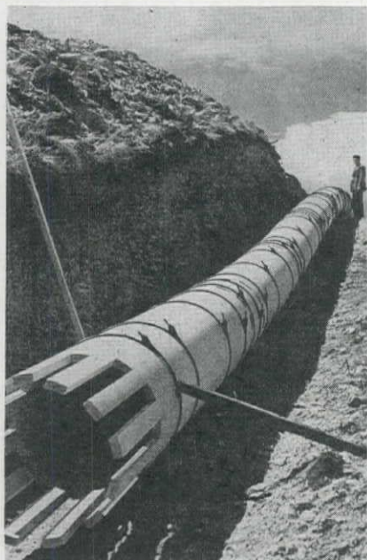
WOOD STAVE PIPE to be used for conveying irrigation water, under construction. The pipe is built to follow the general shape of the ground by using long-radius vertical curves placed in the pipe by shaping and tapering of staves. Photo by National Tank & Pipe Co., Portland, Ore.
