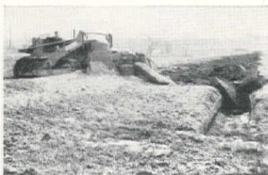
Backfilling a trench in frozen soil with Buckeye Dozer and Winch.
