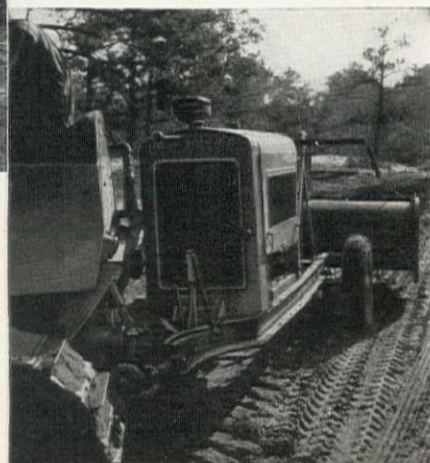
ABOVE: Mixing clay and sand to depth of 12 to 14 inches on experimental project for U. S. Naval Construction Battalions (Seabees). Note fine pulverization and uniformity of mix.
