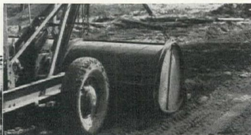
ABOVE: Mixing clay and sand to depth of 12 to 14 inches on experimental project for U. S. Naval Construction Battalions (Seabees). Note fine pulverization and uniformity of mix.
