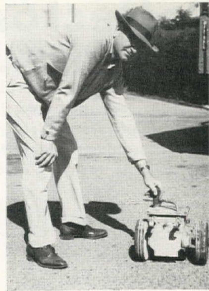
FRANK H. BLAIR , foreman and co-designer of the marking machine, is holding the hopper from which beads feed onto the painted strip. The proper proportion of beads to paint used has been determined from experience in the field.
