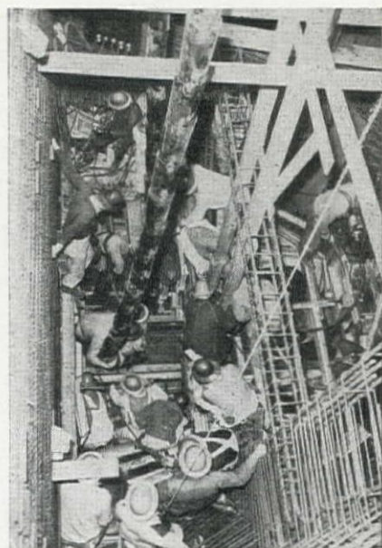
JOINTED swinging chutes enable workmen to distribute the concrete in the bottom of the hull. Air-driven vibrators tamp the concrete to make it dense, watertight and smooth-surfaced.
