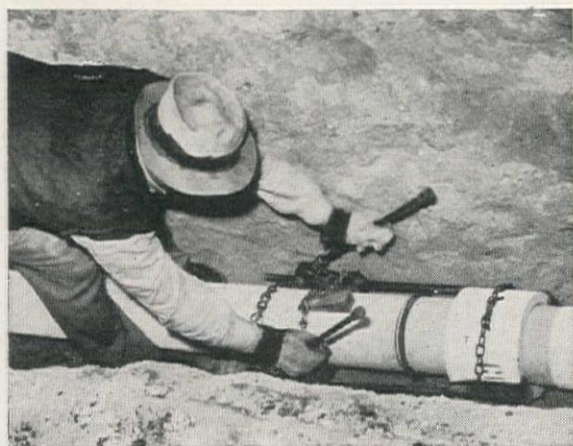
RAPID ASSEMBLY. The absence of hot-poured jointing materials eliminates the necessity of maintaining heating equipment at the trench and makes the assembly of Simplex Couplings a fast, economical operation easily accomplished by unskilled workmen.
