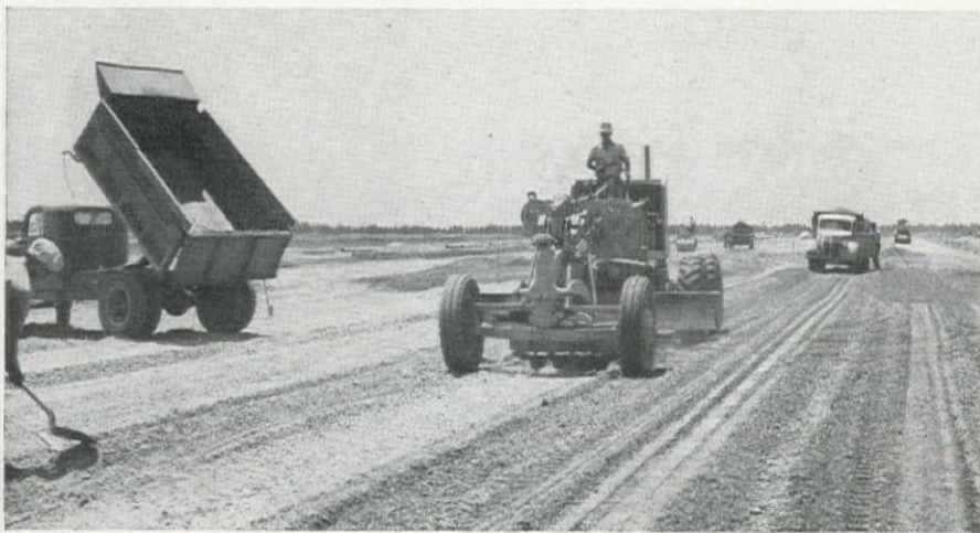
PAVING on flight strips is nearly always of the flexible, bituminous type, and may be laid by either plantmix, roadmix, or penetration methods. Minimum thickness is 2 in.
