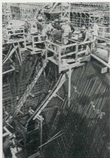
CONCRETE moves from the mixer to the hull in mixer trucks, and is chuted to hoppers inside. Outside plywood shell forms and reinforcing rods can be seen at the right of the photograph.
