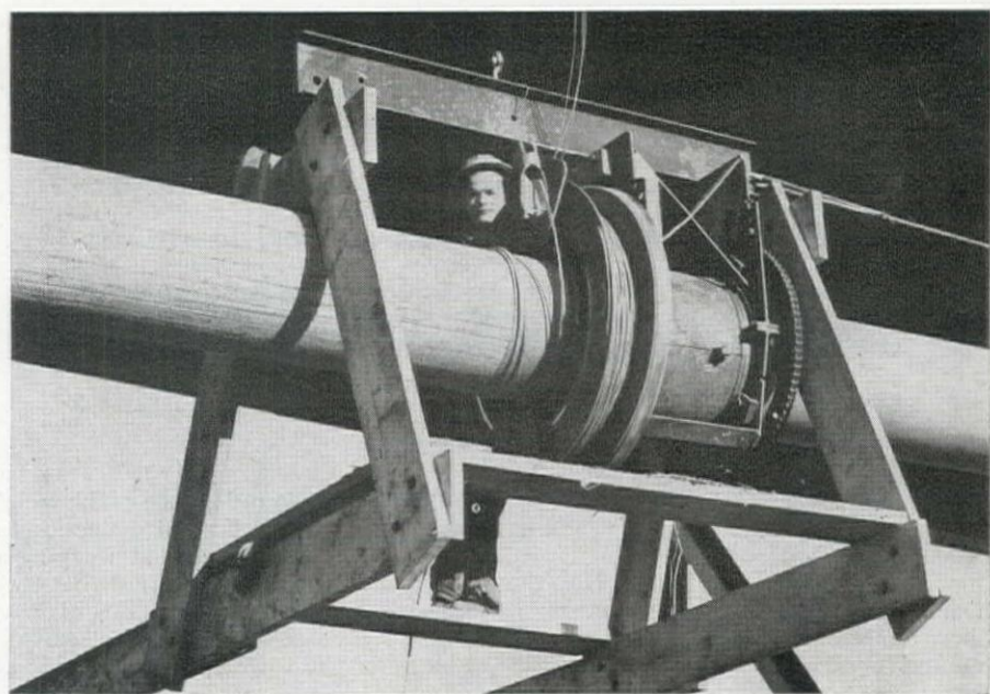
THE WRAPPING wire unwinding rig is shown being operated by "Kelly" Currah at the west end of the bridge under the approach span.
