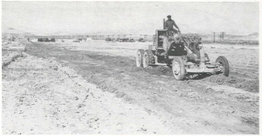
GRADING and preparation of sub-base are important factors in construction of a flight strip, since flexible type surfaces must not be allowed to settle or become pitted.
