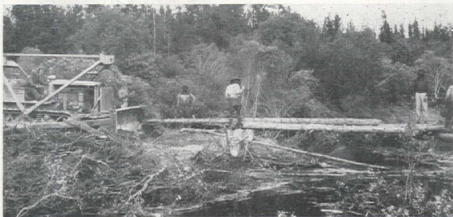
A TRACTOR is used in assembling piles for construction of one of the temporary bridges along the Highway. Mosquitoes present a great problem here.
