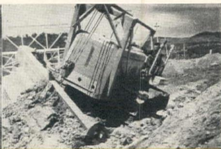
2. Cutting second side of V-ditch. Operator has turned around, leaves Angledozer blade tilted and angled, keeps tractor track in bottom of ditch.
