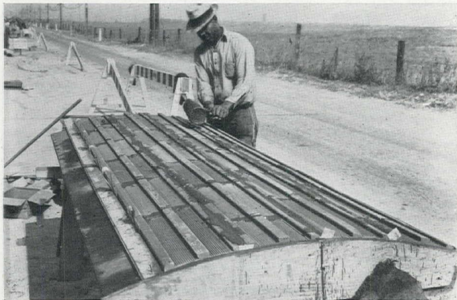
A BITUMINOUS joint compound is being poured into the cracks between tiles after the lining tiles have been made into panels while on jigs.
