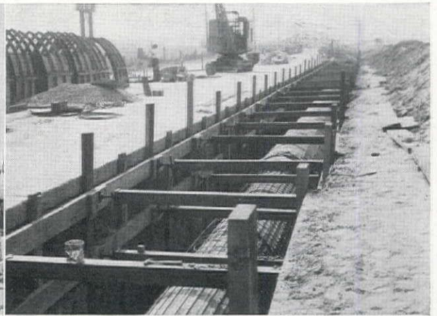
LEFT , a portable I-beam gantry lifting a tile panel into place. RIGHT , shows tile lining in place ready for arch pour.
