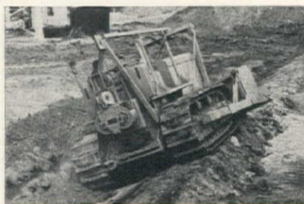
1. Cutting first side of V-ditch. Note how material excavated by lower point of Angledozer blade rolls out under upper track, thus holds machine and blade to a constant cutting angle.
