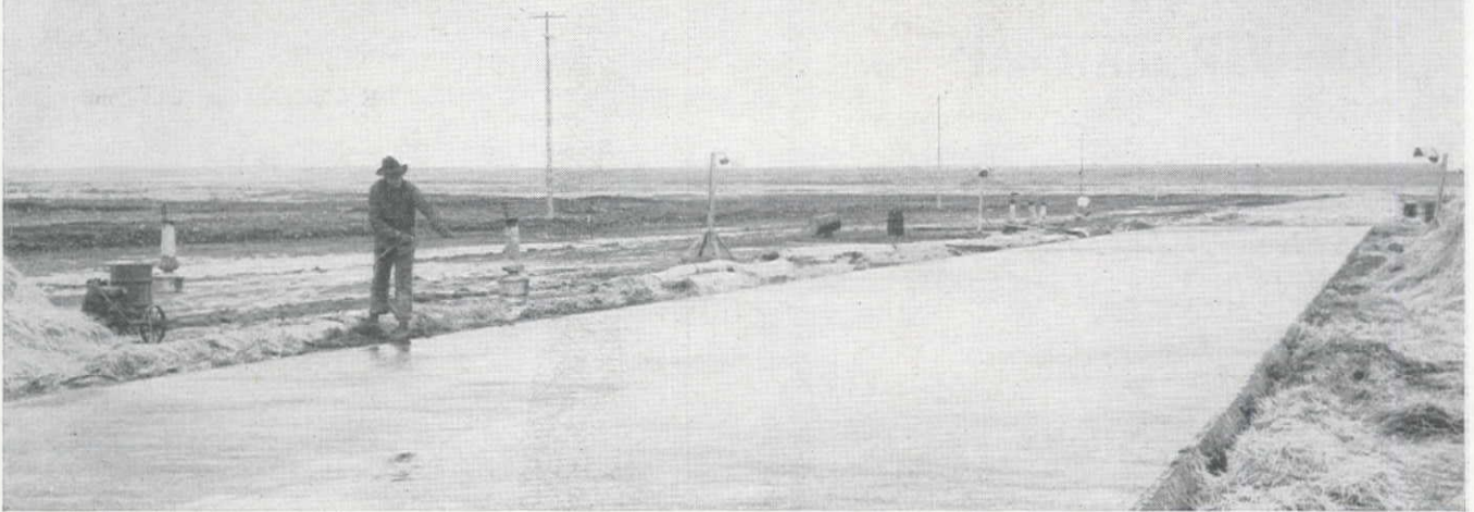
Spraying Hunt Process Curing Membrane on big airport runway in Pacific Northwest that had to be completed despite temperatures as low as 5 degrees. Note ease of application.
