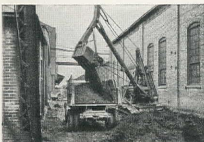
Excavating area between two buildings that will soon be roofed to increase war production. Unit is an A-W Badger.
