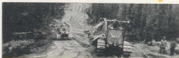
Rugged LeTourneau Dozers, Carryalls and Cranes, used by U. S. Army Engineers and contractors, help punch out 1650-mile Alcan Highway in record breaking time.
