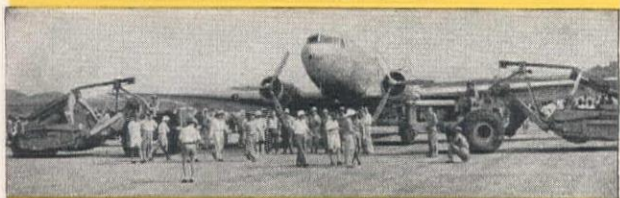
Fleet of 22 LeTourneau units, Tournapulls, Carryalls, Dozers, Cranes, Rooters and Sheep's Foot Rollers, build airports and supply roads in Africa.
