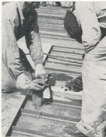
PLACING the top deck of the double steel floor is done after flow tests have shown the floor permits even distribution. Note the separating strips welded to the lower plate.
