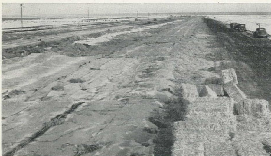
FOUR PROTECTIVE coverings were applied to the green concrete to prevent freezing. A curing membrane was sprayed on, and covered by a layer of paper curing mat. Next was a 12-in. blanket of wheat straw, which was covered by another layer of paper.
