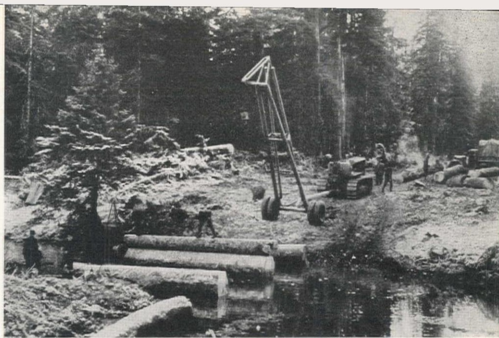
TRACTOR CRANE is used by Army engineer troops to construct a bridge from nearby standing timber across a small creek on the pioneer road. Army construction will be improved and more permanent structures built under Public Roads Administration direction.
