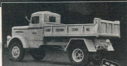
Fleet of Indiana State Highway Commission, equipped with Heil Quality-Built 3 yd. dump bodies with Model DA7-17 Hoists.
