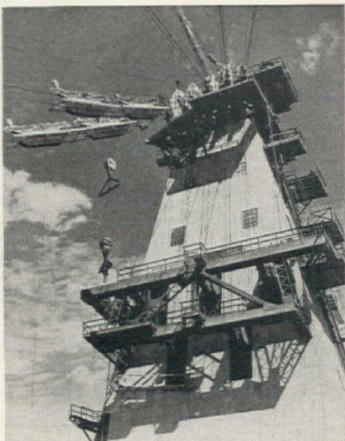
460 foot Head Tower carrying 7 LIDGERWOOD CABLEWAYS on SHASTA DAM
