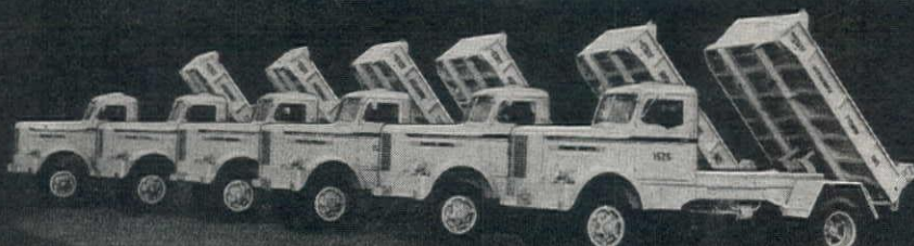
Fleet of Indiana State Highway Commission, equipped with Heil Quality-Built 3 yd. dump bodies with Model DA7-17 Hoists.
