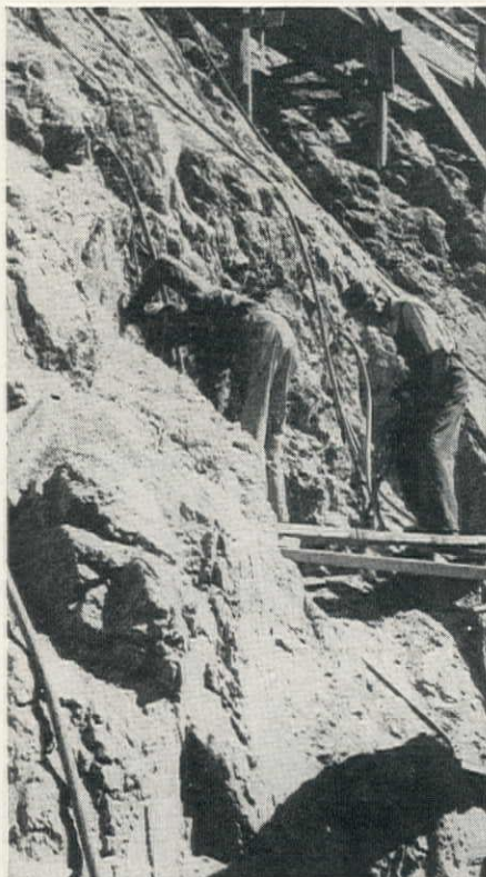
• Preliminary Rock-Drilling for the Power House at the P G & E Pit No. 5 Project, near Redding, Calif. Contractor—H. H. Larsen Co.
