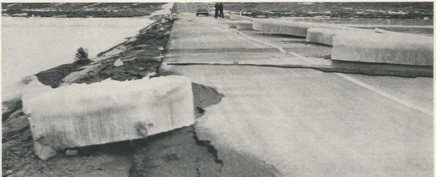
PRACTICALLY ALL THE ICE was deposited between the upstream shoulder of the road and the center line. The cakes were about two feet thick, and as much as 20 ft. square. The roadway was not seriously damaged.
