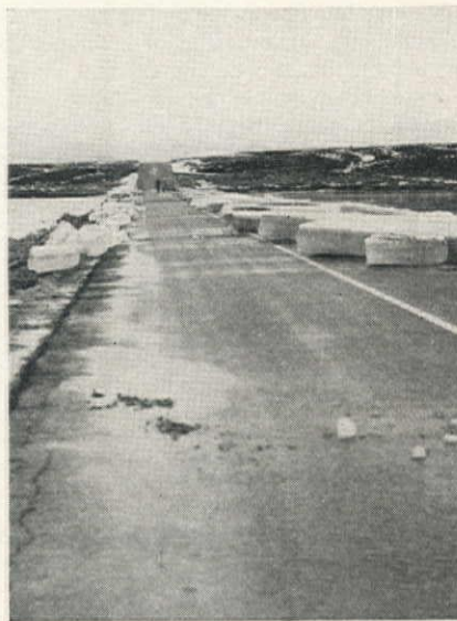
PRACTICALLY ALL THE ICE was deposited between the upstream shoulder of the road and the center line. The cakes were about two feet thick, and as much as 20 ft. square. The roadway was not seriously damaged.
