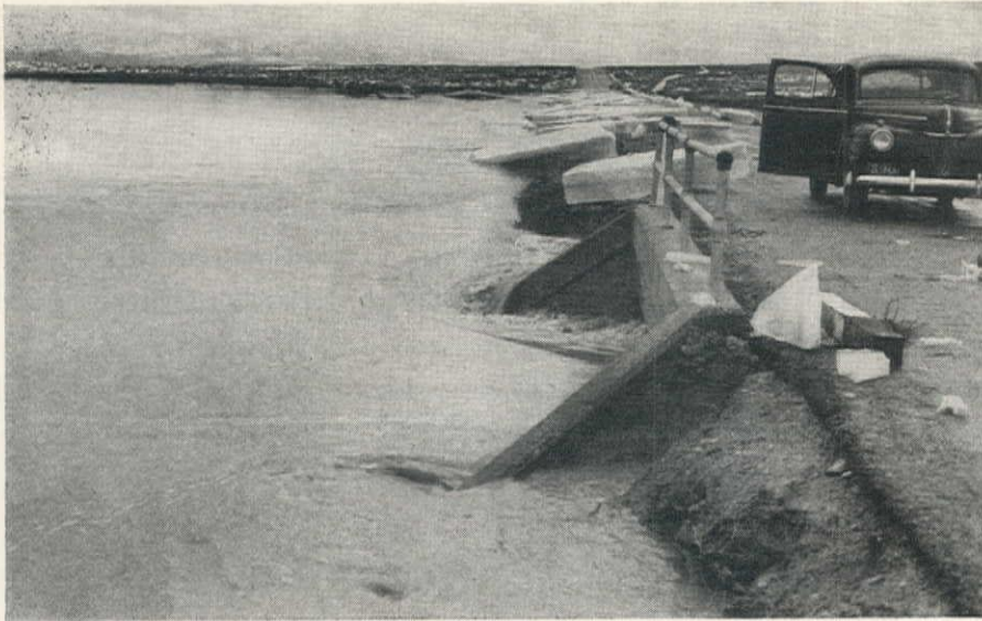
WATER from the wrecked reservoir is shown flowing through the only culvert provided under the highway. At the time of this picture, the crest of the flood had passed, and the culvert was handling the normal thaw flow.
