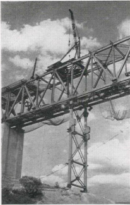
FALSE BENT NO. 6, composed of three panels from suspended span, being dismantled by S-2 traveler, following completion of span 7 above it.
