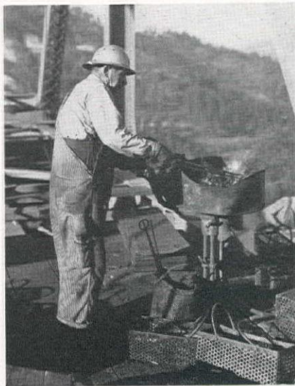
RIVET HEATER operates hand-driven bellows and coke forge high on deck of Pit River Bridge, assuring ample supply of rivets near point of use.
