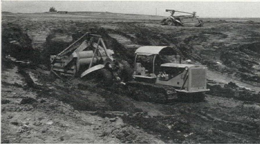
LAKE BEDS were excavated with tractors and scrapers. Drainage systems consisted of 6-in. perforated concrete pipe in herringbone patterns placed in the excavations on a 6-in. layer of crushed rock secured from the rock excavated in other locations.
