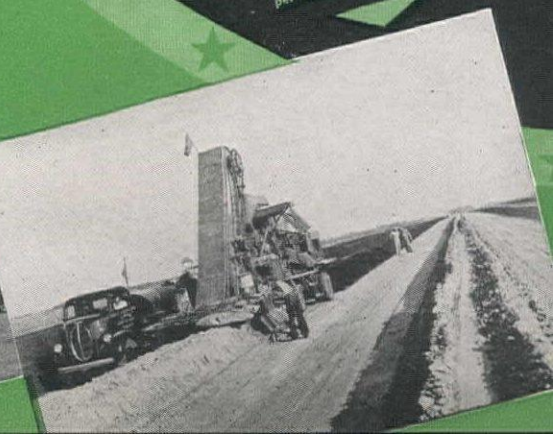
B-G TRAVEL PLANT mixing sand and asphalt for U. S. Navy. It is delivering 3 cubic yards of mixed material per minute in this picture.
