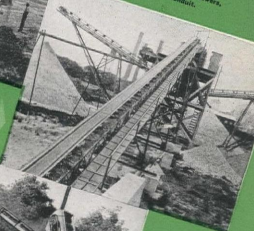
B-G PERMANENT CONVEYORS are being used in many Defense Projects. This is a typical application elevating sand and gravel to a central screening plant and storing the various sizes.
