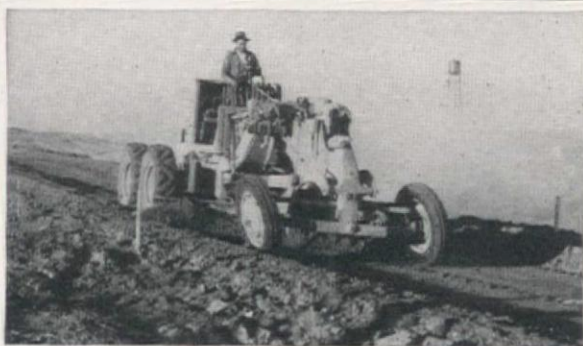
● Adams heavy-duty motor grader builds miles of connecting roads within new ordnance plant in the east.
