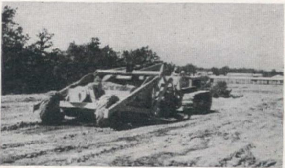
● Adams hauling scraper cuts, hauls and fills to level ground for motor and artillery park in new western camp.
