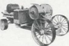
Four Wheel Maintenance JAW CRUSHER with Power Unit
