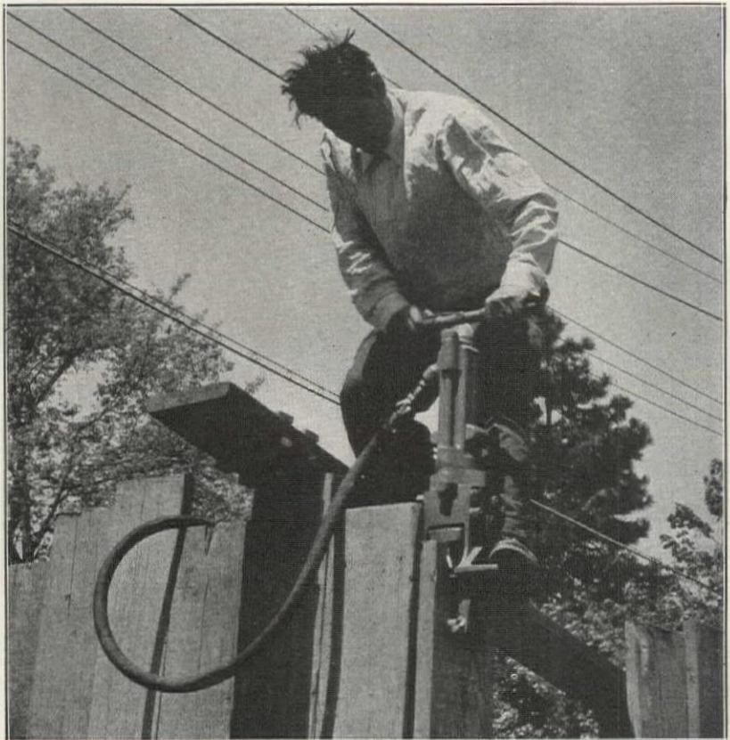
↑ DRIVING 4 FEET per minute in gravel is an easy performance with a CP 116 Sheet-
