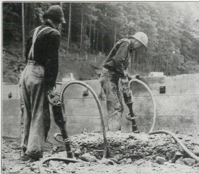
↑ KNOCKING DOWN A BATCH at Cottage Grove Dam with CP Model 417 one-man type Pneumatic Vibrators. Note harsh, stiff mix, with 6-inch cobbles — convincing proof of the power and ruggedness of CP Concrete Vibrators, Pneumatic and Hicycle Electric.
