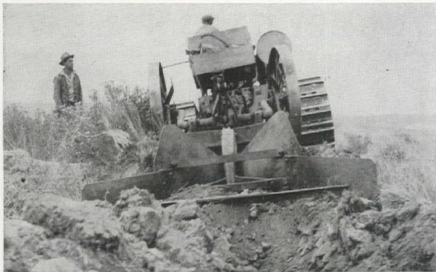
A V-DITCHER with extra wings added to the moldboard and towed by a tractor, was used to uncover the pipe, which had been laid in a 4-ft. trench, with 2-ft. cover.
