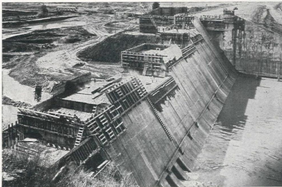
Cottage Grove Dam on coast fork of Willamette River in Oregon. Concrete poured against Fir-Tex Absorptive Form Liner.
