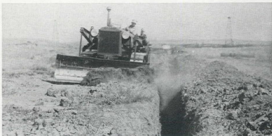
A HOMEMADE BULLDOZER made of two grader moldboards welded together, and set at a sharp angle with the tractor, was used to backfill after the pipe was removed.
