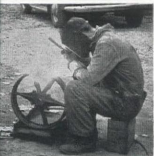
Worn out gears can be rebuilt to last longer than originally with P&H "Harcote" electrodes.
