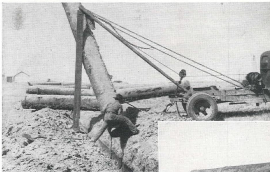
TWENTY-INCH REDWOOD stave pipe was removed after 20 years of service. Above, a section of pipe being pulled out of 4-ft. trench by gin pole mounted on 1½-ton truck with a power winch; right, the sections of pipe were trucked 60 miles to the nearest railroad at Casper, Wyo., for transshipment to Vancouver, Wash.
