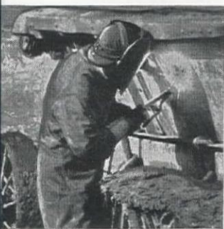
The battered side of this "cat wagon" is put back in shape with P&H electrodes.
