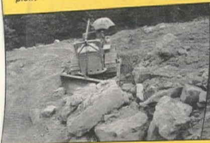
Sidecasting rock on D. B. Hill's highway job, near Huff, Arkansas. Blade can be set straight for bulldozing—no extra bowl to mount. This is but one of three Angledozer Hill is using to handle rock, clay and sand. Two LeTourneau Carryalls handle the longer hauls.
