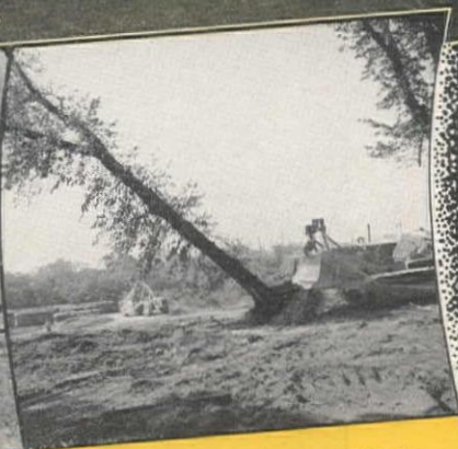
Powerful LeTourneau Bulldozer and "Caterpillar" D8 tractor uprooting full-grown elm trees for public utility in Peoria, Illinois. Upward blade lift can be applied simultaneously with forward tractor shove for added leverage to dig out stumps, trees, boulders.
