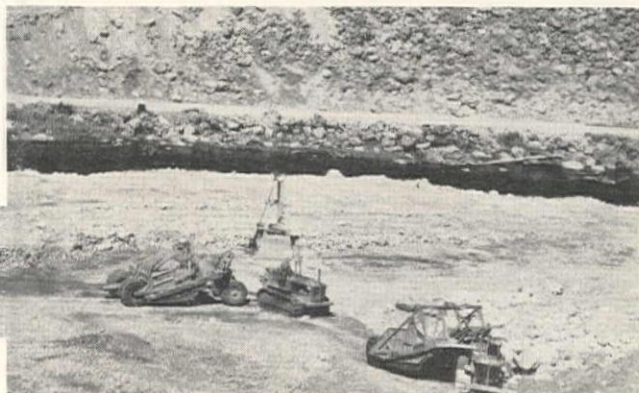
4 of the 5 Wooldridge "3-line" Scrapers operating on the Anderson Ranch Dam
