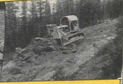
LeTourneau Angledozer clearing stumps and side-hill rock for logging railroad grade, near Shevlin, Oregon. In the logging woods, where work like this is the toughest, LeTourneau 'Dozers outnumber all other makes combined!
