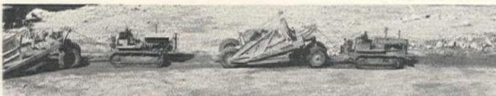
4 of the 5 Wooldridge "3-line" Scrapers operating on the Anderson Ranch Dam
