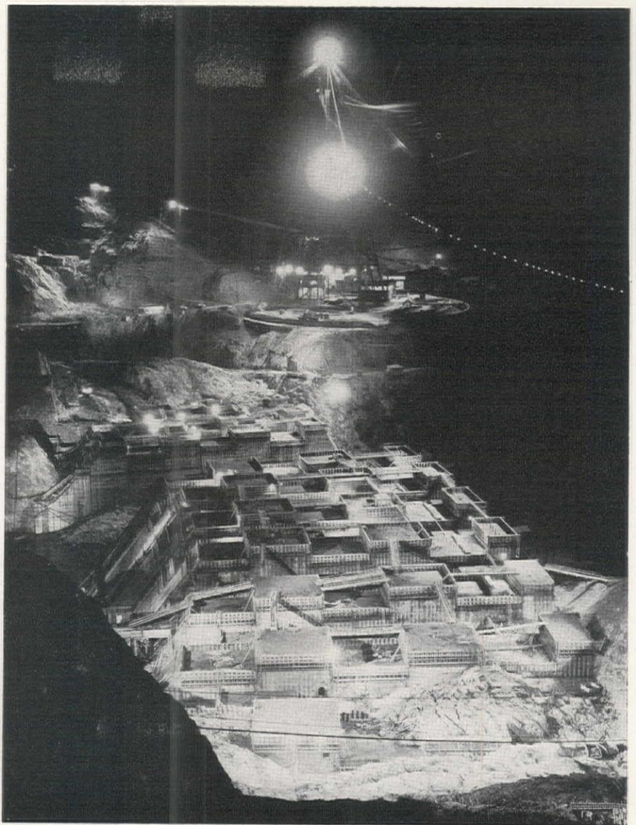
AT SHASTA DAM on the Sacramento River in northern California Pacific Constructors have a total lighting load of about 760 kw. Light intensity at the west abutment averages 10 ft.-candles. Suspended across the dam site on a steel cable are 64 24-in., 1500-watt flood lights with searchlight distribution characteristics. A total of 212 of these units is employed, all with dust-tight covers made of a special heat treated safety glass to prevent injury in case of breakage.
