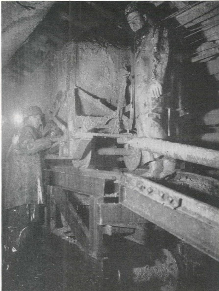
CARS WERE run onto a specially fabricated steel platform over a half-yard concrete pump and the 2-yd. load of concrete successively dumped in four parts.
