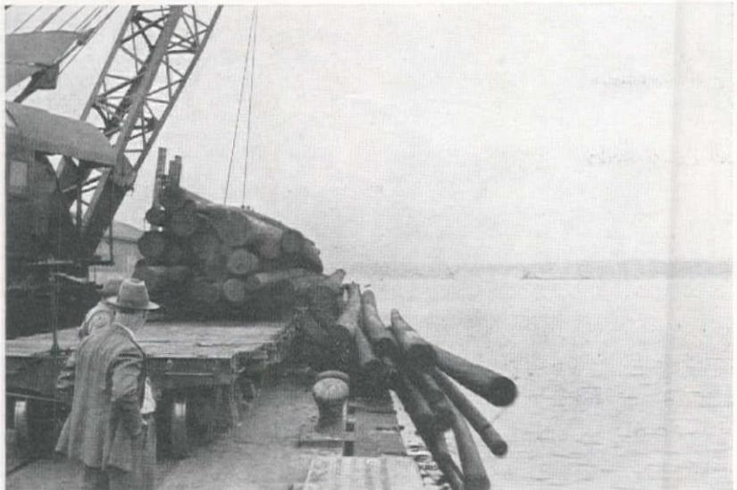
JUMP SKIDS are fastened in place by means of a small metal hook which is placed in the pocket on the side of the car. These piles are 75 and 65 ft. in length. Before this idea was developed, unloading of a car of piling required a crew of five men and occupied about three hours time, each piling being unloaded separately.
