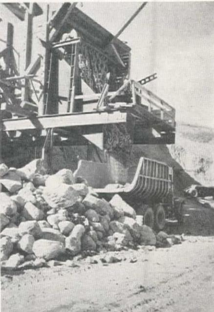
RAW MATERIAL passes over a grizzly which removes 7-in. rock and a secondary vibrating grizzly which removes 3-in. rock. Both oversizes are loaded into trucks at the bottom of the plant to be used in the rockfill and riprap sections.
