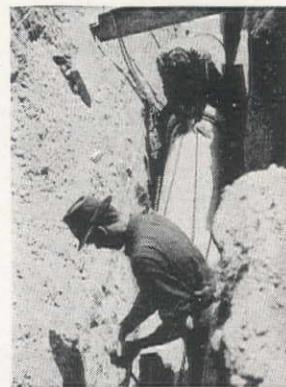
The Simplex Coupling is assembled with a hydraulic puller. The collar engages the edge of the Transite sleeve; the jack fits over the open end of the pipe.
