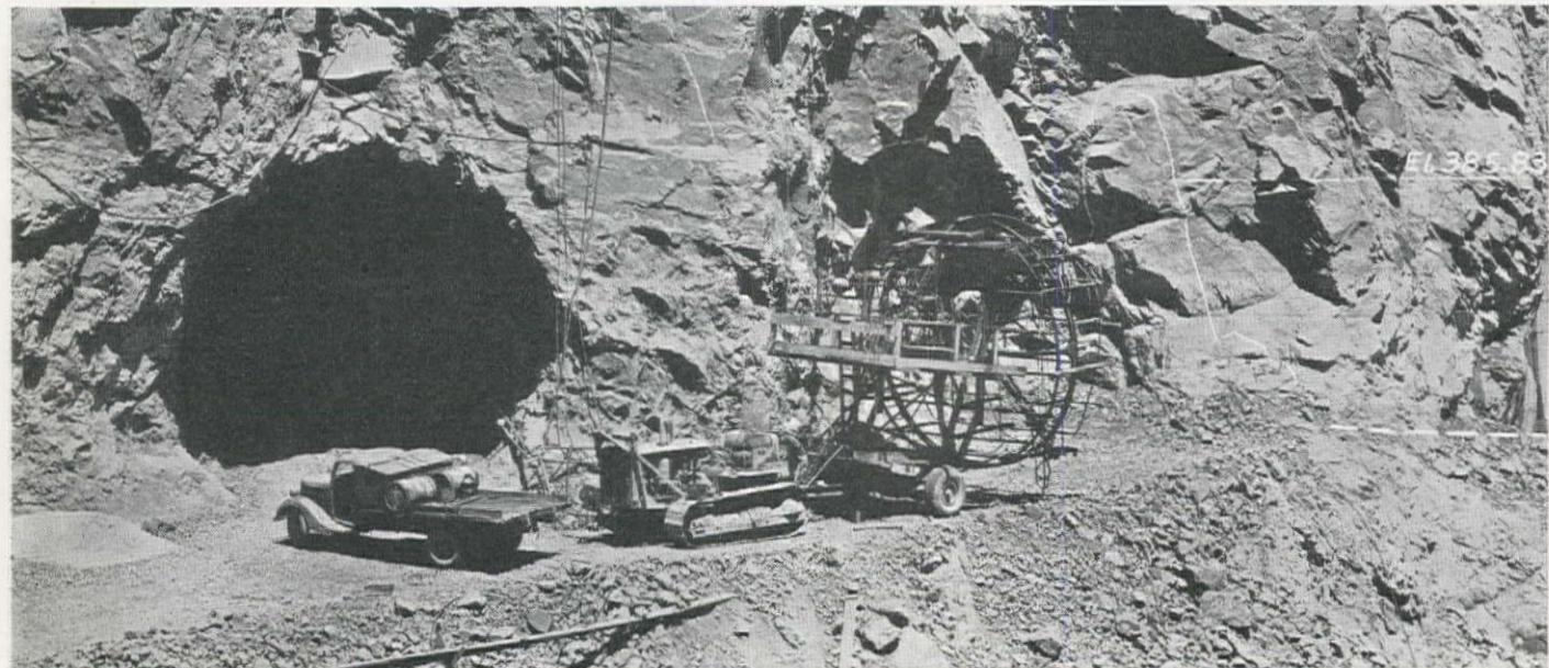
AS A PART of the contract for completing the power plant excavation at Parker Dam on the Colorado River, Clyde W. Wood, Los Angeles contractor was required to drive four 27-ft. penstock tunnels of varying length on grades which varied from 20 to
