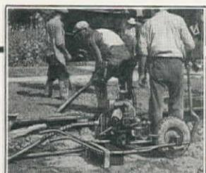
Equipped as a Concrete Vibrator
