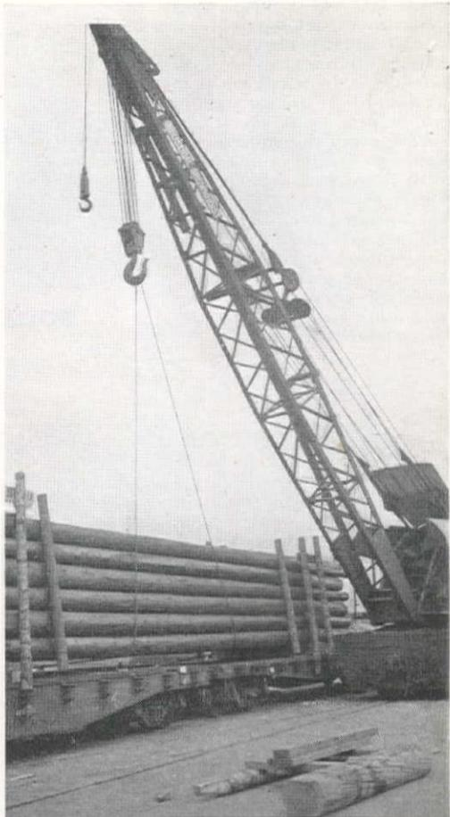
A CABLE is placed under the piling with the loop over the railroad crane hook and the free ends fastened to the metal pockets on the side of the car nearest the water. All tie wires on that side are cut and the upright timbers on that side are partially cut away, permitting them to break as the crane lifts the cable and the piles.
