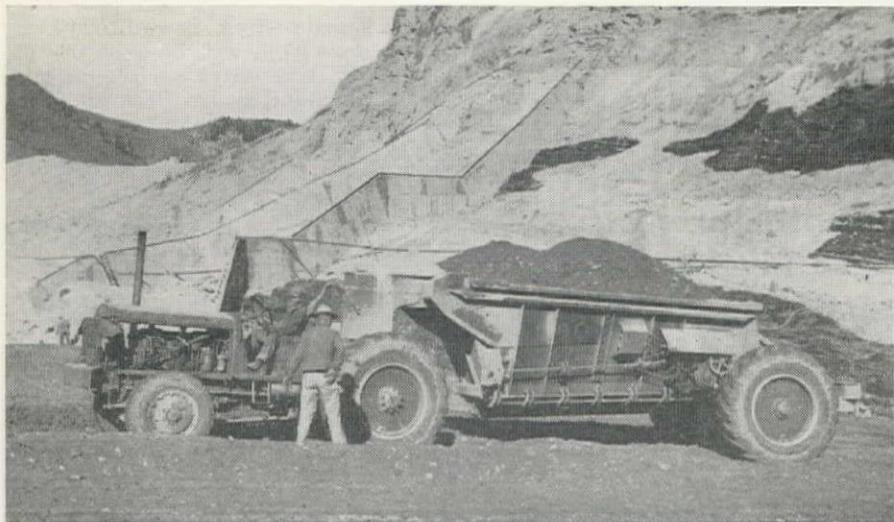
**FINE MATERIAL** (minus 3-in.) is hauled from the screening plant to the embankment in Euclid tractor and semi-trailer. The favorable type of material available and careful control will probably establish compaction records at Green Mountain.
