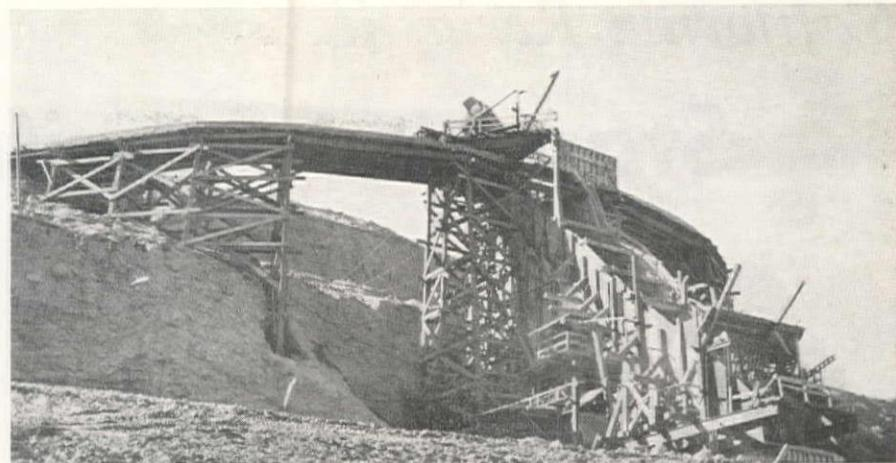
REMOVAL of plus 3-in. material from the spillway and borrow pit excavation is accomplished by a large screening plant erected on the bank. The high approach ramp eliminates steep construction roads and permits gravity flow of materials through the plant.
