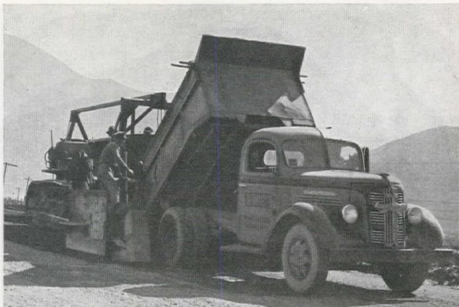
**SPREADER BOX** for placing the cement stabilized base consisted of a bulldozer mounted on a tractor with side walls added to the dozer blade. Wheels and screw jacks provided the depth setting facilities.
