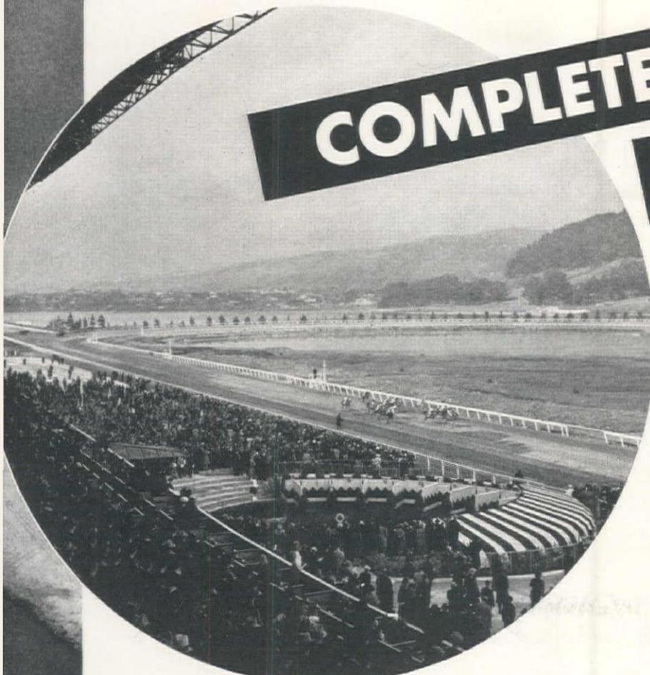
At the halfway stage the site of the track looked like a busy ant hill from the air. The grandstand rests in the center cut and the fill at the right was completed to form the car-parking area.
