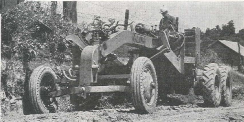
Here we show how all of the hard work is taken out of Galion motor grader operation. At the touch of a lever (see photo left) all adjustments are made instantly and quickly. Note also the wheel which controls the hydraulic steering mechanism, giving the operator a break on tough maintenance. Note, too, the 3-passenger seat. Investigate this salient feature on Galion 101 - 201 motor graders.
