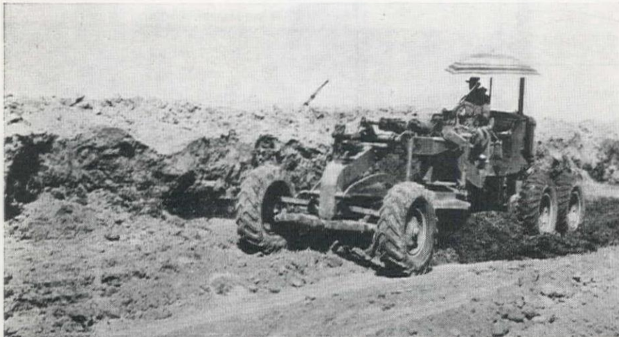
LARGE TIRES float blade on wet muck.
