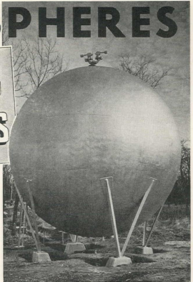
BELOW, LEFT: 36 ft. diameter Hortonsphere installed at a sewage disposal plant in Sioux Falls, S. D.
