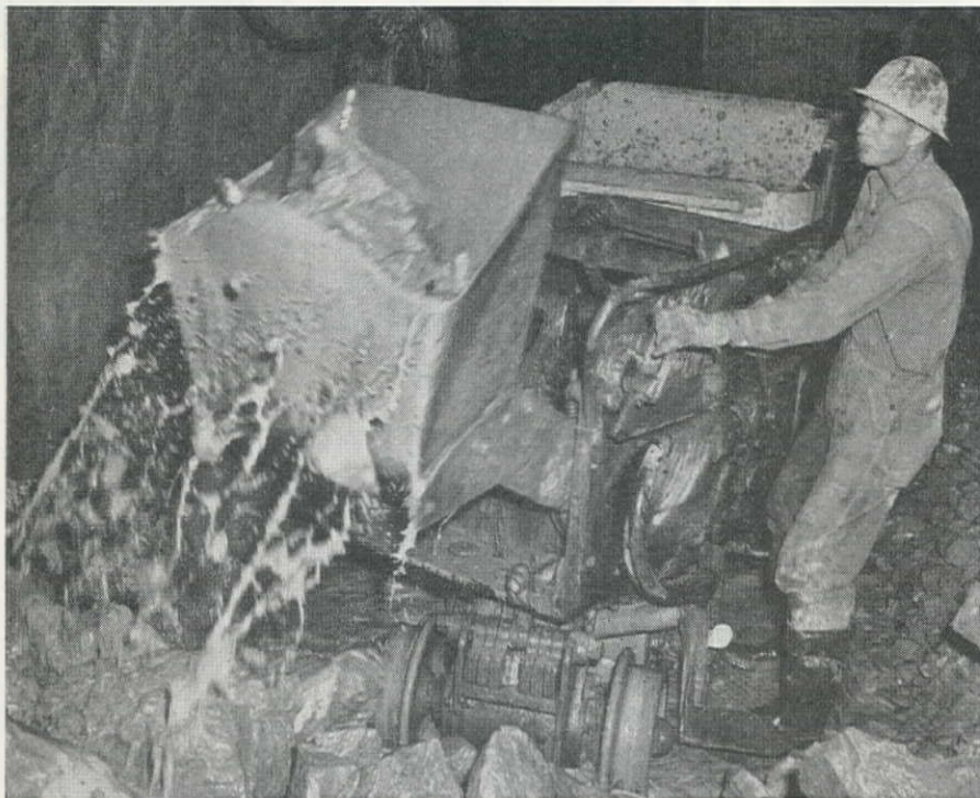
MUCKING out a 7-ft. round which averages 30-cu. yd. in a loading time of about 1 hr. 30 min. Rounds are loaded with about 250 lb. of 40% or 45% explosive (60% in the lifters).
