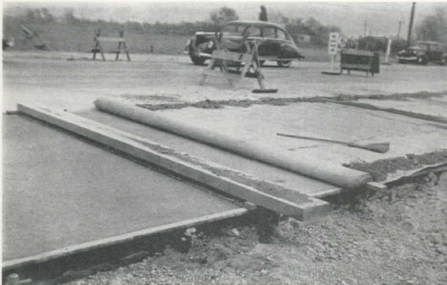
CURING of the test sections was carried out under a waterproof membrane, as indicated, which was placed on the pavement and held down by small ridges of dirt.
