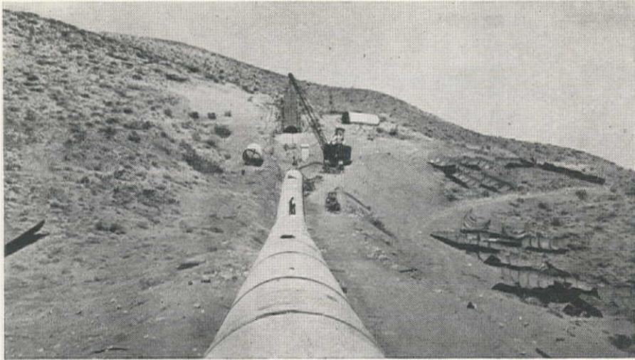
PLACING new pipe on Big Jawbone siphon. Work was started simultaneously at both ends and the water level kept as nearly as possible up to the work to maintain an even temperature.
