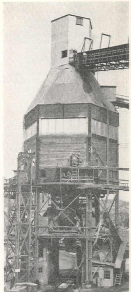
MIXING plant is located at the south abutment with facilities for direct discharge into buckets on concrete trains.
