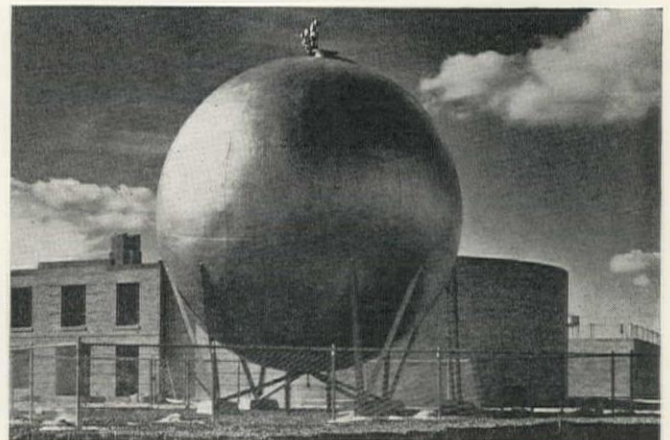
BELOW, RIGHT: 28 ft. 8 in. diameter Hortonsphere used to store 25,000 cu. ft. of sewage gas at a large New England sewage disposal plant.
