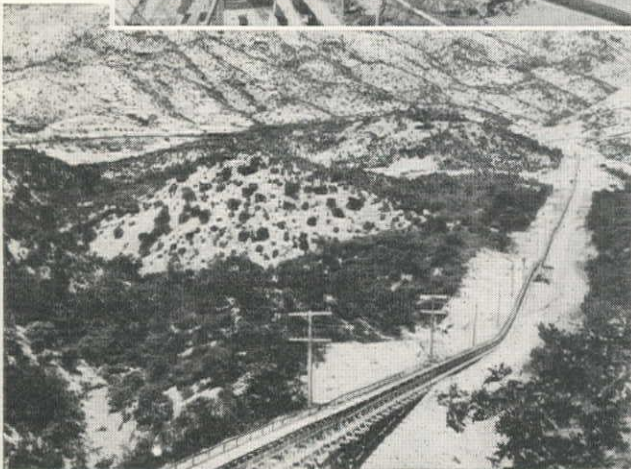
The start of the 9.6-mile conveyor system. Aggregate is carried from Redding, Cal., to the dam site over rivers, highways, and mountains.
