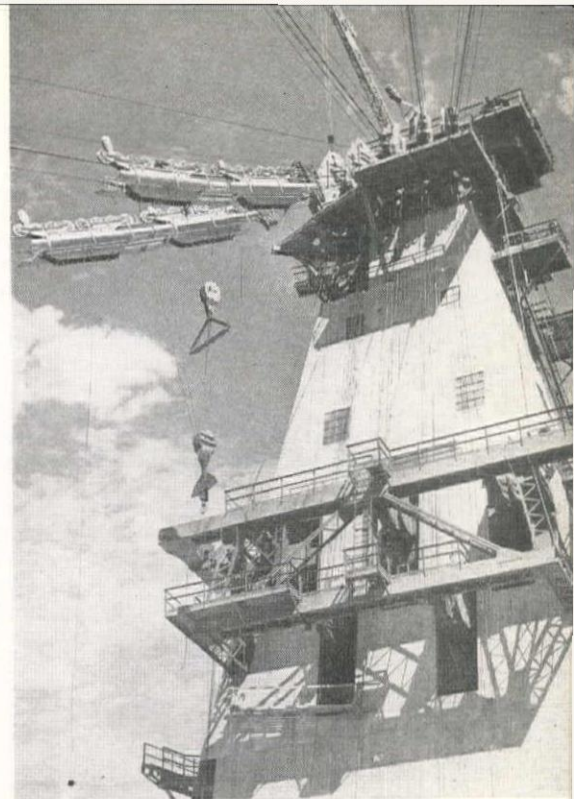
CONVERGING on the head tower, the seven cableways are arranged to cover the dam and powerhouse area. Weight of concrete, bucket, and rope and carriage total about 33 tons, handled with a 6% sag in the main track cable.
