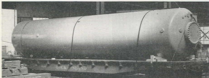
RIGHT: 20 ft. diam. by 85 ft. elevated ore bin of welded steel construction.
