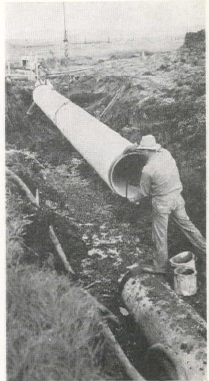
PREPARING the spigot end by placing the rubber seal in groove. Bell and spigot are special steel ring sections welded to the shell.
