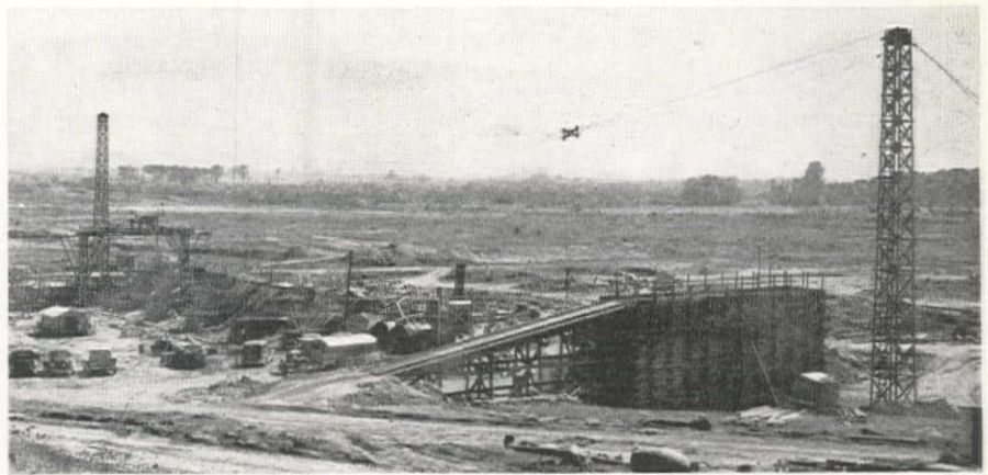
SPILLWAY CONSTRUCTION at Fern Ridge Dam indicating the contractor's method of concrete distribution from the batching plant in the foreground. Spillway discharge will be controlled by six automatic hydraulically-operated radial gates.
