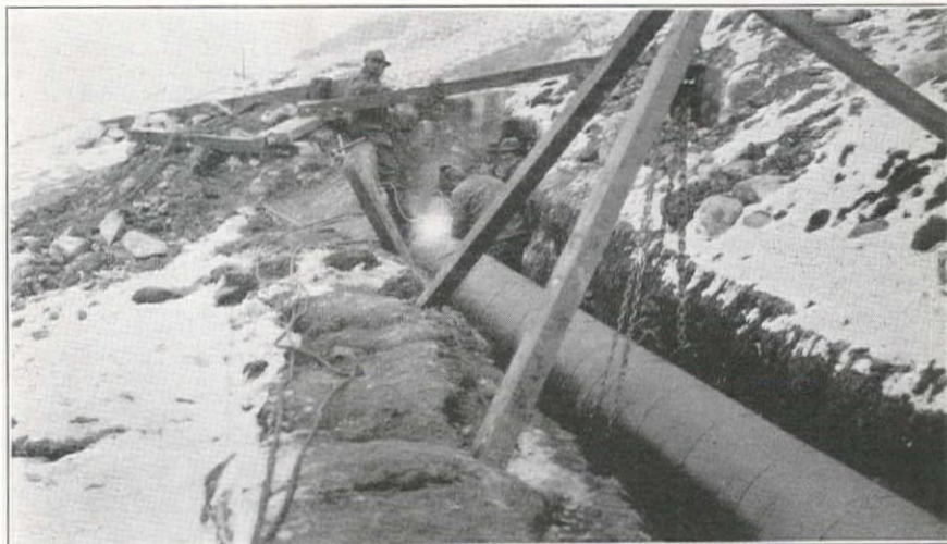
Logan, Utah, installed 2885 feet of 20-inch, and 400 feet of 16-inch Calco Spiral Welded Pipe, with field welded joints near mouth of Logan Canyon.
