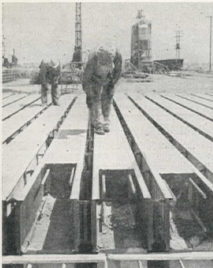
AFTER FORMS have been stripped from the highest tier the sections are separated and loaded onto a flat-bed truck for hauling to a new casting location. Piles are kept moist during the curing period by an occasional spraying.
