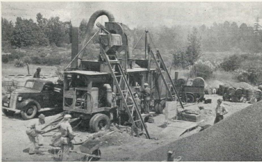
PORTABLE hot mix plants are used by Oregon maintenance forces in surface repair work. These plants, of which there are eight, consist of two drum heaters with a pug-mill type of mixer placed between them. They have a capacity of about 175 tons per 8 hr., running batches of 1,000 lb.
