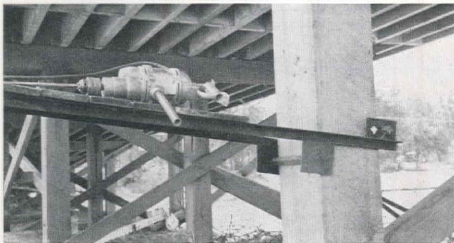
THE SCAFFOLDING , shown here in place on a 12-in. timber column, functions on the old lever principle with the lower cross bar acting as the fulcrum. To raise or lower the scaffold it is only necessary to lift the far end (at the left) and slide the scaffold up or down the column.
