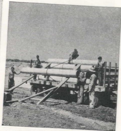
HONOLULU, T. H. Long, light, 13-foot lengths of Transite Pipe reduce handling costs. Smaller trucks carry large loads to location. No mechanical equipment is needed for loading and unloading.
