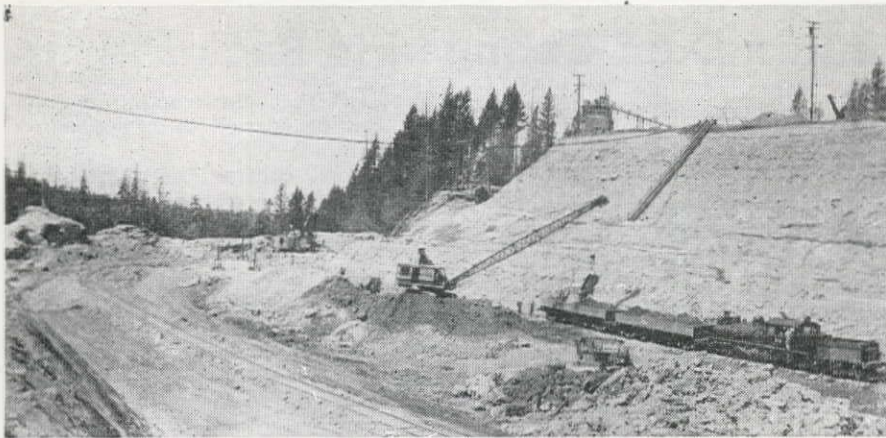
IN THE SPILLWAY where more than 1,150,000 cu. yd. were excavated by shovel and dragline and hauled by railroad train to disposal areas. Spillway capacity is 139,000 sec. ft.; the maximum flood of record (1933) is 28,000 sec. ft.
