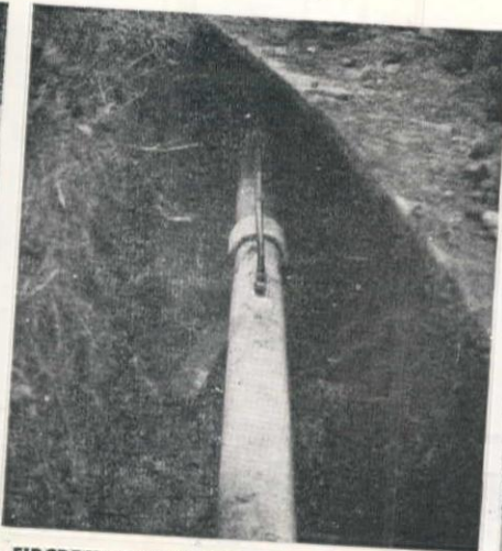
FIRCREST, WASH. Fittings and service connections may be cut into J-M Transite Pipe quickly and easily, for this modern material can be readily cut, sawed or drilled with ordinary tools.
