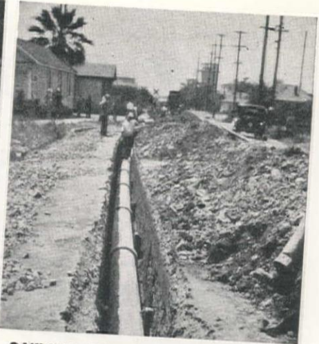
OAKLAND, CALIF. J-M Transite Pipe is non-metallic and inorganic... cannot tuberculate under any conditions. As a result, carrying capacity (C-140) stays high, pumping costs low.
