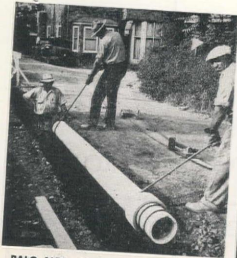
PALO ALTO, CALIF. On the job, crews can lay J-M Transite Pipe as fast as the trench is opened. Transite's long lengths and simple, rapid assembly method assure unusually low installation costs.
