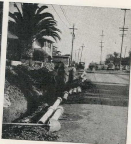
MARTINEZ, CALIF. Simplex Couplings are quickly assembled, even by unskilled crews. They provide unusually tight, flexible joints that stay tight in service . . . keep leakage at the minimum.
