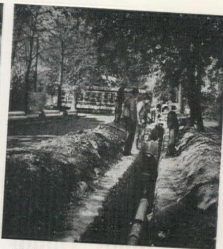
YONKERS, N. Y. No large bell holes are needed at joints when J-M Transite Pipe is installed. This means that trenches can be narrower and more economical and that damage to pavements is minimized.
