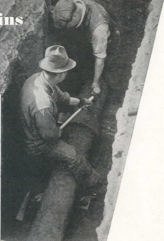
When New York City engineers uncovered this 105-year-old cast iron water main to cut in a new valve, their comment was "that pipe looks good enough to last another hundred years."
