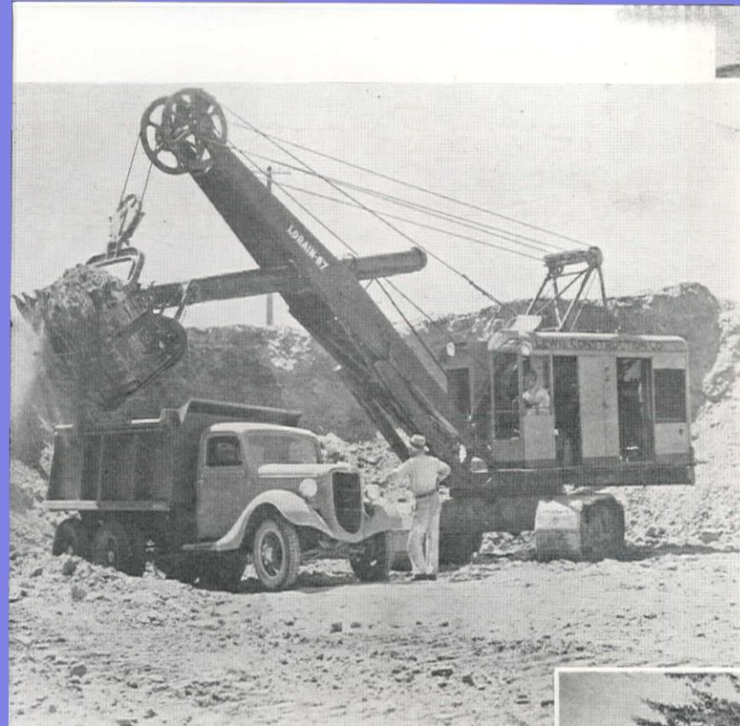
All-American Canal work ( above ) continues with the project more than 50% complete. At Potholes, Calif., on the contract of the Lewis Construction Co., this 2-yd. Lorain-87 is moving material on a 900,000 cu. yd. section of the work.
