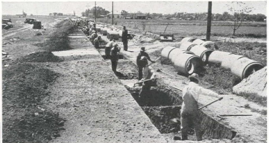
Trench digging (above) by WPA labor to install a 30-in. combination sanitary and storm sewer to connect with the outfall sewer of the city. This new connecting line is about 1 mi. long. General grading operations (left) on the site of the old amusement park after the buildings had been removed. The oval marks the location of the midget auto track.
