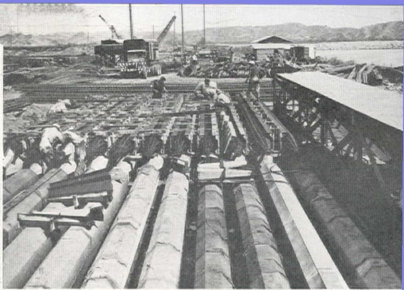
Casting of concrete piles ( above ) is one of the first steps in the construction of the Imperial Dam, the diversion structure for both the All-American Canal and the canal for the Gila project from the Colorado River. This pile casting work is part of the contract of Morrison-Knudsen Co., Inc., Utah Construction, and Winston Bros.
