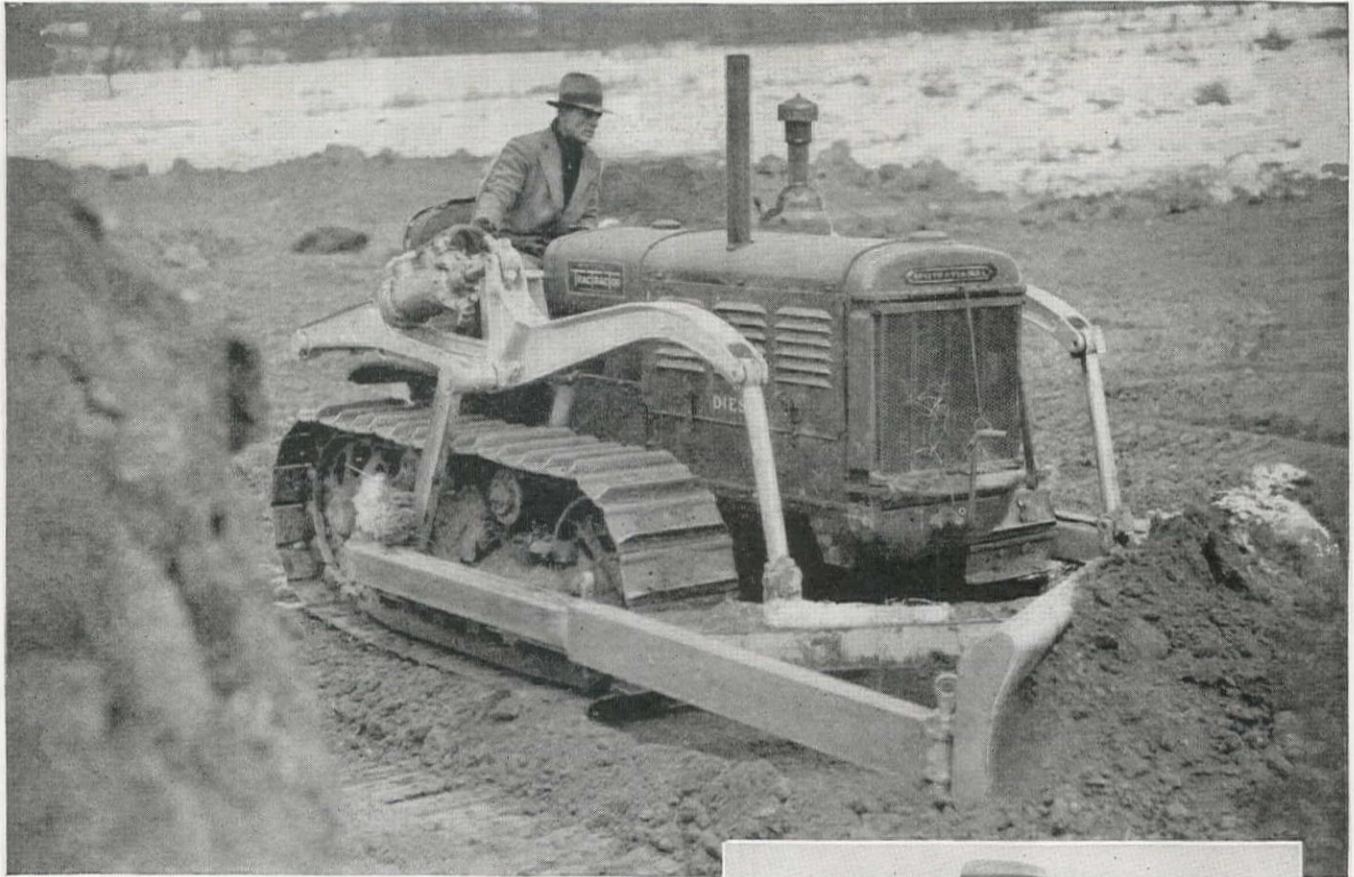
The manufacturer of this side-mounted bulldozer specializes in equipment for a special job. International supplies the power that makes it work—a Diesel TracTracTor.
