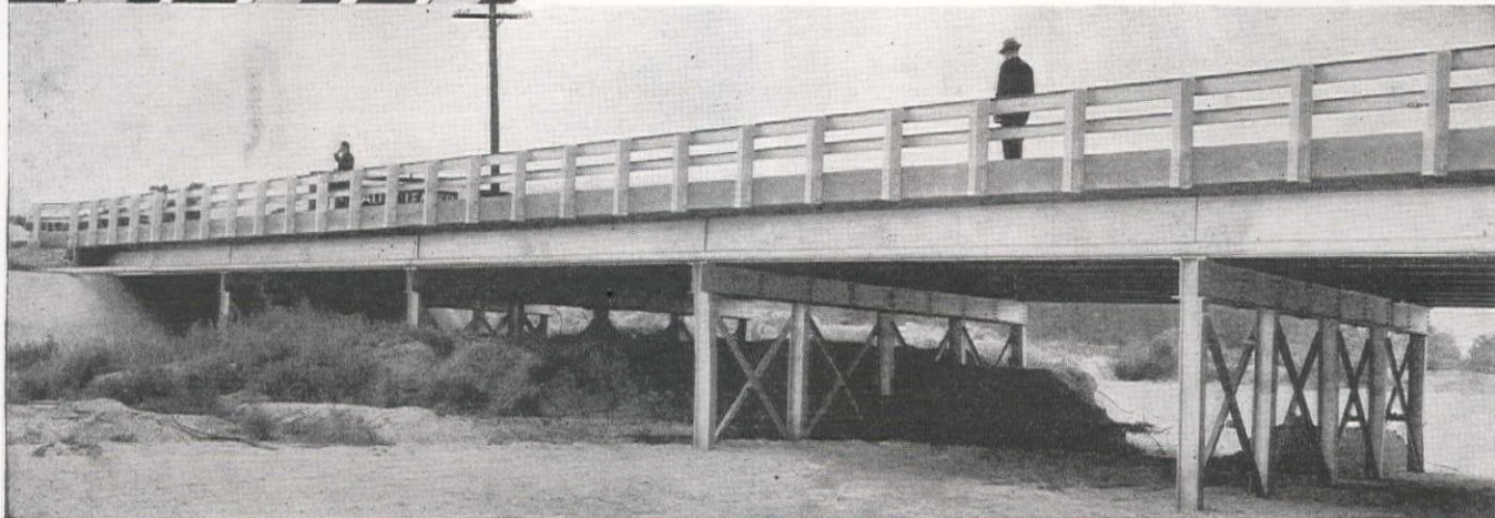
This bridge, at San Bernardino, Calif., is built on Bethlehem Steel H-Piles. Note the alignment and sturdy appearance of the steel H-piling bent. The steel girders of the bridge rest on a cap consisting of two structural-steel channels, riveted to the H-piling.
