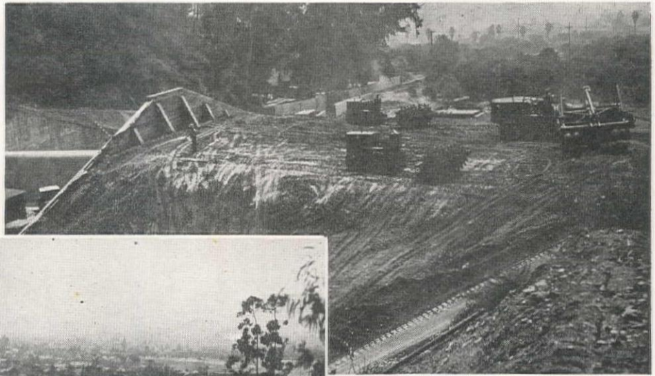
Compacting the earthfill for the west abutment of the dam for Brand Canyon basin. The spillway crest appears at the left. Construction of the spillway channel appears in the background.
