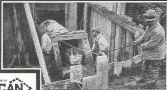
Jacking Toncan Pipe Under Railway Tracks at Geneva, N. Y.
