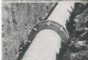
Illustrated, a 7,000-foot installation of 8-inch, 10-gauge Calco Spiral Welded Pipe, recently placed by Downey, Idaho.
