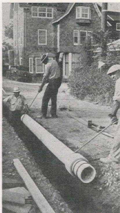
Placed in proper position on the pipe, the rubber rings and the collar are pulled into place by a jack. The rings flatten as they roll under the collar.
