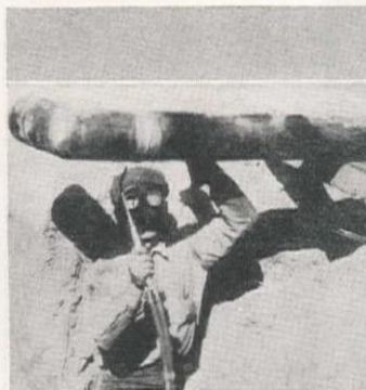
Field joints may be welded as shown above, or made with standard couplings as shown below.
