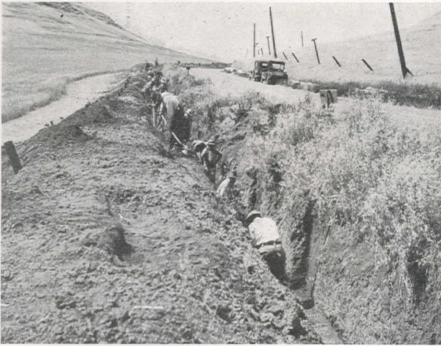
A crew of about 60 WPA laborers excavated the entire 3-mi. line by hand. The crew is shown clearing out the trench, excavated several weeks before, after they had been taken off for emergency flood work.
