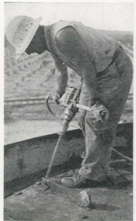
Finishing the surfaces of a pipe, using an air rotated steel rod, moved along the sides of the forms. This procedure, immediately following casting, eliminates air and water pockets and reduces surface defects. The operator is standing on the top of the inside form.
