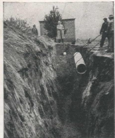
INSTALLATION SAVINGS. A 16" line—an unusually deep trench; but lightweight Transite was laid down quickly, economically, without mechanical equipment. (W. Warwick, R. I.)
