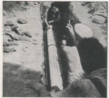
ENDING TUBERCULATION. In relatively few years tuberculation had seriously reduced the capacity of water lines at Belmont, Mass. Hence, for their recent Cushing Ave., project, they specified Transite, the non-tuberculating pipe.
