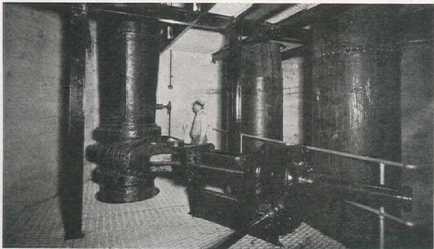
Forty feet below the operating level are the valves (below.) The opening and closing mechanism of the horizontal unit is operated by worm gear driven through a shaft from the water motor above. These riser pipes are in the lower section of the caisson.
