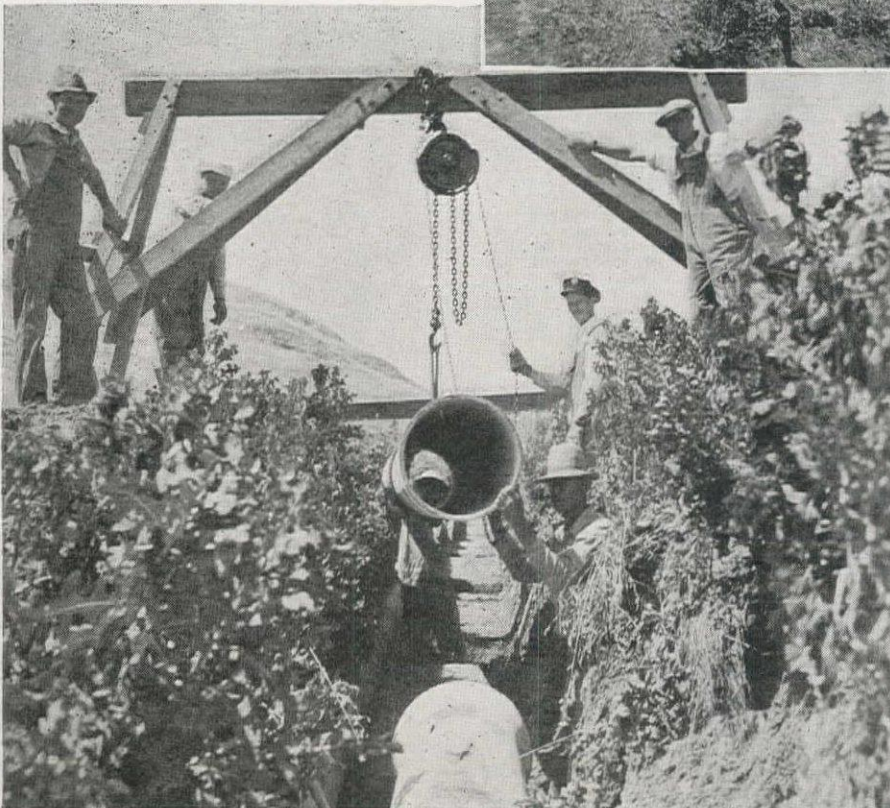
Using only hand equipment, this WPA crew of six rolls the 2,600-lb. lengths of pipe across the road and lowers them into the trench with a chain-block in a time of about 20 min. per length. Note the weed-grown condition of the trench which was originally dug several weeks before by hand labor.
