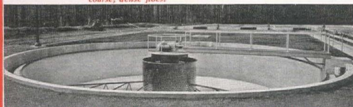
Then, a Dorr Clarifier for the removal of suspended solids.
