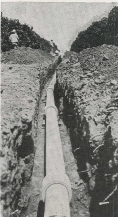
One of the first lines of cement-asbestos pipe to be placed in service in the West.
