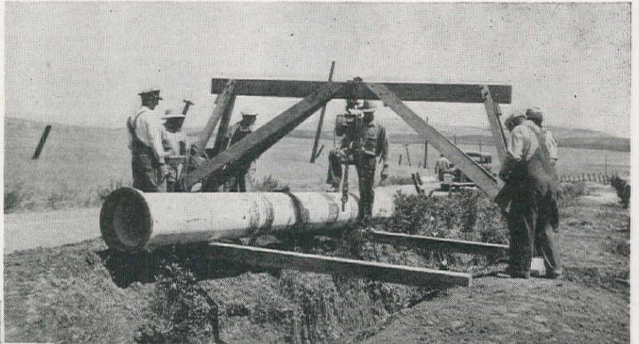
Using only hand equipment, this WPA crew of six rolls the 2,600-lb. lengths of pipe across the road and lowers them into the trench with a chain-block in a time of about 20 min. per length. Note the weed-grown condition of the trench which was originally dug several weeks before by hand labor.
