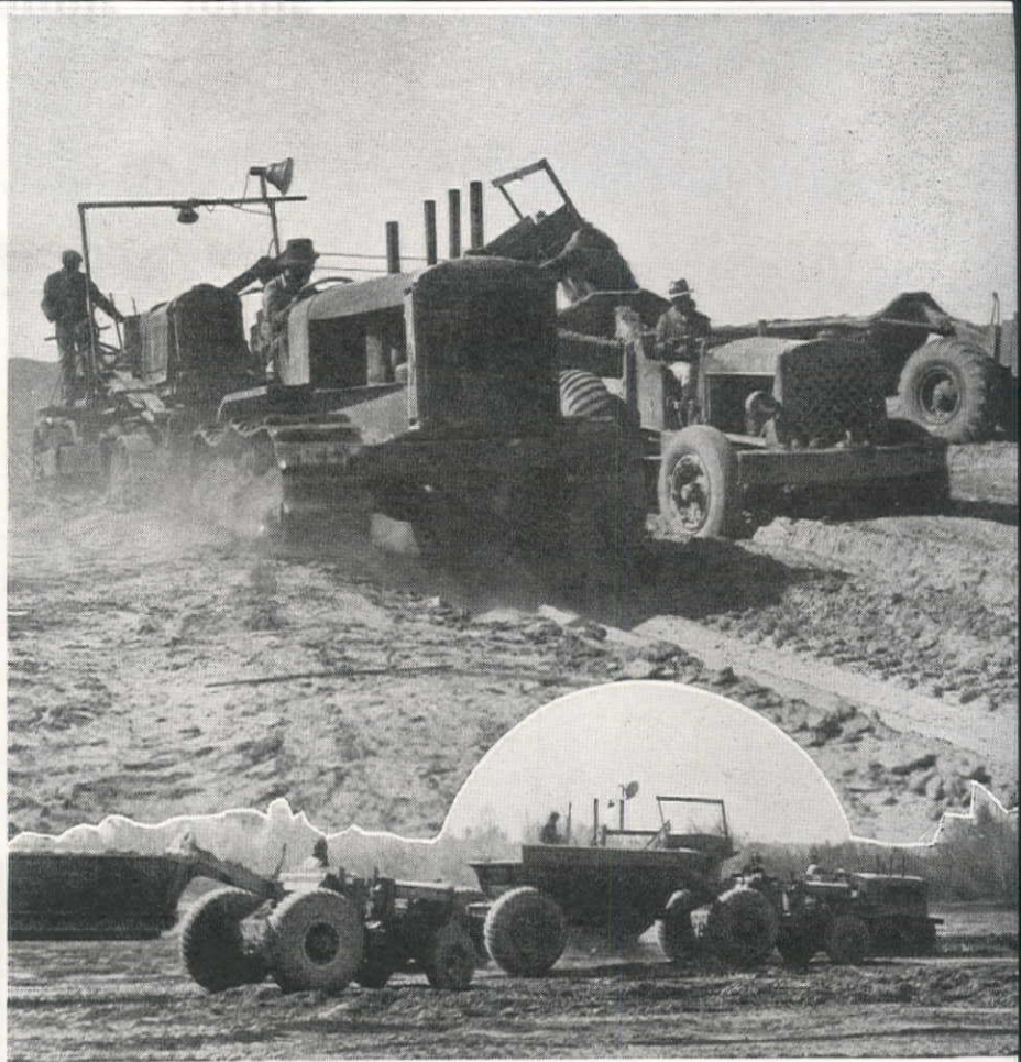
On the extensive flood control work being carried out by the U. S. Engineers on the Los Angeles County Flood Control project, this Bucyrus-Erie (CT-50) loadmaster (left) handles brick from stockpile to bottom of trench. The work involves 5½ mi. of 12-ft. diameter storm drain in Kenter Canyon near Santa Monica.
