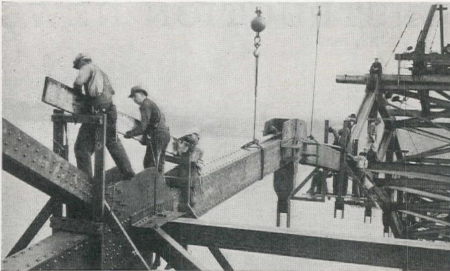
Final connection of the lower chord member of the main arch. Details of the box type chord members are shown. This closure was effected by lowering the two halves of the arch by means of the cable tie-backs.
