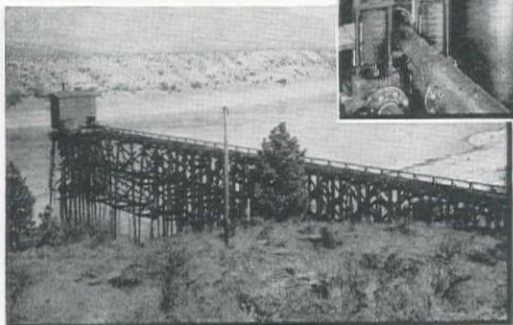
Two of three Worthington Deep Well Turbine Pumps ... each pumping 2500 g.p.m. against a total head of 670'
