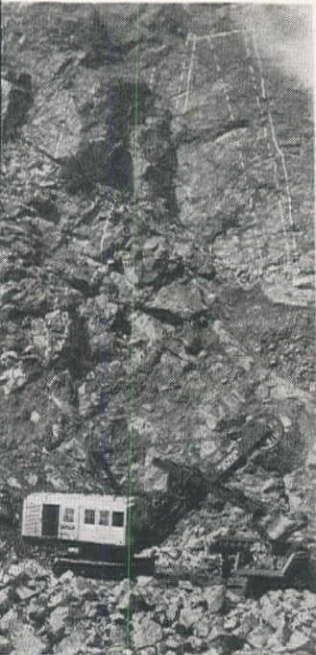
Heavy excavation (above) starts at the site of the Seminole dam in Wyoming with a 4-yd. Bucyrus-Erie electric shovel. The contract is held by Morrison-Utah-Winston-Lawlar Co. J. H. Warner is resident engineer for the Bureau of Reclamation.
