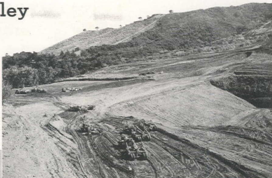
Typical dam site conditions (Stevens Creek dam) showing the earth-moving equipment bringing fill to be rolled in 6-in. layers.
