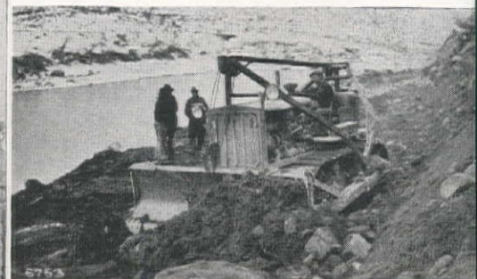
Quinn Robbins Co., on an Idaho highway job near Emmett, is using one of the new model LeTourneau Angledozer for moving sidehill cut as shown below. This mounting places all stress on the track frame of the tractor, rather than on the motor frame.
