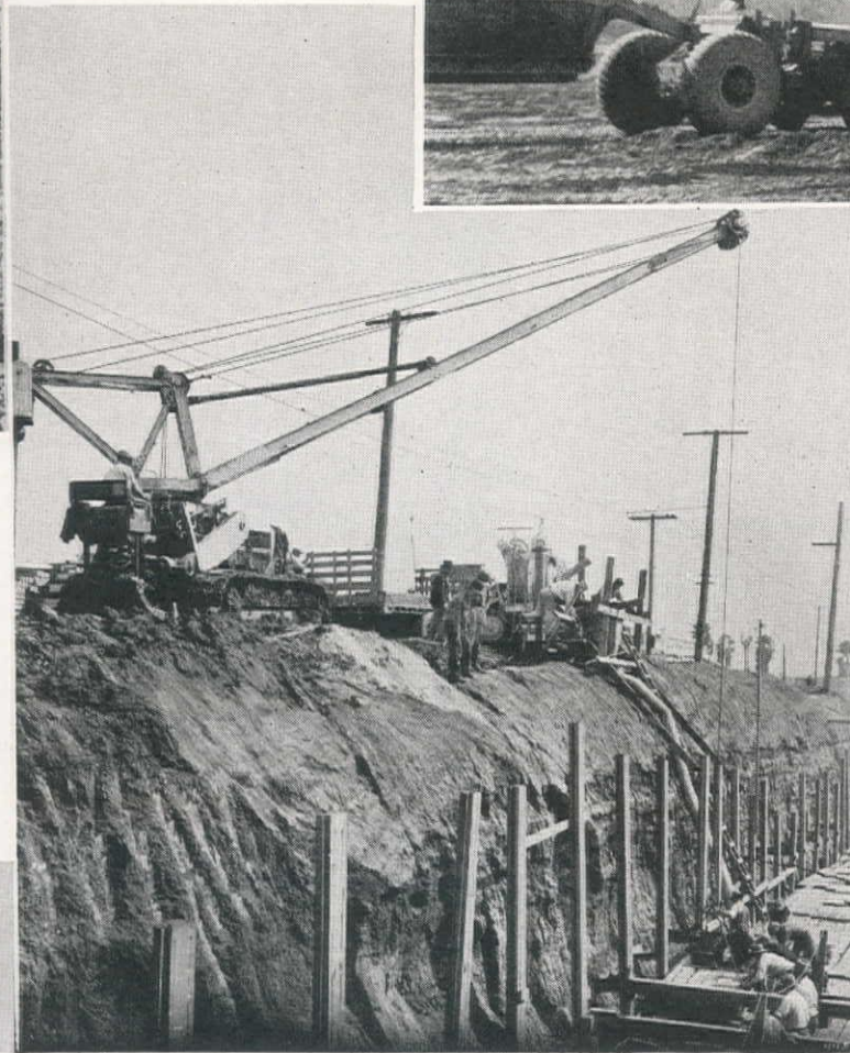
Heavy excavation (above) starts at the site of the Seminole dam in Wyoming with a 4-yd. Bucyrus-Erie electric shovel. The contract is held by Morrison-Utah-Winston-Lawlar Co. J. H. Warner is resident engineer for the Bureau of Reclamation.
