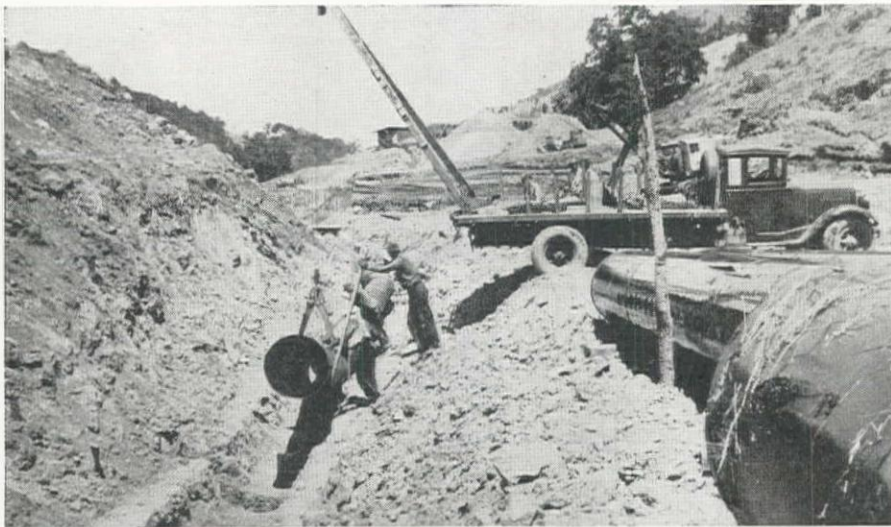
Outlet works consisted of steel pipes, jacketed with poured concrete, placed in trenches excavated into the foundation material.
