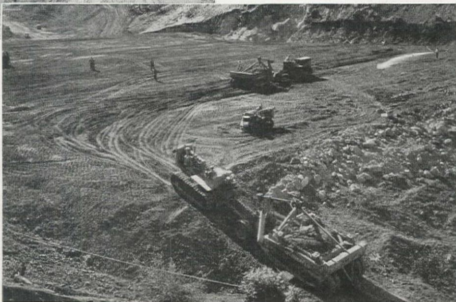
Typical earth-moving methods (Almaden dam) showing the Caterpillar tractors and LeTourneau Carryall scrapers used to handle most of the fill.
