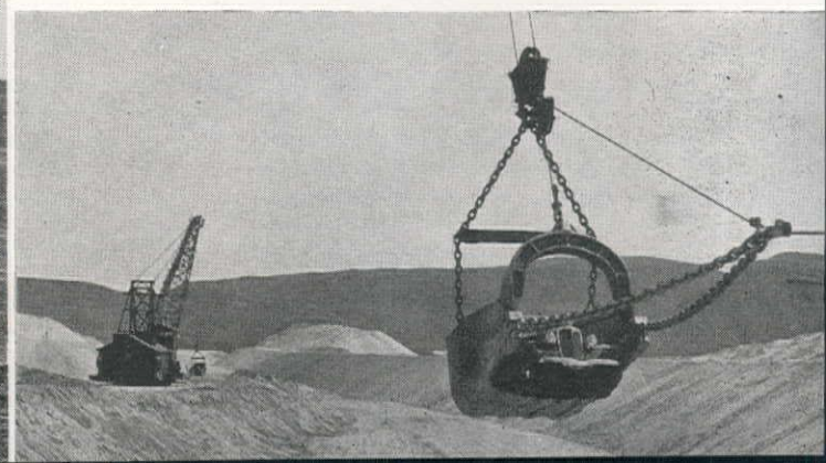
The 12-yd. dragline buckets (below) used in excavating the All-American Canal, handles the engineer's automobiles without any crowding.
