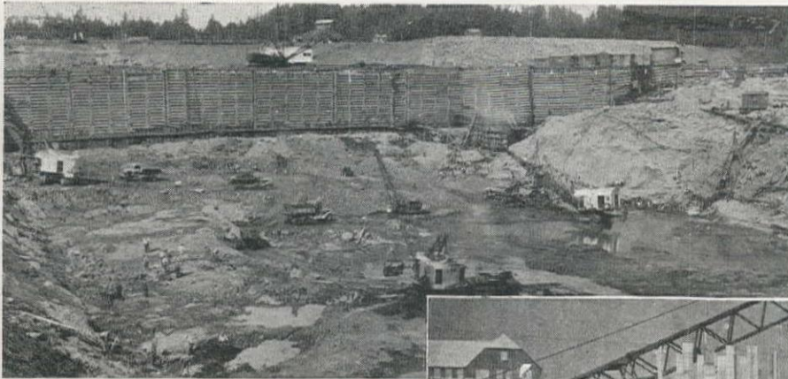
Inside the unwatered south cofferdam for the main spillway dam. An idea of the tremendous size of the cribs may be obtained from this view.
