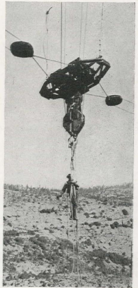
Main control block and fall block showing control lines to the up- and downstream control cables. The fall lines run through the control block, as shown, to the main cable carriage.
