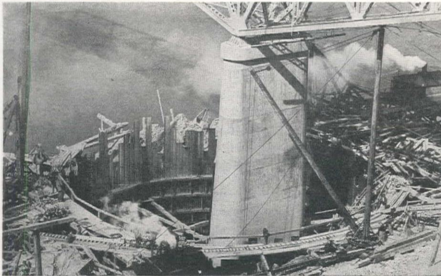
Steel sheet pile cofferdam and excavation operations used in bringing the east pier back to plumb.
