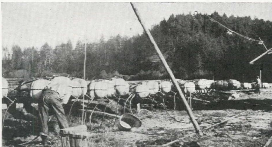
Fender piles were treated with a solution of mineral salts, forced into the butts of the piles with a 6-lb. pressure. Using the rubber pressure caps shown, six days are required for the solution to saturate the sap wood of a 75-ft. pile. Cost of treatment was 28¢ per lin. ft.
