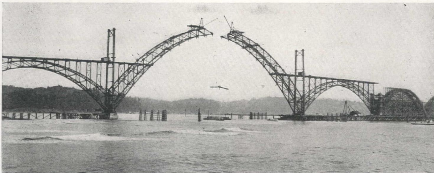
Closing member of the bottom chord of the main span going into position. This arch is 250 ft. high at the crown, and spans the navigation channel at the entrance to Yaquina Bay.
