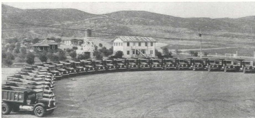
To haul the 7,000,000 cu. yd. of earthfill material, this fleet of 30 Mack trucks is used. They have been converted to burn butane gas, and consume 2,500 gal. per 24 hr.
