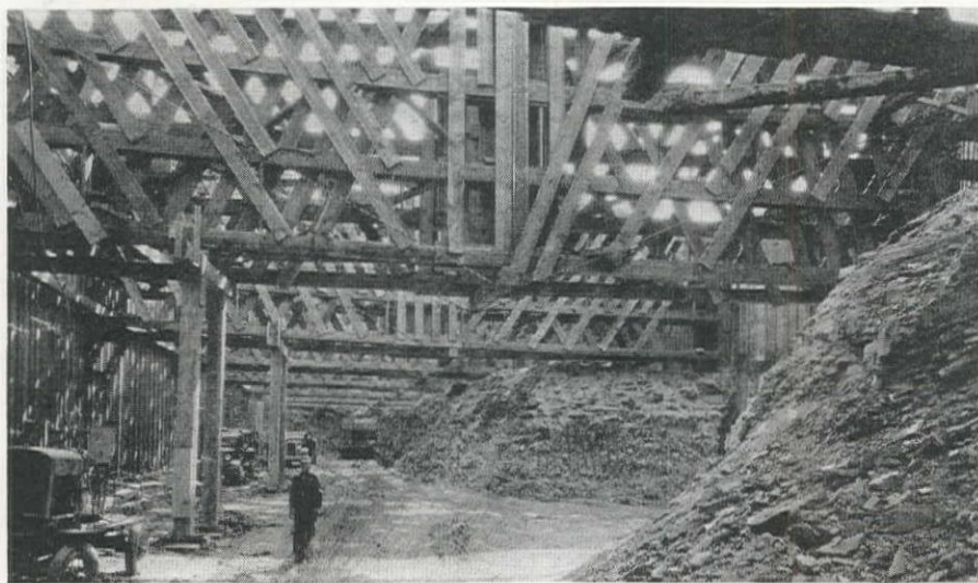
Extensive timber bracing was used to hold the area excavated for the placing of concrete in Block 40 immediately behind the cofferdam wall.
