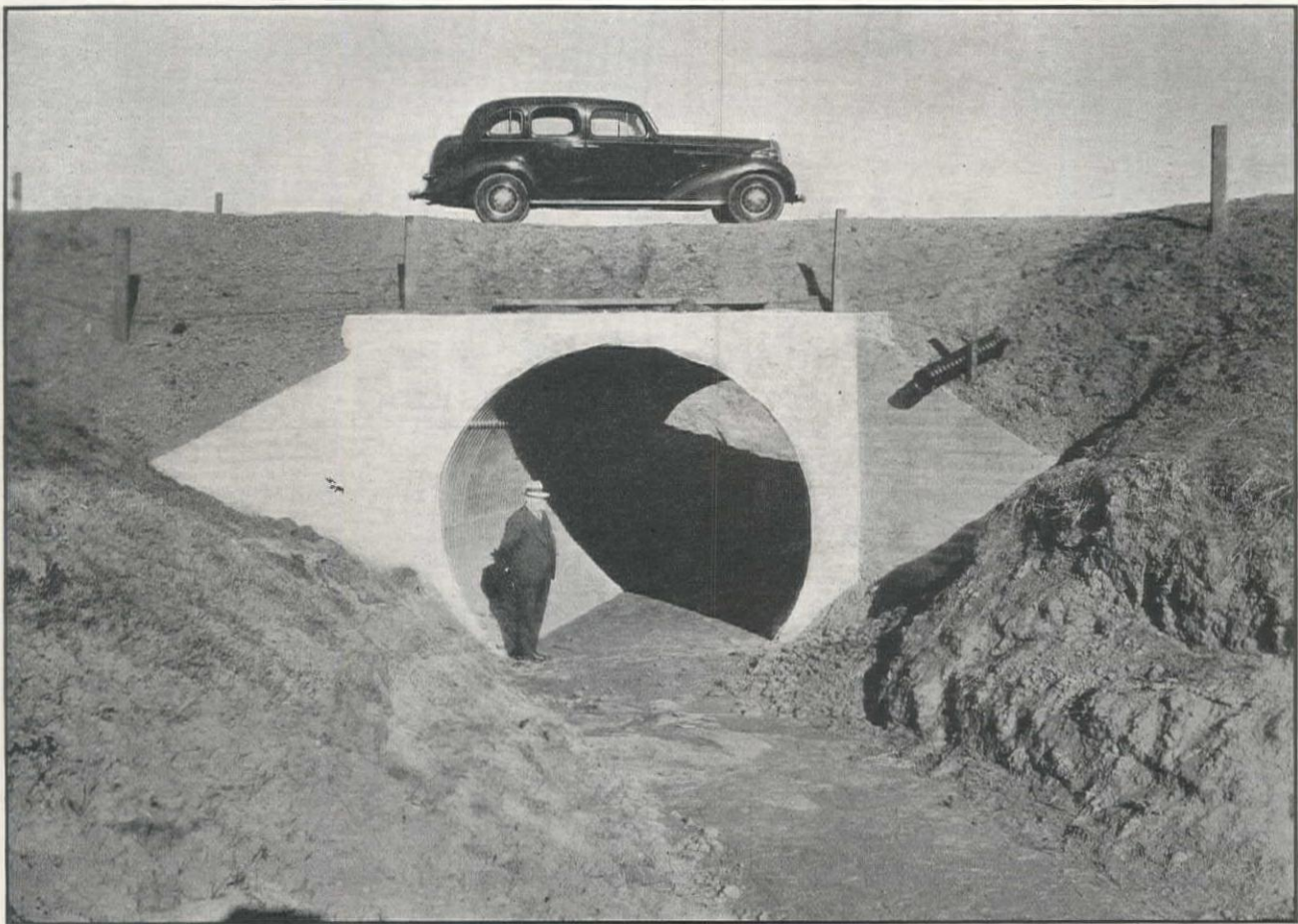
150" Multi Plate which replaced old bridge near Antioch, Contra Costa County, California.
