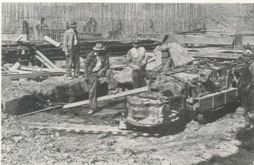
Fig. 6—Modified coal-cutting saw used in digging trenches for the cutoff collars and trimming the horizontal surfaces of the foundation shale for the gate structure. This type of saw, capable of cutting through an arc of 180° was advanced on rails after completing each arc. The loose material was removed by a pull shovel or by hand as the saw advanced.
