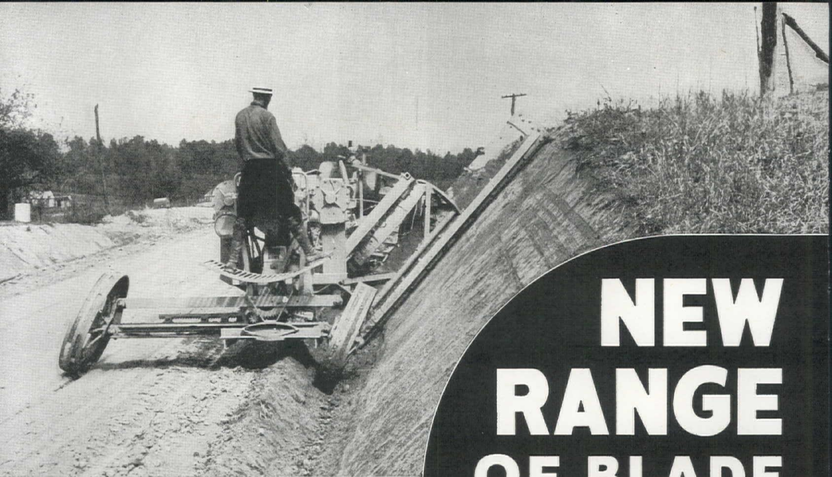
This 12-foot blade is cutting a 1 to 1 slope on a bank 8 feet high; it is capable of cutting much higher of course on steeper banks.
