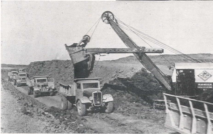
Fig. 4—Typical excavation and hauling operations on the entrance and lined section of the canal, which were remarkable for their efficiency and speed. Work was continuous on a 7-day per week basis and the organization of men and equipment was so well arranged that a record of 46,754 cu. yd. was moved in one day. High speed, 6-yd. trucks shown above, formed the bulk of the hauling equipment on this contract of Spillway Builders, Inc.
