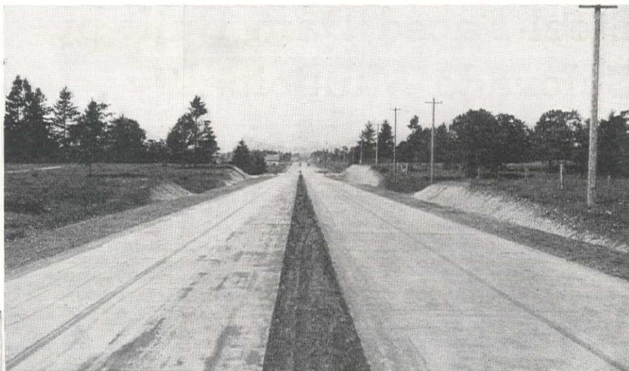
Double-strip design (above) which features the reconditioning of the Pacific Highway. Note the 4-ft. sodded neutral zone between opposing 20-ft. traffic lanes.
