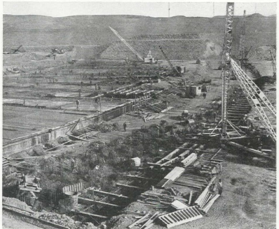
Fig. 9—General view of the excavation and foundation work on the gate structure. Foundation consisted of 467-5-ft. diameter concrete piles placed in bored holes, and a 10-ft. cutoff trench 30 ft. deep. The piles support a reinforced concrete foundation slab 75 ft. wide by 12 ft. thick on which rest the piers for the gates. Concrete placing is under way on the foundation slab in the background and the boring of the holes for the piles is under way at the left.
