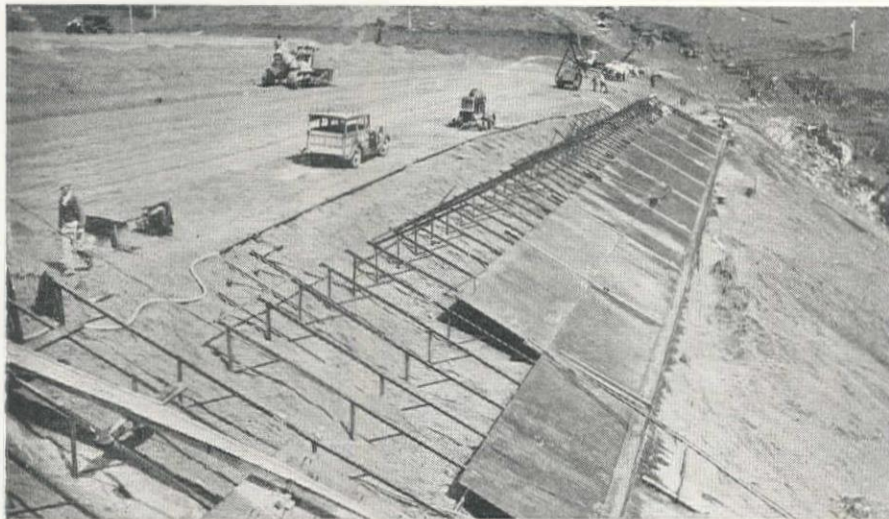
Beginning of the steel face above the concrete slab, which extends from cutoff to the elevation of the outlet pipe. Note the size of the steel plates and the supporting system of steel angles.
