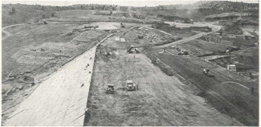
Carrying forward the fill and facing operations at the same time. Decomposed granite was used for the fill, sprinkled and rolled in 8-in. layers. Welders are shown at work on the steel face plates.
