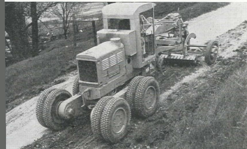
An impressive demonstration of power—scarifying a hard gravel road while traveling up a steep grade.
