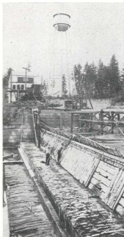
Condition of old timber dam at the time the new work was started. Trestle on the right was built by the contractor to support equipment.
