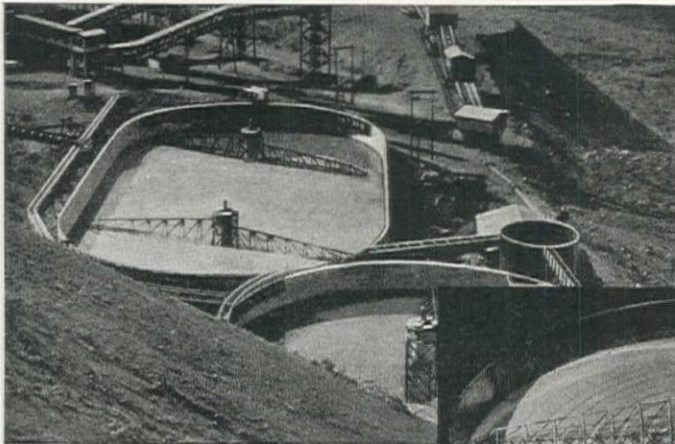
Three Dorr Torq Clarifiers at Grand Coulee Dam
