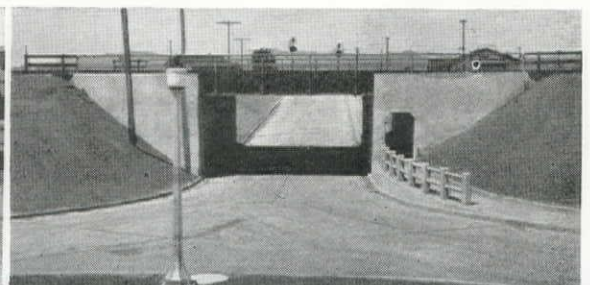
New Mexico is improving its highway system (below) by the construction of grade separation structure, such as this modern underpass at Lordsburg.
