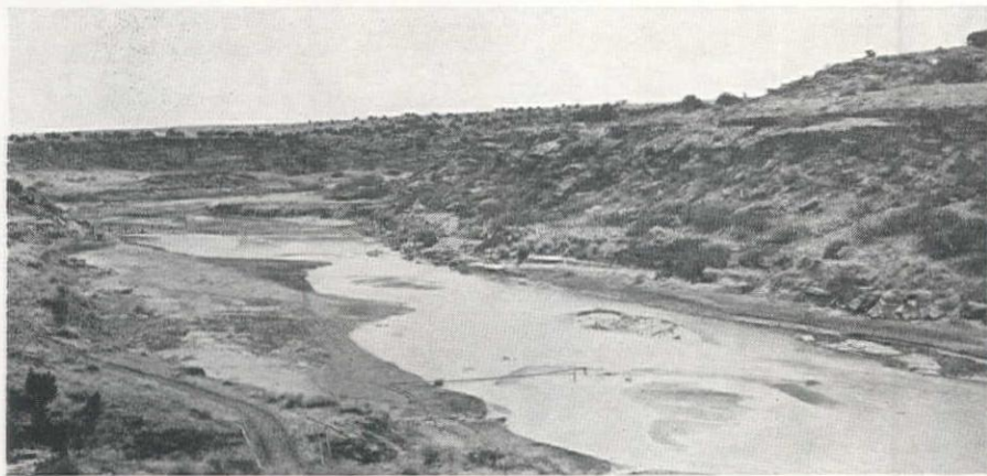
Conehas Dam site on the South Canadian River looking upstream. A dam 230 ft. high at this location will store 800,000 ac. ft. for flood control, irrigation, and municipal use.
