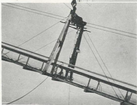
Completed catwalk (left) showing one of the gallowframes which support the hauling ropes at 230-ft. intervals. These frames rest on the four 2 1/4-in. cables and are held by guy wires as shown.
