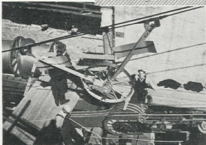
Arriving at the anchorage (left), the loops of wire are taken off the spinning wheel and placed around the strand shoe, and others placed on the wheel for the return trip.
