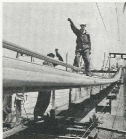
Each series of strands (right) is spun above the cable to permit adjusting, before lowering into position.
