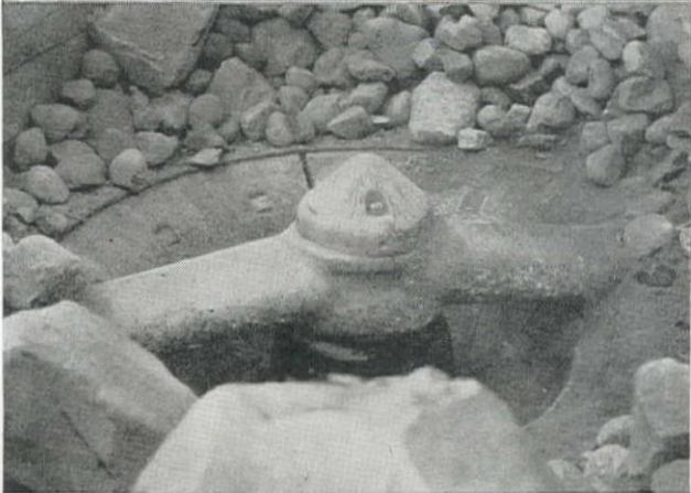
A No. 20 TELSMITH PRIMARY BREAKER CRUSHES ALL THE ROCK FOR THIS BIG PROJECT
