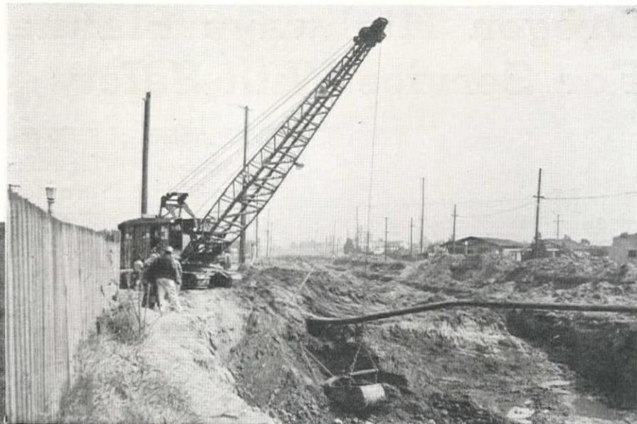
Present excavation work (above) on one of the flood channel units with 2-yd. P. & H. dragline.
