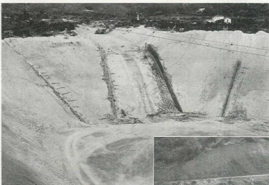
Inlet structure of a debris basin previously completed by the flood control district, which illustrates the type of approach work and detention space to be used in the new units.
