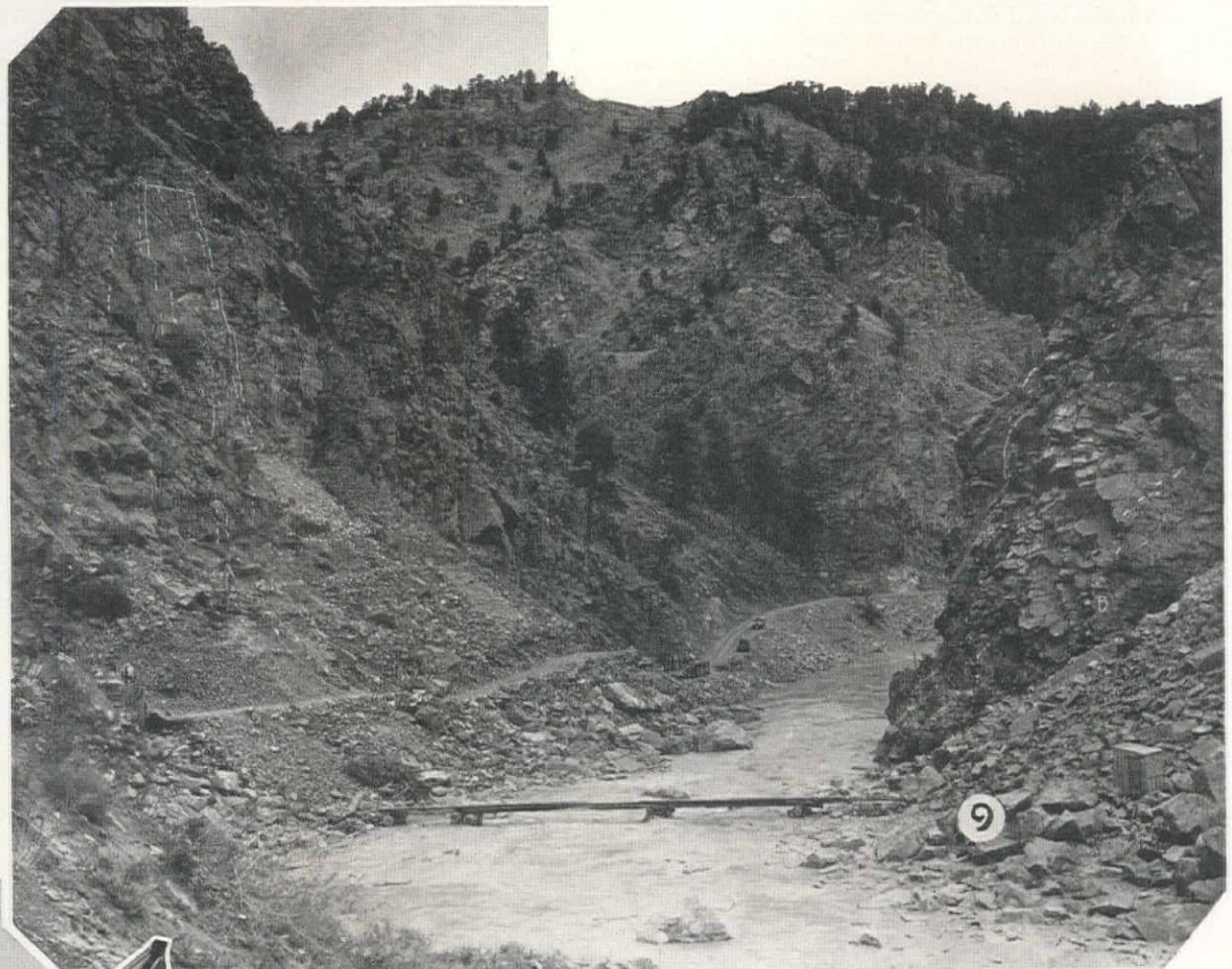
9—Seminoe dam site on the North Platte River in Wyoming, where a 260-ft. concrete dam will be built by the Bureau of Reclamation as the major structure on the Casper-Alcova project. White lines on the left abutment indicate the line of the dam.
