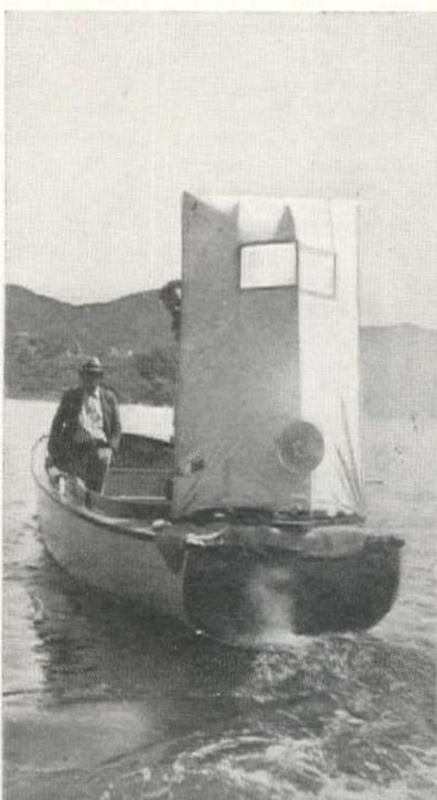
Appearance of the broadcaster (above) which scatters crystals uniformly over a width of 50 to 100 ft.
