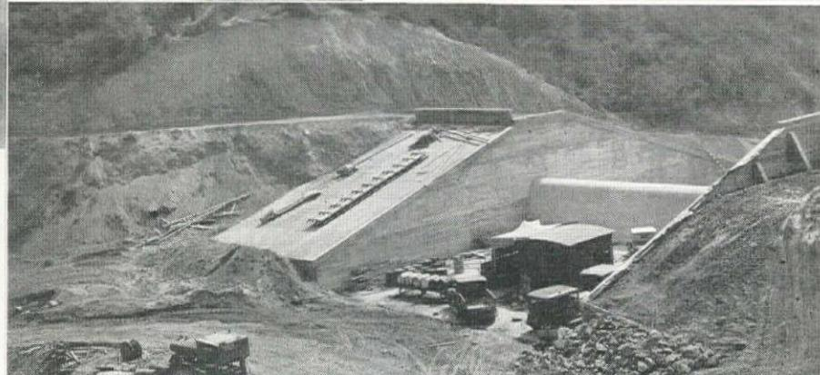
Outlet structure of previously completed unit, indicating the type of work to be done for the additional basins.
