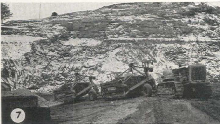
7—Early snows hit the job of the Utah Construction Co. on the Red Lodge dam project in Montana. The Caterpillar drawn LeTourneau scrapers are hauling as far as 1,600 ft. from the north borrow pit.
