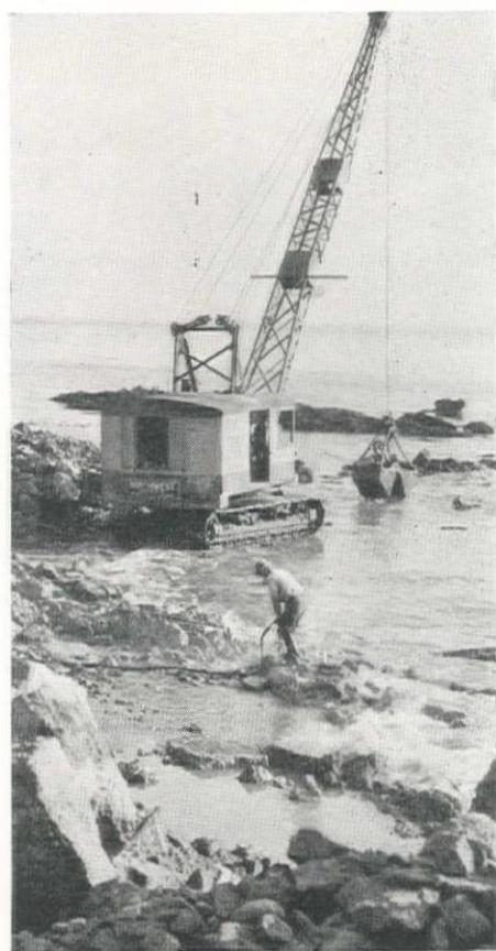
Across the beach from the tunnel portal this excavation marks the start of the work for the mile-long submerged outfall. Operations include digging a trench through soft rock and building a working trestle.
