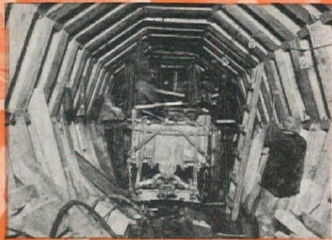
Tunnel No. 5—Station 178, working in wet sand—Owyhee project in Oregon and Idaho—an \$18,000,000 irrigation project.
