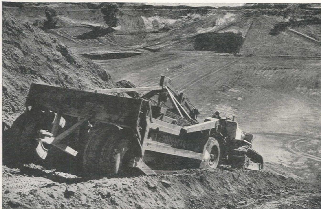
12-yard Carryall hauling down a steep grade onto the fill at Calero Dam.
