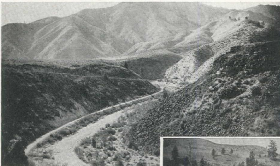
In this section of the canyon the railroad location forced the subsequent county road to climb out at various points. Note the road climbing the far side of the canyon on a steep grade.
