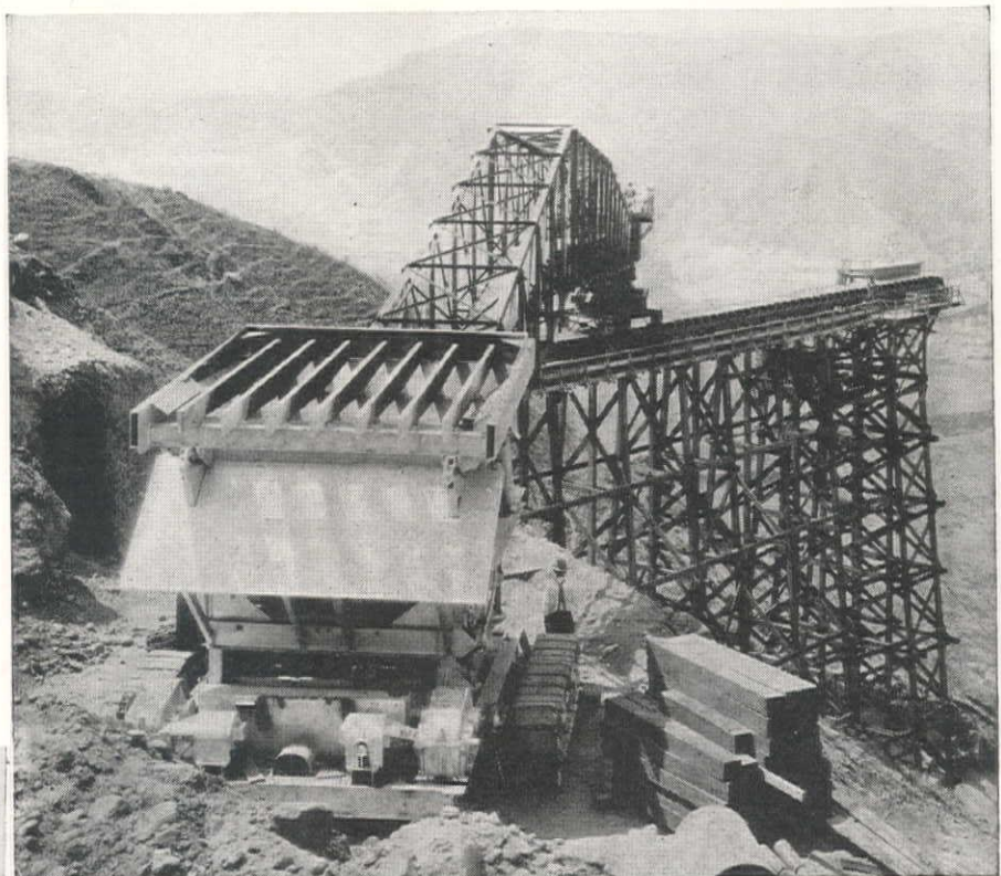
Grizzly at the pit with 16-in. spacing feeds the 42-in. belt on the movable boom. This grizzly is crawler mounted and moves with the shovel; loading is direct, without intermediate haul. Hinges at one side and hydraulic jacks at the other permit the grizzly to be tilted to dump off the oversize material.
