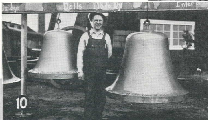
10—Navigation bells which will be placed on the piers of the San Francisco—Oakland Bay Bridge. The larger one weighs 3,000 pounds.
