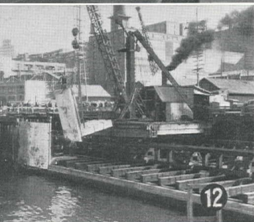
12—Setting one of the precast concrete slabs in the Seattle seawall, which has a length of 6,000 feet.
