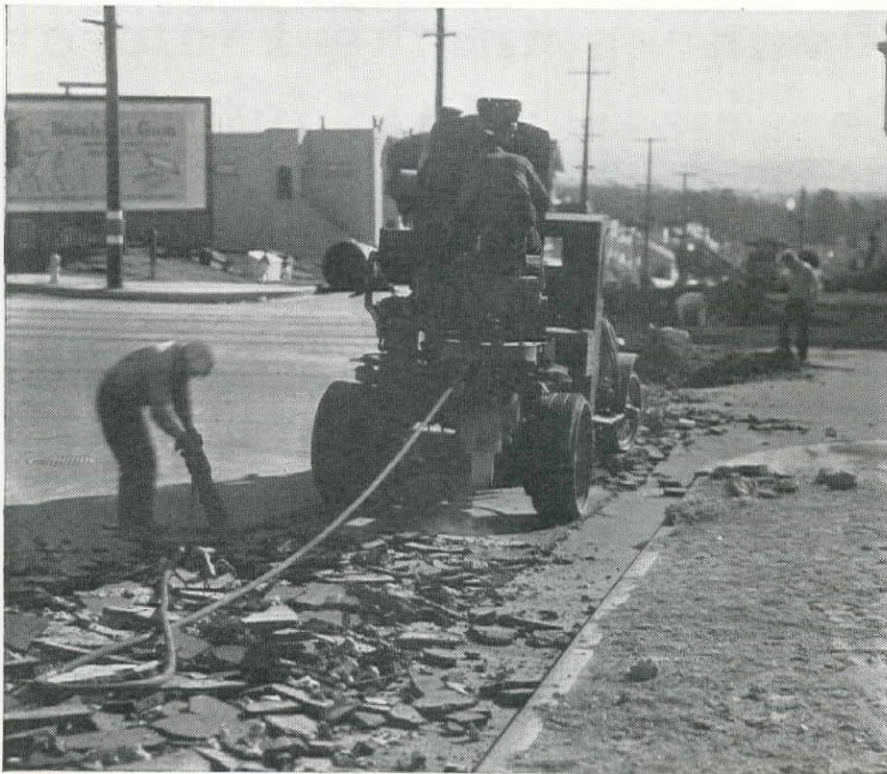
Examples of the use of mechanical equipment in the construction of distribution systems, where hand labor was used almost exclusively in 1920.
