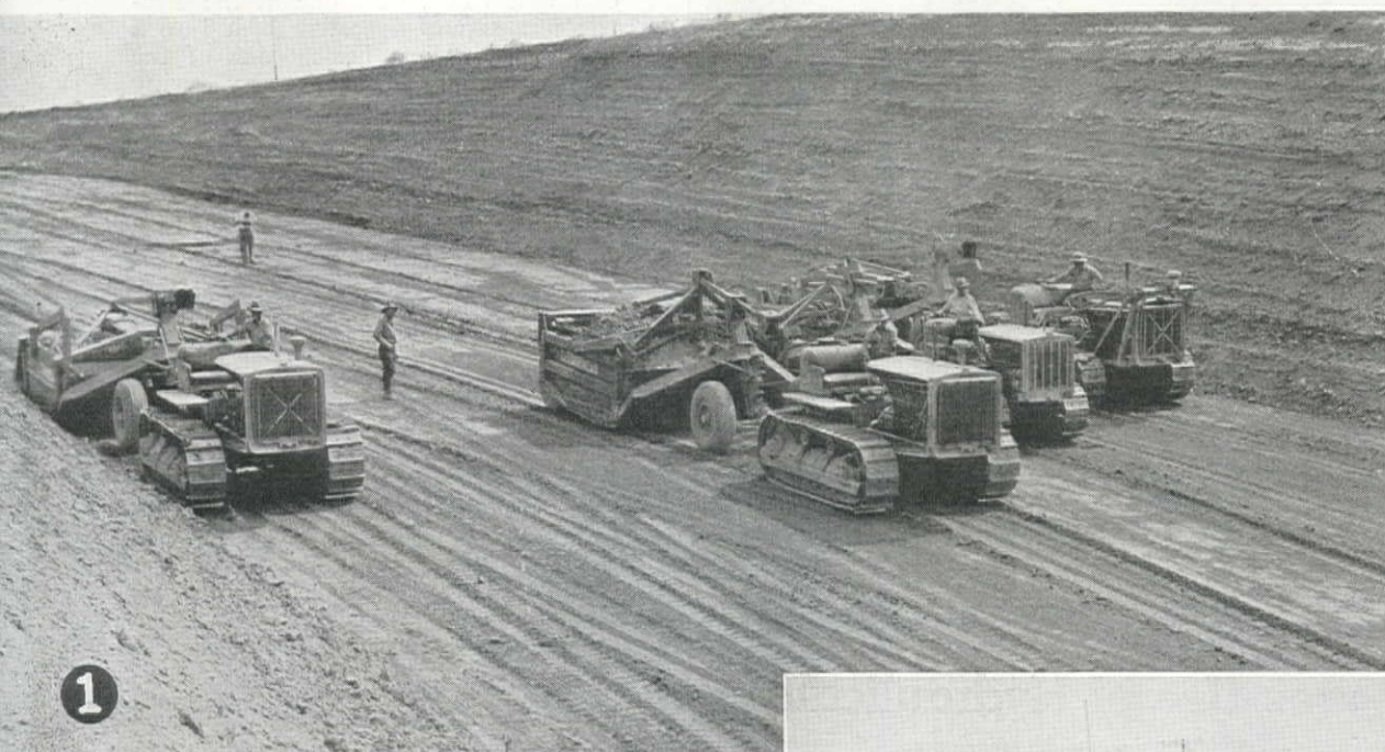
1—On the plains where Buffalo Bill chased Indians, the Taggart Construction Company are using Caterpillar and LeTourneau equipment on this highway grading job near Cody, Wyoming.
