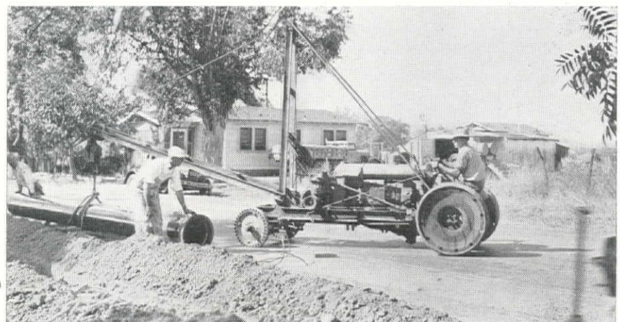
W. J. Tobin, contractor (above), used this crawler-mounted machine to handle 16-in. cement-lined cast iron pipe on a job for the San Francisco Water Department. At Gilroy (below) this tractor-mounted machine was used to place 16-in. pipe in the trench.
