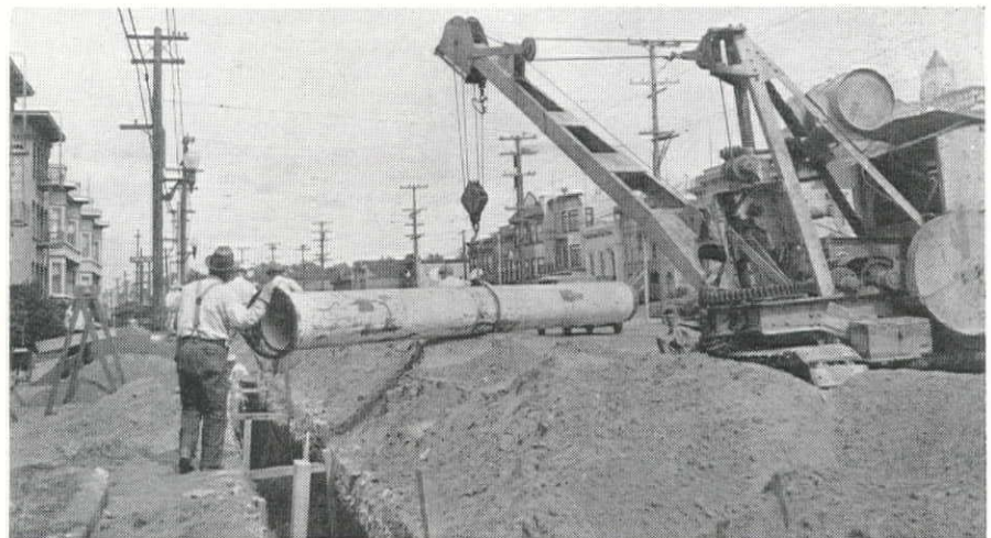
W. J. Tobin, contractor (above), used this crawler-mounted machine to handle 16-in. cement-lined cast iron pipe on a job for the San Francisco Water Department. At Gilroy (below) this tractor-mounted machine was used to place 16-in. pipe in the trench.
