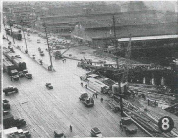
8—Seattle's seawall project nears completion. The record for slab setting has been eleven in six hours, and eighty-one batter piles have been driven in six hours.
