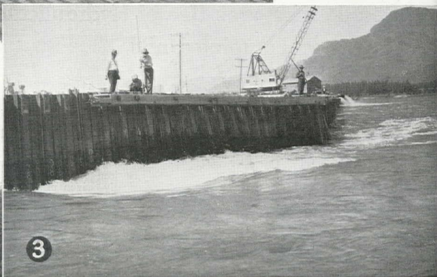
3—On the river side of the main cofferdam at Bonneville, following the high water season. This area was unwatered in August by the Columbia Construction Company.
