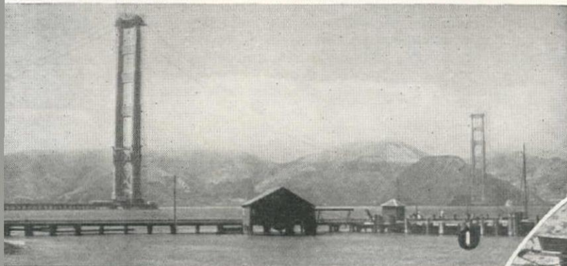
1—Lost in the fog, the cables to support the catwalks now span the 4,200-ft. distance between the towers of the Golden Gate Bridge.
