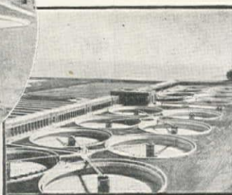
CLEVELAND—16—112 ft. round Dorr Sifeeds—activated sludge.
