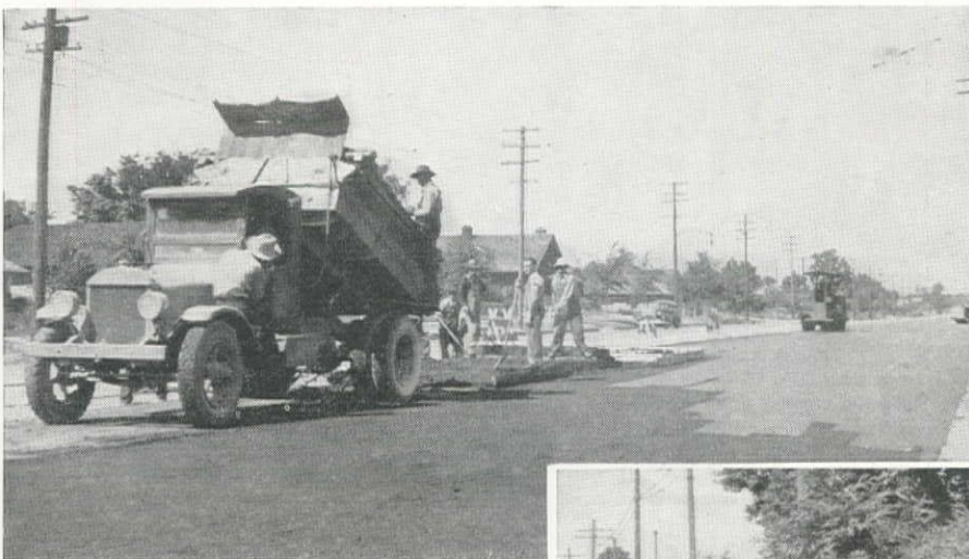
Complete equipment used to spread sheet asphalt on recent Utah highway work, consisting of only a truck-drawn, timber drag, followed by rolling. Note the width of street being resurfaced.
