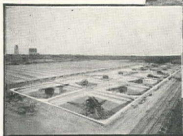
CHICAGO—15—97 ft. square Dorr Sifeeds: 32—126 ft. round ones on order—both activated sludge.
