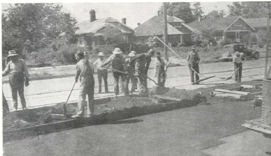
A crew of four men rides the drag for weight and to shovel the material evenly across the strike-off members.
