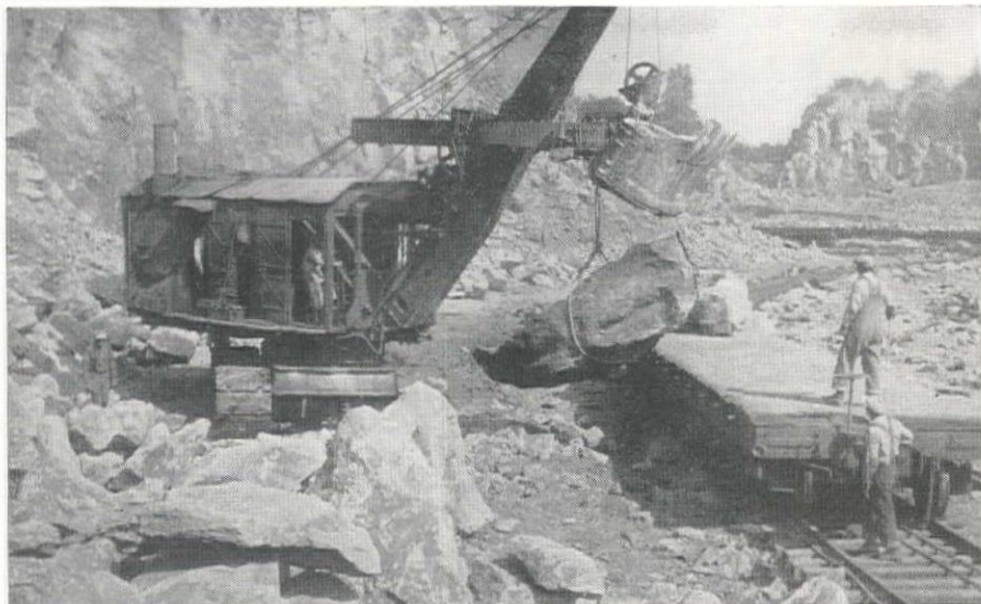
Fig. 7—Loading rocks in the quarry with a Bucyrus-Erie shovel and a sling. The average carload of rock weighs 56 tons.
