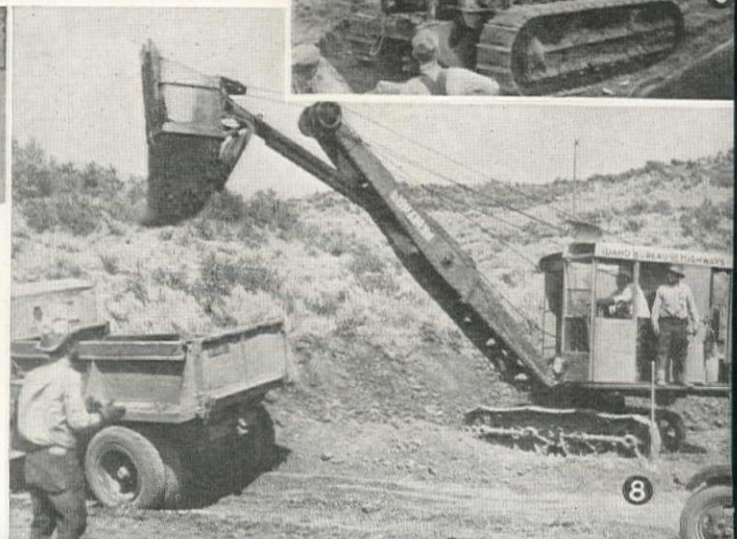
8—The Idaho Bureau of Roads recently started this Lorain 30 shovel on borrow pit work and, according to report, it was moving 600 yds. in an 8-hr. day.
