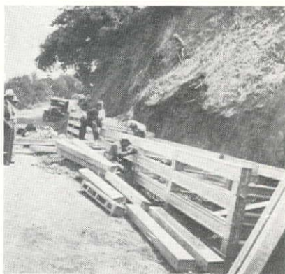
Assembling the crib wall with work-relief labor, under the direction of a skilled foreman.
