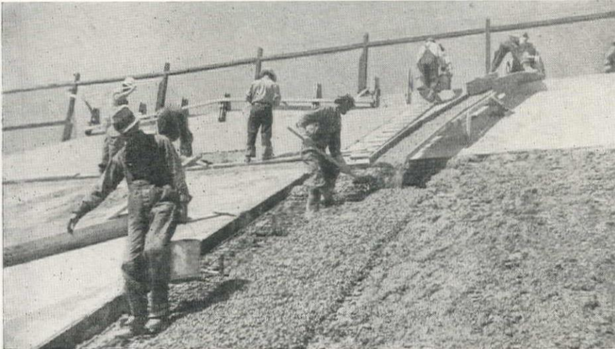
Concrete on the slopes was chuted directly into place followed by finishing operations.
