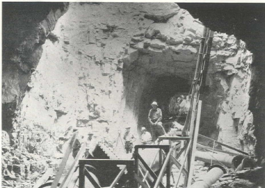
At the gate-chamber junction between the outlet-diversion tunnel and the operating shaft. The pipe for the Ogden municipal supply is shown ready to be encased in the concrete of the floor. The delivery pipe from the Pumpcrete unit can be seen coming down the shaft.
