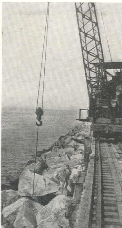
Fig. 4—Trimming the side slopes with a 50-ton Browning crane using a sling to adjust the large rocks.
