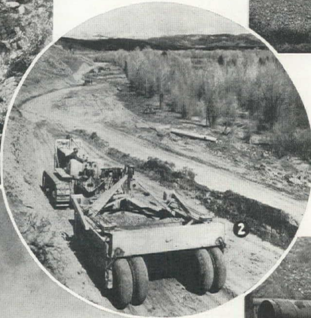
3—Dumping rock into the upstream toe of the Fort Peck dam. This rock is brought in a distance of 70 miles.
