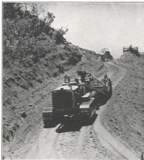
Moving 900,000 yards of excavation, 1,225,000 station yards of overhaul at San Marcos.
