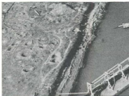
One of the dredges (lower left) in operation showing the 28-in. discharge line extending to the booster plant at the far bank and the land line extending to the dam in the background. Note the small pontoons carrying the power cable from the shore.
