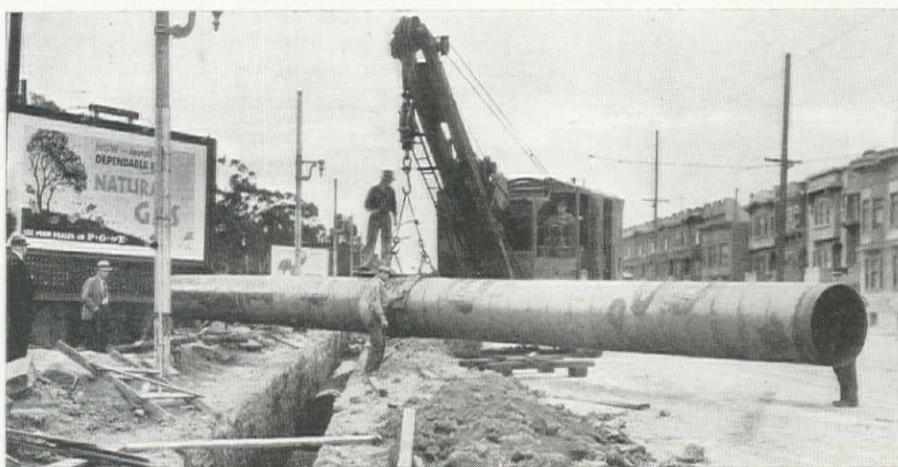
Handling a 60-ft. length of 44-in. pipe on one of the new connections in the distribution system. This pipe was reclaimed from the emergency connection to the East Bay District system laid several years ago.
