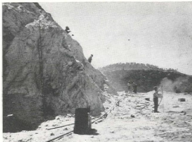
Tamping Halifax Free Flow into holes varying in depth from 5 feet to 18 feet, with 7-foot to 12-foot centers.
