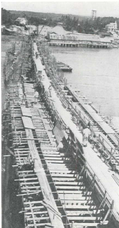
Extensive falsework for the Suislaw River bridge which is 1,650 ft. long, featuring two 156-ft. tied concrete arches.
