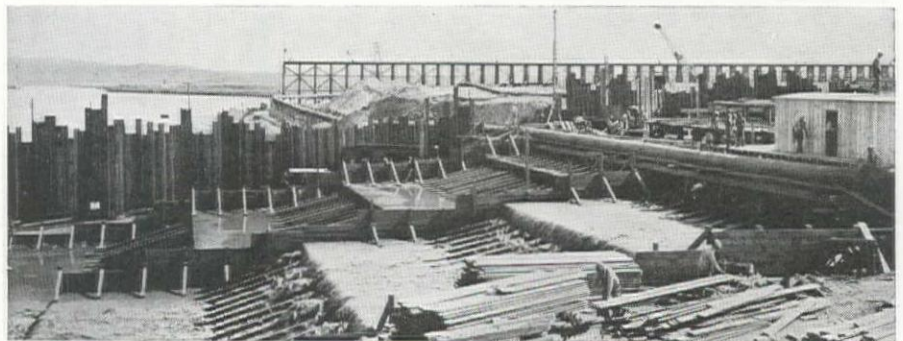
Timber spillway passing the discharge from the core pool over the sand plug. These are built in pairs and one is raised while the other is in use. The sheet pile cutoff is immediately behind the second spillway.
