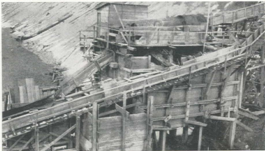
Built at the foot of a high gravel bank of the Cle Elum River, the aggregate plant was fed raw material by sluicing operations from the flume at the right.
