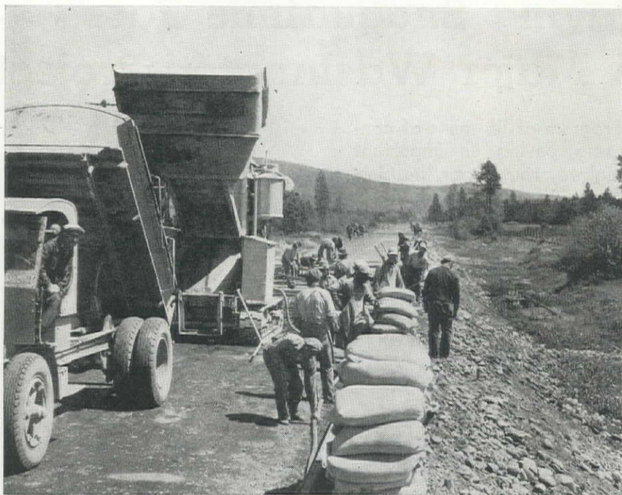
Three compartment trucks supplied batched aggregate to the mixer, with sacked cement added in the hopper. Mixer water was pumped from nearby streams or irrigation ditches.
