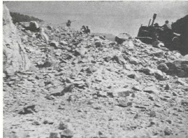
Note indications of excellent fragmentation and size of rock for workable shovel loading.
