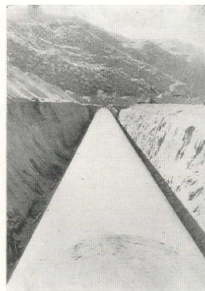
Fig. 4—Completed aqueduct conduit before backfilling, showing whitewashed surface.
