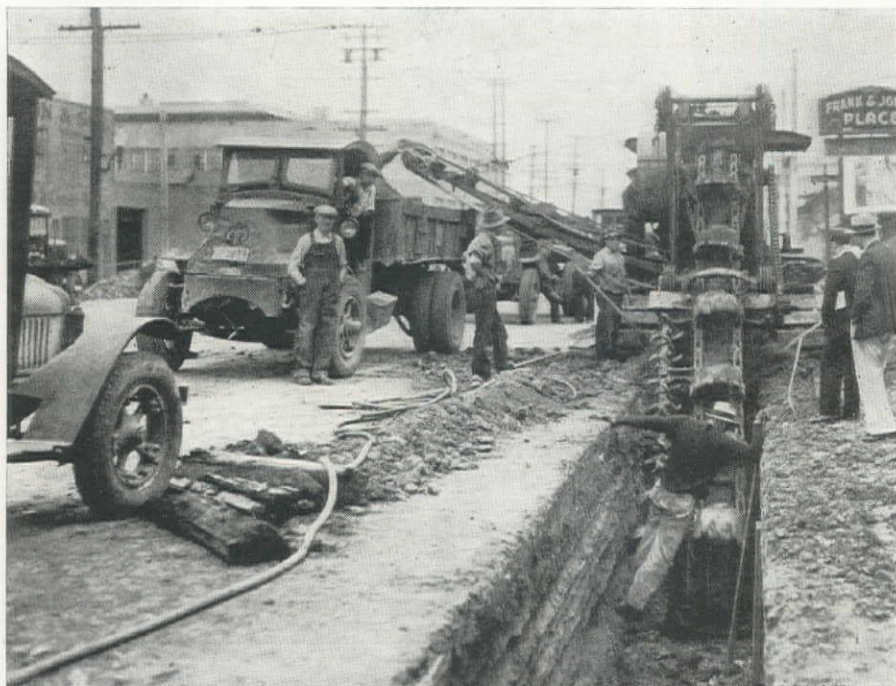
Typical trenching operations for the cast iron mains which were added to improve the grid system and supplement the existing distribution lines. About 80 mi. of 6 and 8-in. mains have been laid in the present program.
