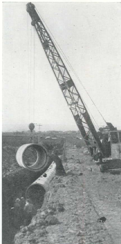
Laying 62-in. Lock Joint type of concrete pipe on the Bay Crossing project with a Link Belt crane.
