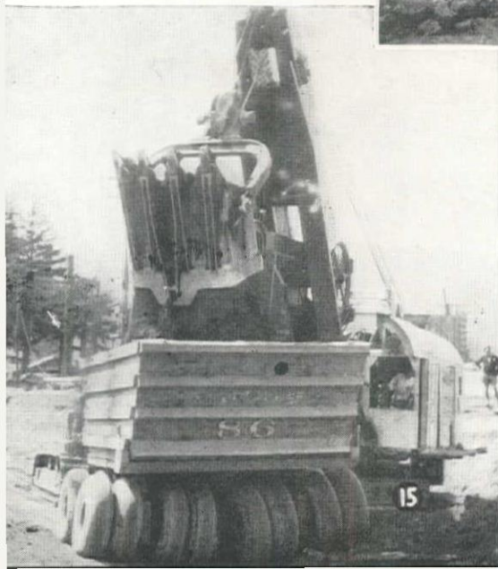
15—On Bonneville dam excavation work this 30-yd. Le Tourneau buggy indicates the action of the oscillating axles in distributing the load on the sixteen 13.5 x 20 tires.
