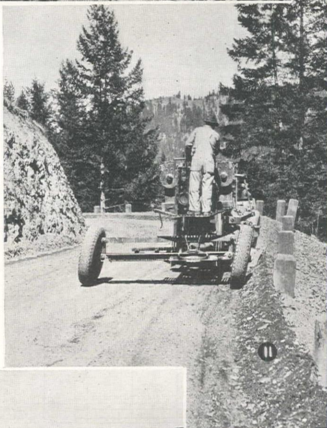
11—On the Blewitt Pass route over the Cascade Mountains in Washington the state highway department uses an Adams Leaning Wheel Grader for maintenance work. The grader is mounted on balloon tires.
