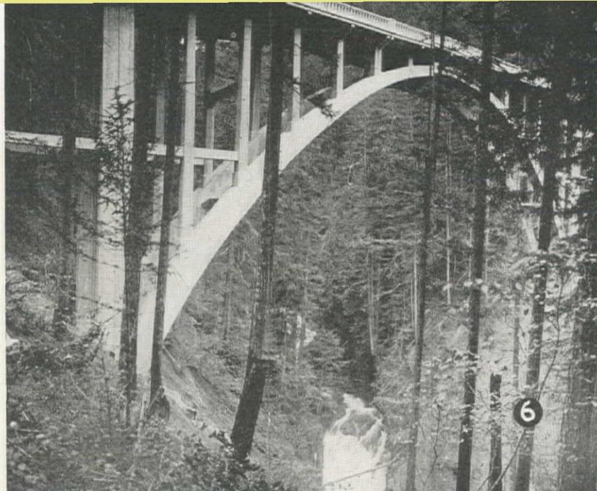
6—Cartright Creek bridge, on the Randle-Yakima National Forest Highway in Lewis County Wash., is a 200-ft. open spandrel arch with the deck 180 ft. above the stream. The structure was built by the Western Construction Co., Seattle, for the Bureau of Public Roads.
