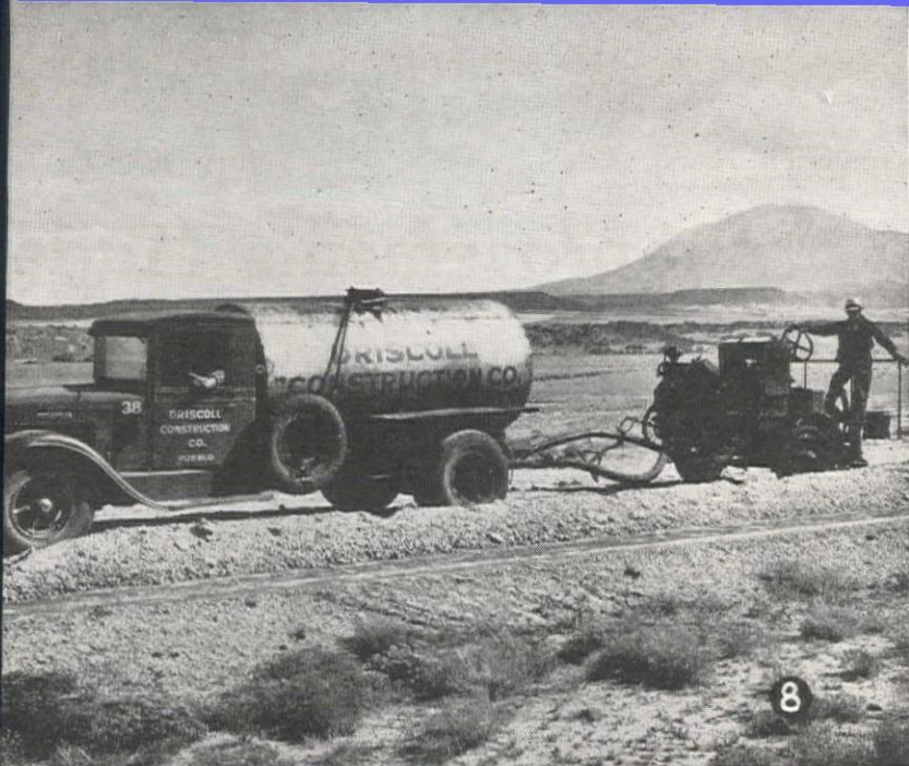
8—On a highway job near Walsenburg, Colo., the Driscoll Construction Co. used a 1000-gallon tank mounted on an International truck to deliver road oil.
