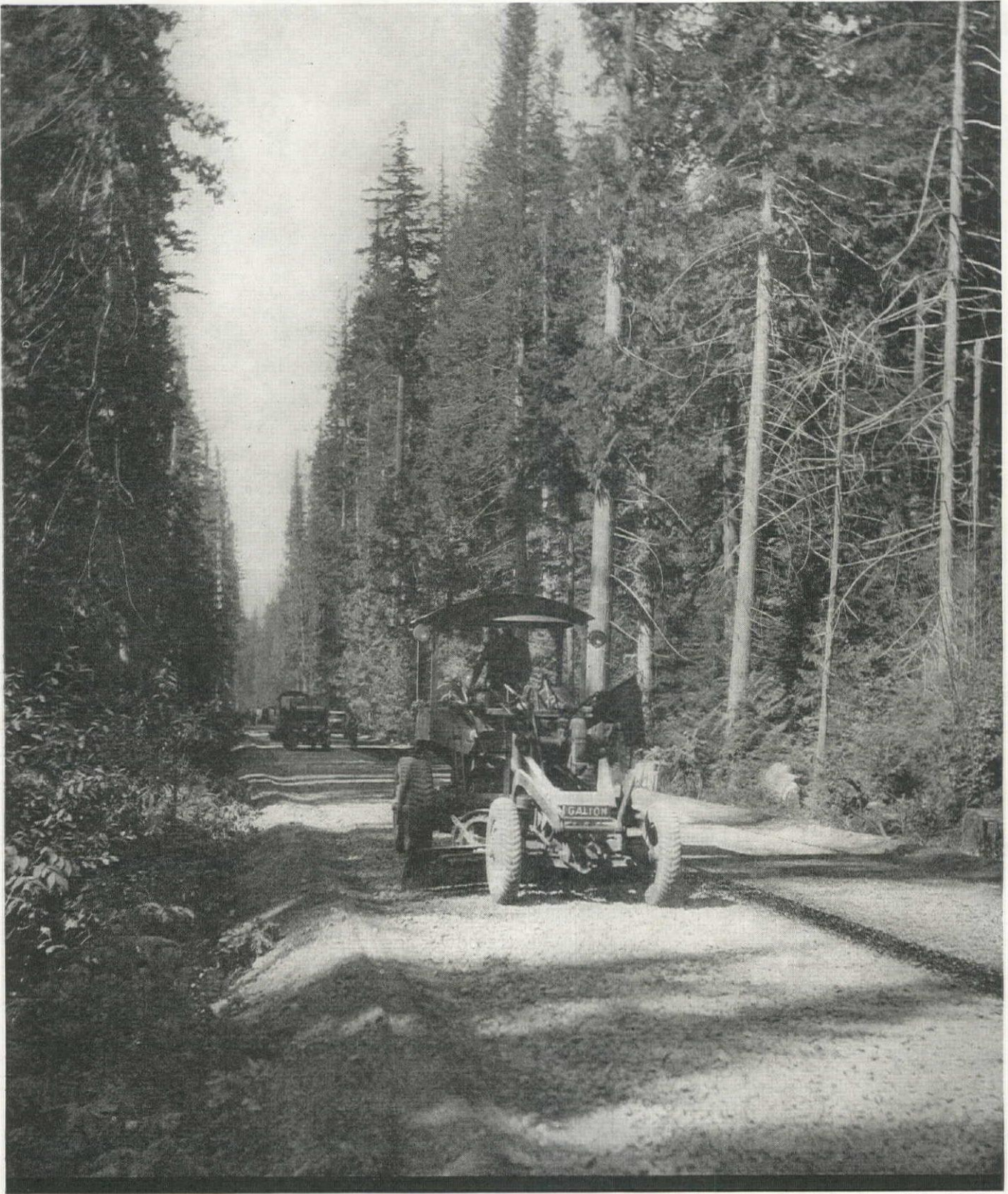
A Galion Motor Patrol Grader with Double Drive leveling off crushed stone surface on a highway in the West.
