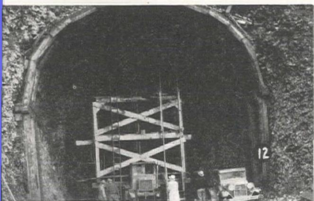
12—A truck-mounted, full face drill carriage was used by the Orino-Bell-Malcom Co. in driving the Tooth Rock tunnel for the OWR&N track relocation on the Bonneville project. A 10-ft round was pulled in driving.
