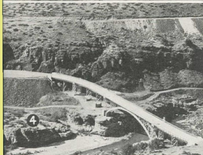
4—Salt River bridge, 40 miles east of Globe, Ariz., includes a two-hinged arch as the main unit in the 455-ft. length of structure. R. A. Hoffman is state bridge engineer.
