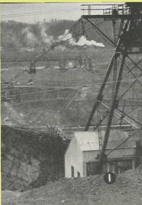
1—Cableway tower used by the General-Shea Co. in building the powerhouse and lock for the Bonneville project. Two of these 15-ton cableways were used for concrete placing.
