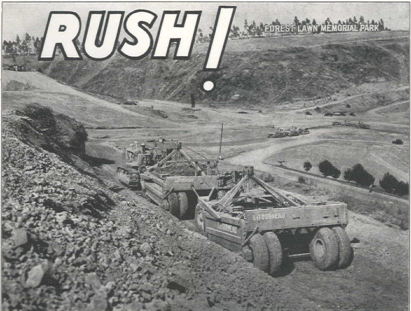
Picking Up a Big Load—Rolling double takes no more tractor power here, but yardage is increased about 60%.
