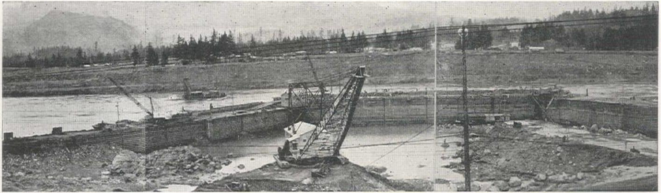
Fig. 2. Timber crib cofferdam for the main, or spillway, dam in the north channel during March, before the high water season. Excavation under way with the 8-yd. Monighan dragline.
