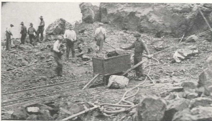
Quarrying on the rich vein of rock asphalt, which is shot out in large pieces and then broken up by air hammers and loaded by hand.
