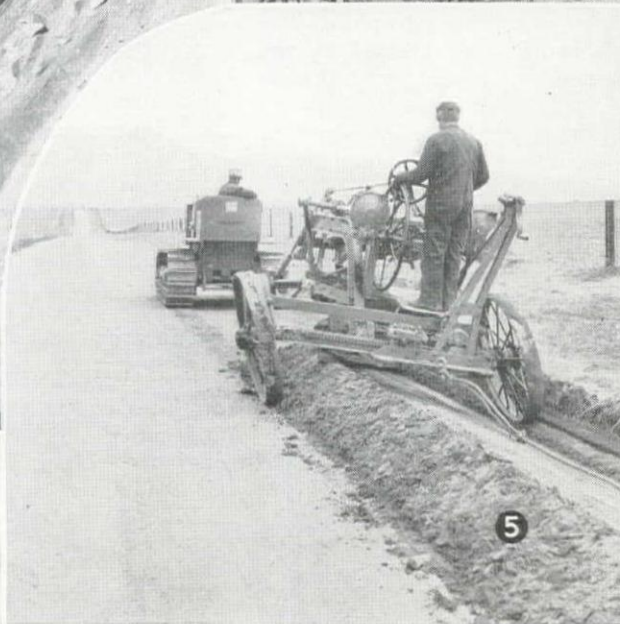
6—In Kittitas County, Washington, Albertson Cornell Bros., contractors, are laying an 8-mile length of 20-ft. portland cement concrete paving on the Sunset Highway.
