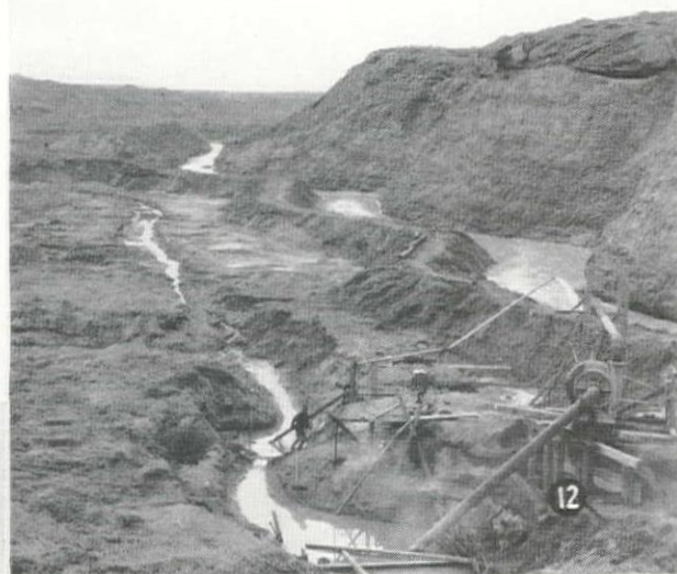
13—Draglines of W. E. Callahan Construction Co. and Gunther and Shirley at work excavating along the All-American Canal project at the eastern edge of the Sand Hill section.
