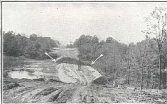
The blast. Note absence of Fill throwing. Gases are properly confined to push mud laterally from under Fill
