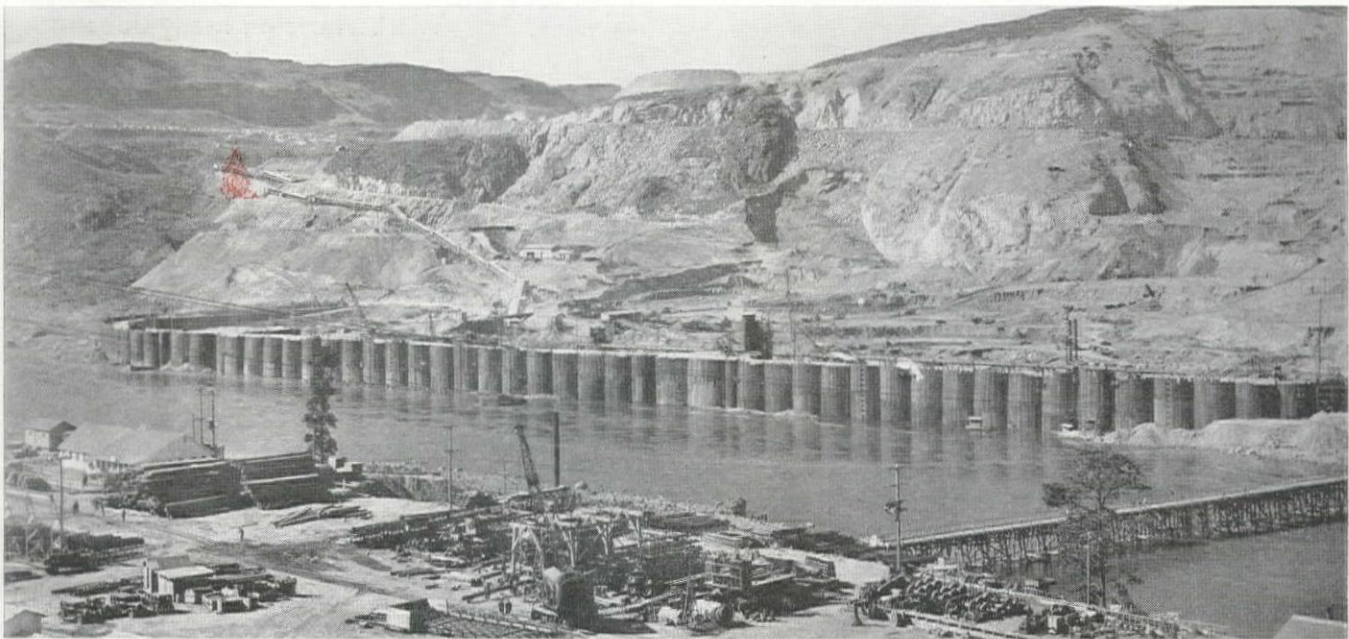
Cellular cofferdam on the west side of the Grand Coulee dam site.
