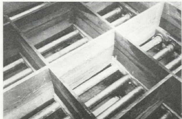
Timber compartments about 2\frac{1}{2} ft. square are used in the bottom of the filters to keep the gravel from moving during the washing operations.
