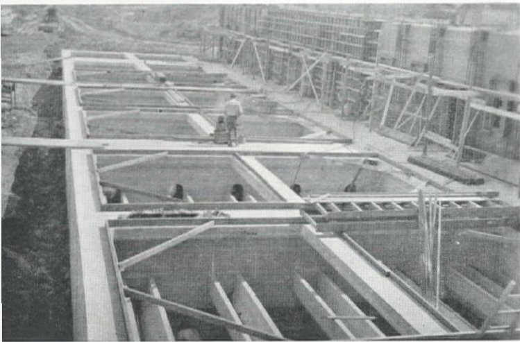
Completed filter units showing wash water troughs in place and ready for placing the filtering material.
