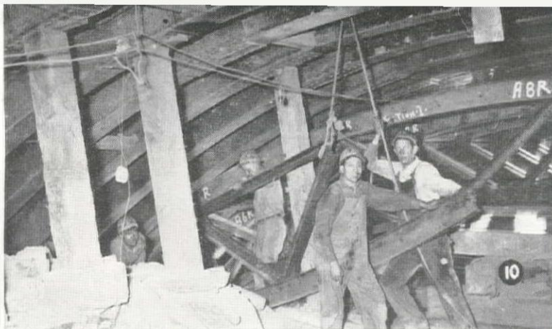
10—In the Yerba Buena tunnel of the San Francisco-Oakland Bay Bridge project, steel trusses are being placed to support steel arch forms for the tunnel lining of concrete.
