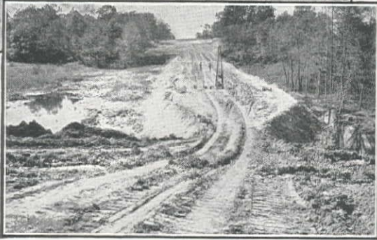
Wiring up Electric Blasting Caps for Fill Settlement Shot
