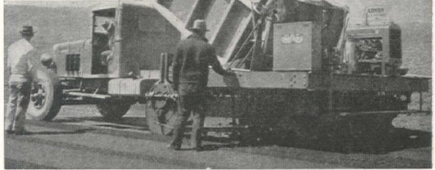
Truck being pushed along by paving machine as it discharges load of bituminous-mix surfacing.
