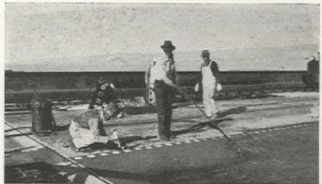
Spraying Hunt process curing compound on finished concrete surface. Workman at left is adjusting and finishing concrete around traffic lane marker laid previously with template shown in background.
