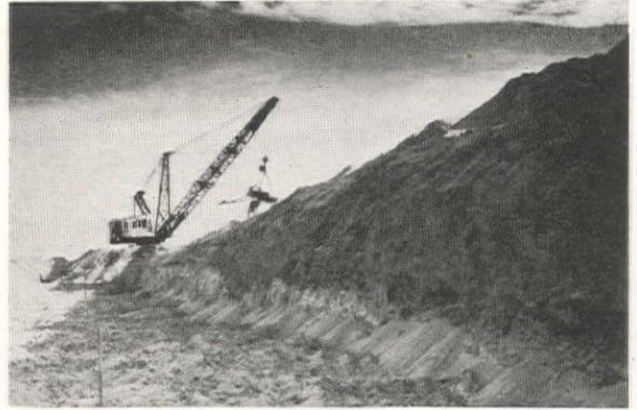
Fig. 1—A Bucyrus-Erie 100-B Dragline Equipped with 4-yd. Bucket and 90-ft. Boom Excavating Conduit Trench on Schedule 3.
