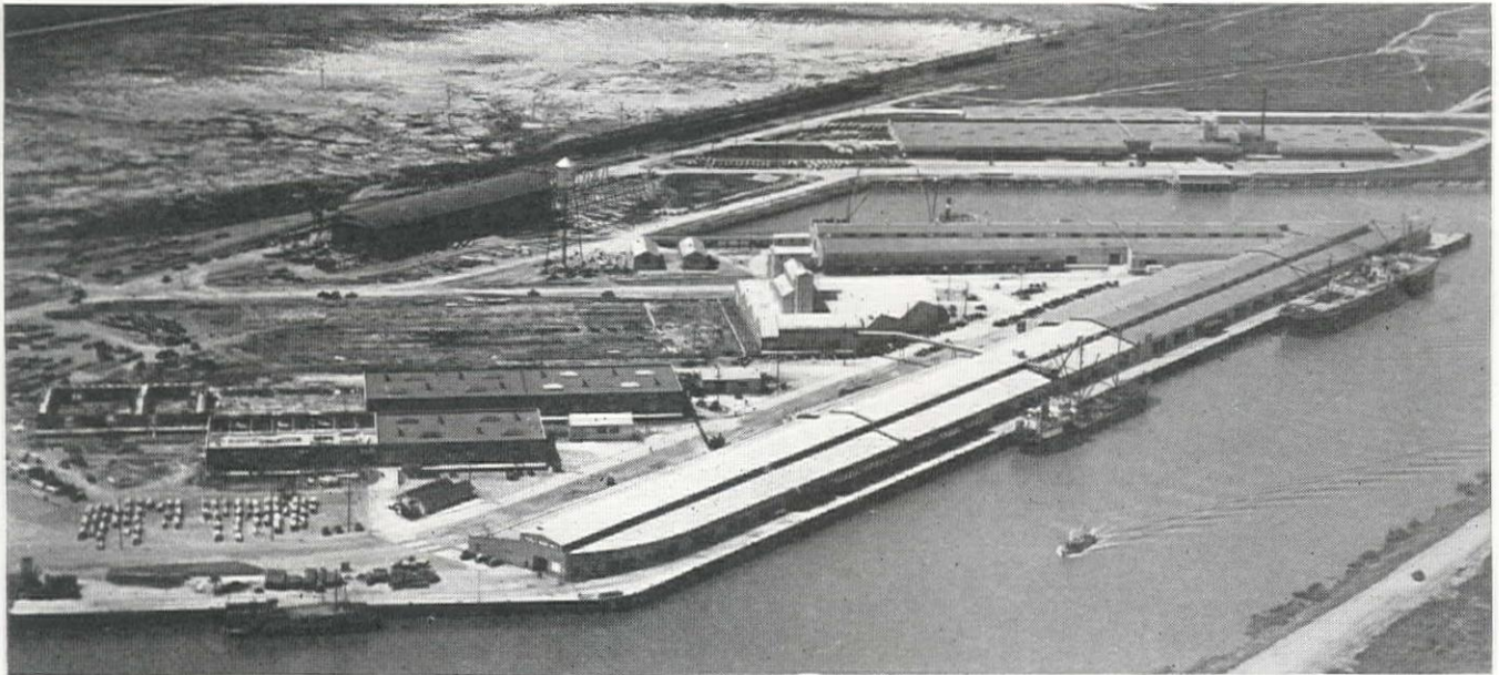
Airview Showing Transit Sheds 3 and 4 Recently Completed in the Foreground with a Combined Length of 930 ft. and an Area of 123,900 sq. ft.
