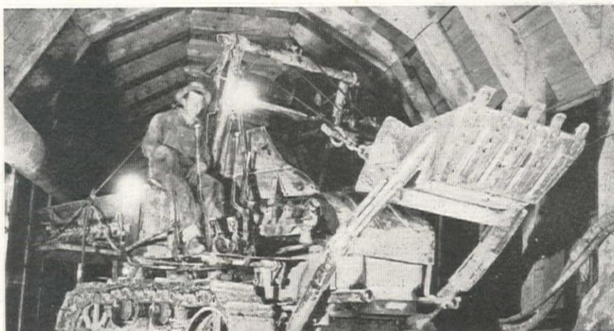
Mounted on a 60 Caterpillar Tractor, This Electrically Operated Mucking Machine, Built Under the Direction of Everett Seabury, Superintendent, Handled a 10-ft. Round (16-ft. Diameter Tunnel) in About 3 Hours.
