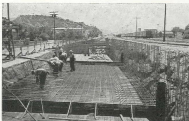
A Section of Reinforced Concrete Closed Conduit in the Work at Nogales Presented Problems Because of the Adjacent Railroad.
