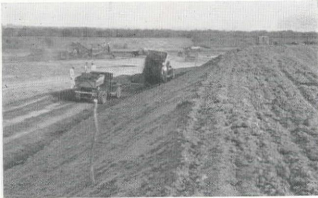
On the Lower River Near Brownsville, Texas, Levee Construction Is the Main Part of the Work.
