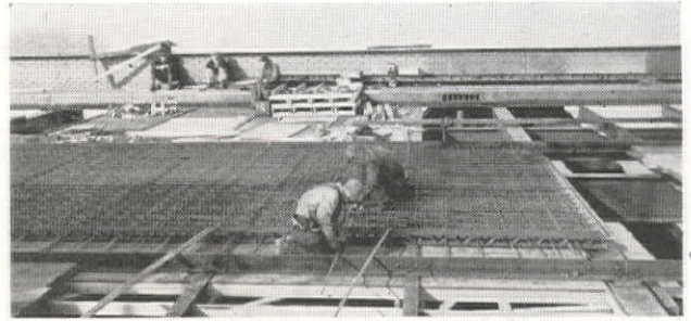
Placing reinforcing steel for upper deck floor. Steel angles forming longitudinal expansion joint and plywood forms are shown in foreground.
