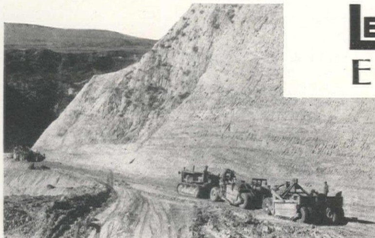
Over the Jack Rabbit Trail (above) with 65 yards an hour on a 4000-foot round trip. A LeTourneau Angledozer (below) cuts a fire trail out of a mountain side and makes a forest safe at North Fork, California.
