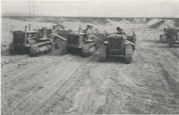
Fig. 2—In Rough Terrain on Schedule 3, LeTourneau Scrapers and Ripper Are Used to Pioneer Deeper Cuts and Prepare a Flat Sub-Grade for 4-yd. Dragline to Operate On.
