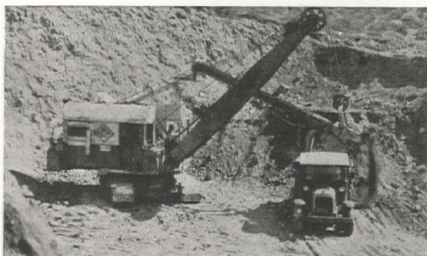
Fig. 10—One of the Few Shovels Used on Trenching Work at Work on Conduit Excavation on Schedule 20.
