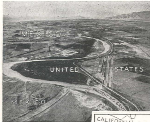
River Cutoffs Which Transferred Land Between the United States and Mexico will be eliminated with completion of the present river control work. View Shows Channel Straightening Near El Paso.
