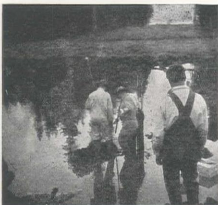
Loading Holes for Mat Shooting Along Line of Fill Indicated by Clearing in Timber Ahead.
