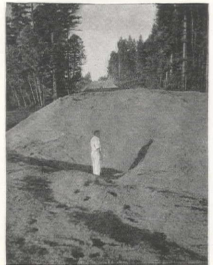
The Extent of Surface Settlement Occurring When Under Fill Shots Force the Underlying Muck Out to the Side Is Shown by the Relative Size of Man Standing in the Depression.
