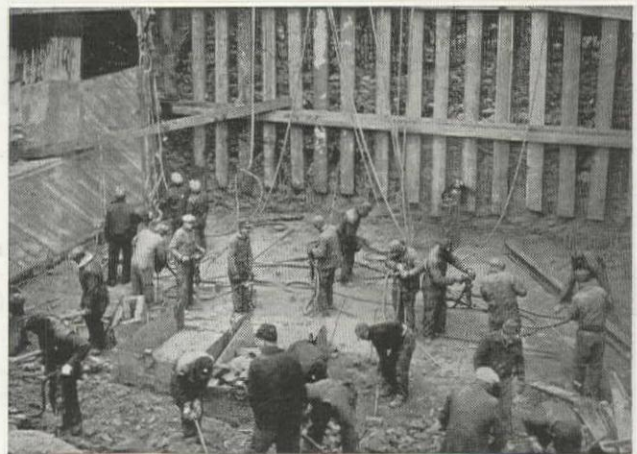
Excavating Through Bearpaw Shale with Air Drills and Chippers for Foundation of Unit Block in Concrete Headwall.
