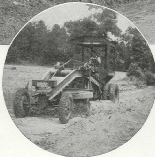
Adams Motor Grader—2-wheel Drive—reshaping a dirt road.
