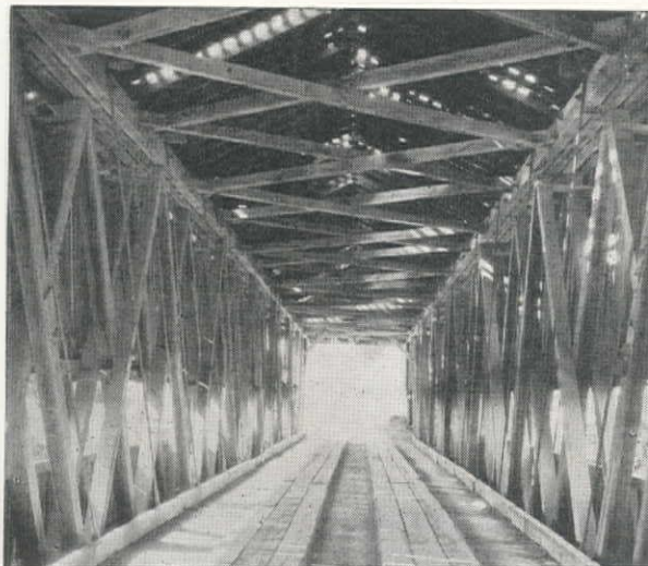
REDWOOD (below)—Service Life—Over 40 Years. Built about 1890, replaced in 1933. New highway required. Wider roadway, heavier loadings.
