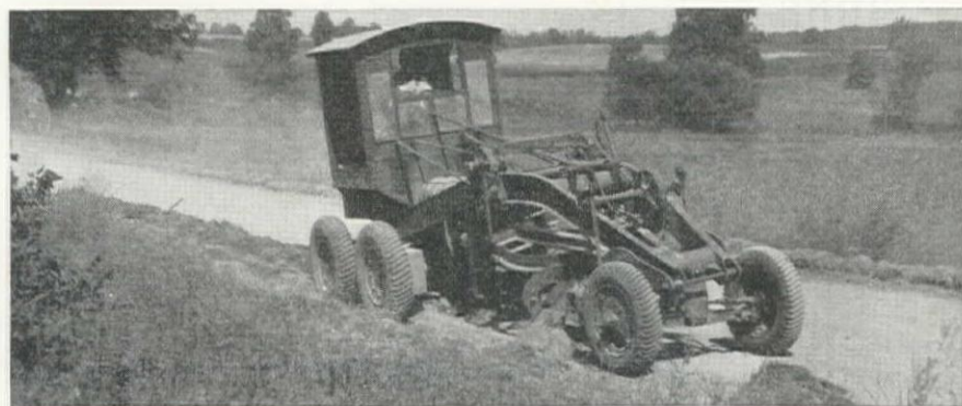
Adams Motor Grader—4-wheel Tandem Drive—reditching a gravel road.
