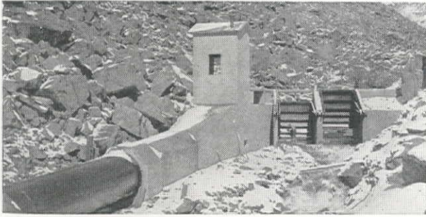
Intake Structure on Clear Creek Showing 10 by 10-ft Radial Gate, the Right One Being Partially Open.
