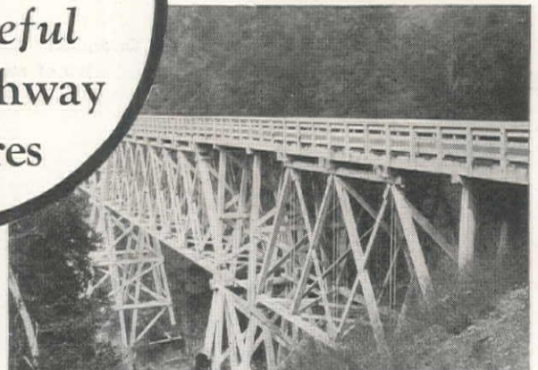
REDWOOD—Service Life on main Highway—15 years. Built in 1917, highway relocated in 1932.
