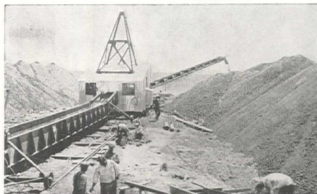
Disposal End of Jeffrey Belt Conveyor System Extending 2000 ft. from Upper Portal Showing Method of Extending Stacker Unit Over Dump by Mounting Last Section of Belt Conveyor on a Track Carriage.
