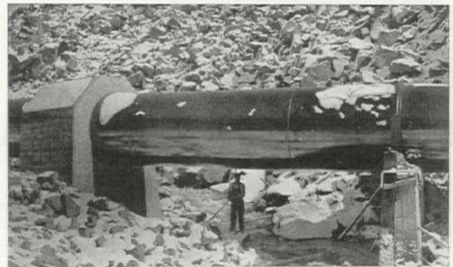
A 35-ft. Span Over Willow Creek Showing Anchor and Pipe Support.
