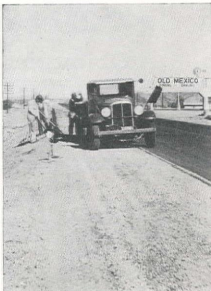
Maintenance Crews Building Asphalt Pre-Mix Berm Along Edge of Roadway Shoulder.
