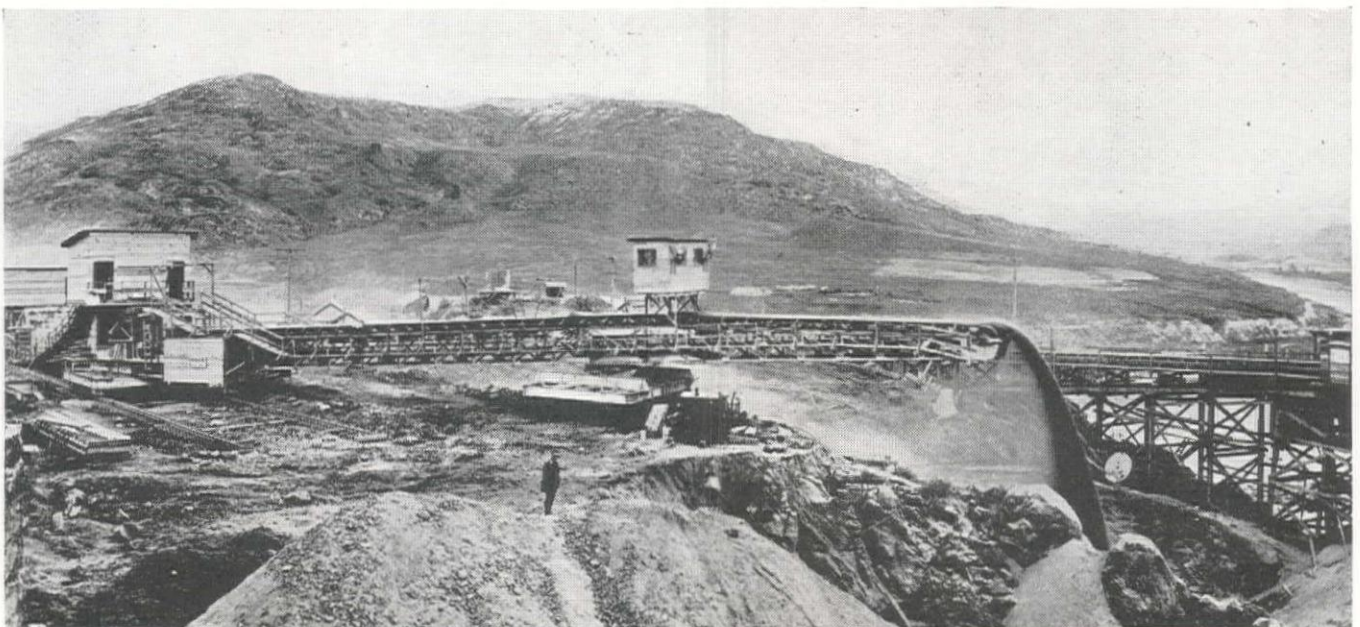
The Stacker Unit at the End of the 60-in. Conveyor System Dumping Material Into Rattle Snake Canyon.
