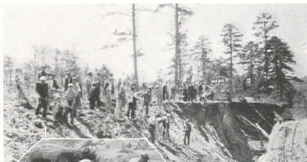
(Upper) Grading Sides of Deep Gully Preparatory to Planting Controlled Vegetation. (Center) Constructing a Rubble Masonry Check Dam for Gully Control. (Lower) A Diversion Dam Constructed for Erosion and Flood Control on Gila River Project in Graham County, Arizona.
