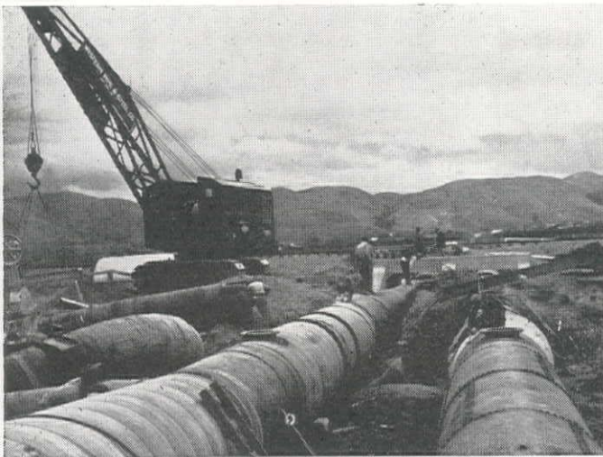
(Left) Pipe Lines No. 1 and 2 Passing Under Western Pacific R. R. Near Irvington. (Right) Unloading 66-in. Steel Pipe Sections Near Redwood City With a Special Crane Mounted on a Caterpillar '60' Tractor.
