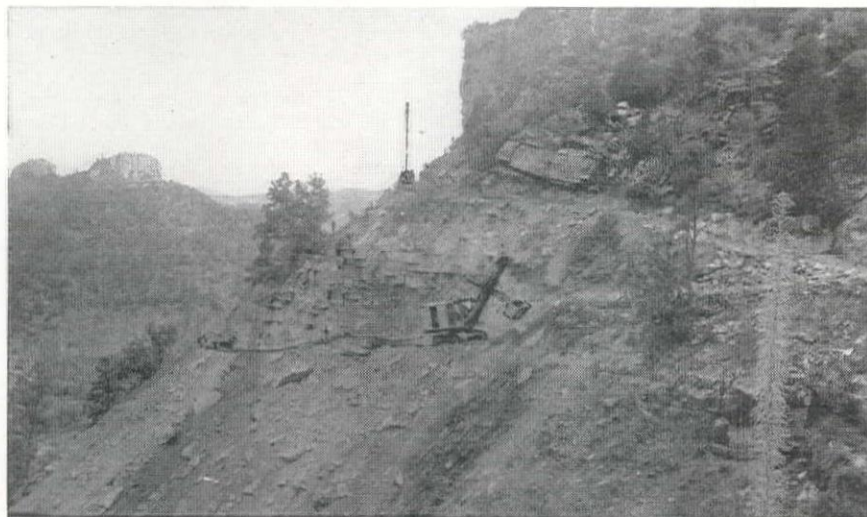
Opening Up a Pioneer Road Around Heavy Rock Cut. Note Wellrig Drilling Blast Holes at Top of Cut Above Shovel.
