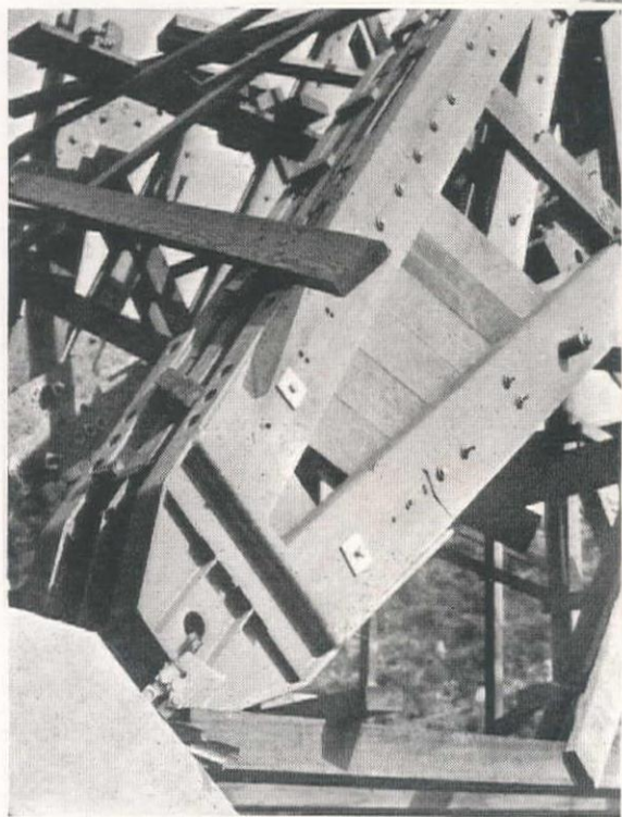
Lower Hinge Detail
