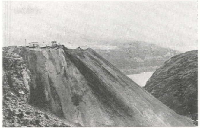
A View of the Waste Dump in Rattle Snake Canyon With Stacker Unit Discharging Material Over Slope.
