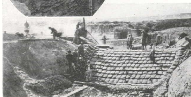
(Upper) Grading Sides of Deep Gully Preparatory to Planting Controlled Vegetation. (Center) Constructing a Rubble Masonry Check Dam for Gully Control. (Lower) A Diversion Dam Constructed for Erosion and Flood Control on Gila River Project in Graham County, Arizona.
