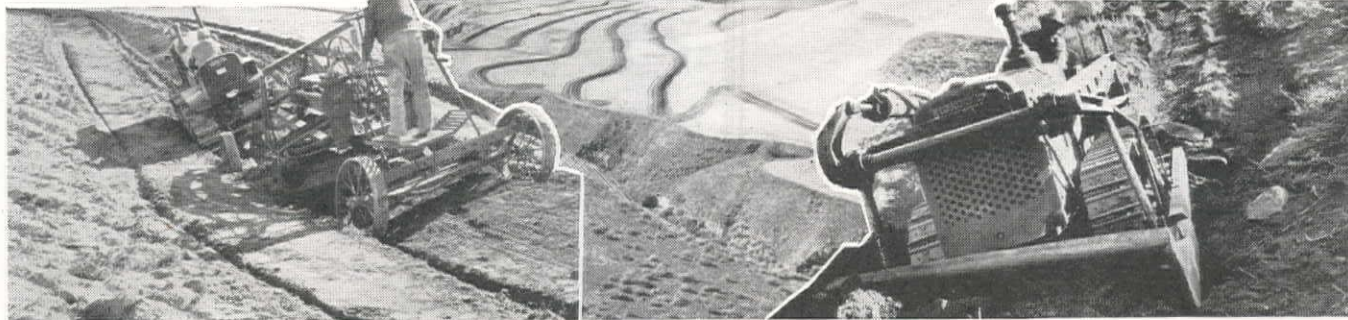
Terracing a Hillside on an Experimental CCC Erosion Project in Wasatch Mountains in Utah With a McCormick-Deering T40 Tractor and a Trail Builder.
