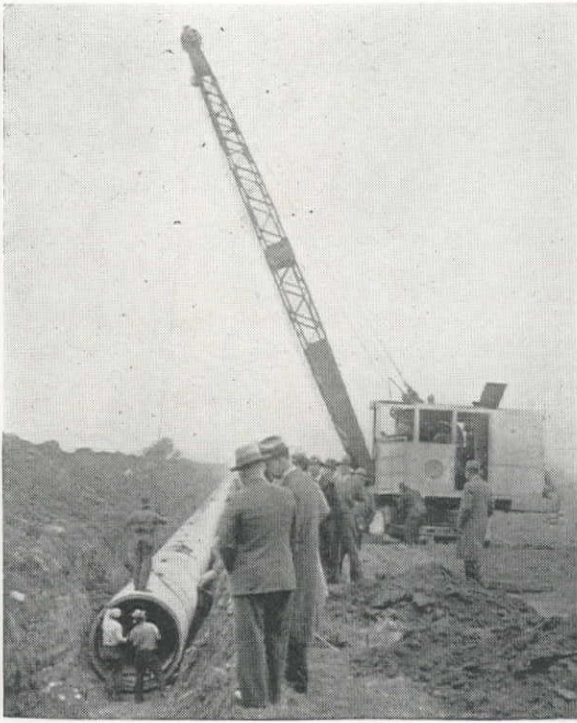
Laying 62-in. Concrete Pipe With a Link-Belt K44 Crane Near Newark.
