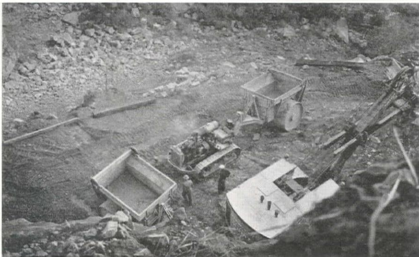
Loading 12-yd. Carts With Bucyrus-Erie 43-B Shovel. These Carts, Designed by W. E. Orr, Have 3-ft. Wide Steel Wheels Which Act as Compaction Rollers on Fills.
