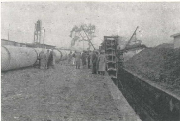
Excavating Trench for 66-in. Steel Pipe Near Fair Oaks with Type 'C' Buckeye Trenching Machine. Coated Pipe Ready for Installation Is Shown at Left.
