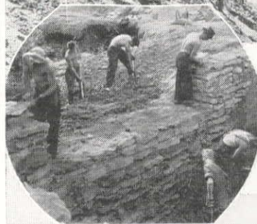
(Upper) Grading Sides of Deep Gully Preparatory to Planting Controlled Vegetation. (Center) Constructing a Rubble Masonry Check Dam for Gully Control. (Lower) A Diversion Dam Constructed for Erosion and Flood Control on Gila River Project in Graham County, Arizona.
