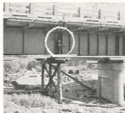
(Lower) Detail of Suspension Point in Girder Showing Overhanging Floor System Above.
