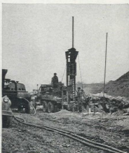
Truck-mounted augers drill 6 in. holes varying in depth from 20 to 35 ft. at the center of the cut. Rock ranges from soft shale through sandy shale to a firm sandstone.
