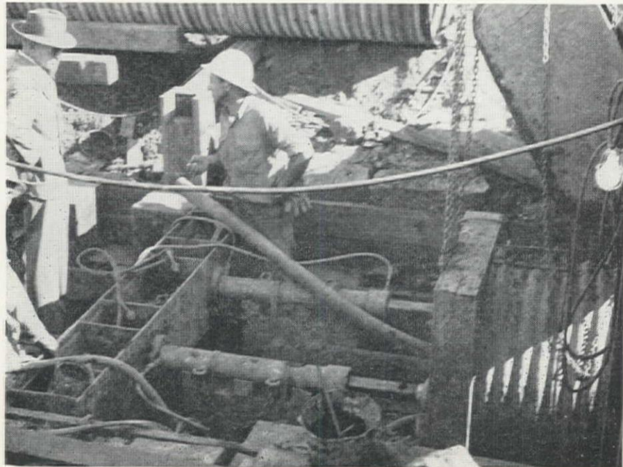
SETUP for one foot of progress per hour. Visible are backstops, movable jacking thrust block, the hydraulic jacks and oil lines leading from jacks to oil pump.
