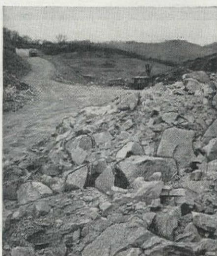
Results of plan have been reduced back break, decreased vibration and better fragmentation. Rock is well broken all along the cut, permitting faster, more economical removal.
