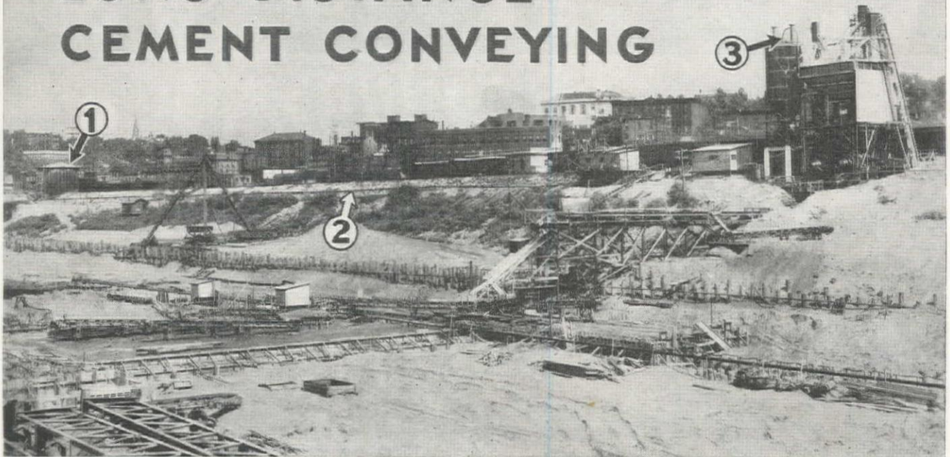
Concrete plant of John Griffiths & Son Co., on Mississippi River Lock No. 26. Bulk cement is pumped from barges to a storage bin (1). A 5" Type "A" Fuller-Kinyon Pump below the bin conveys the cement through a 4" transport line (2) a distance of 850 feet to the mixing plant (3). A second 5" pump, below the tracks is connected to the same pipe-line to unload cement delivered in hopper bottom cars.
