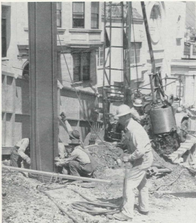
SETTING soldier beams at the east approach. Rig in background is drilling holes for the beams a number of feet below final sub-grade.
