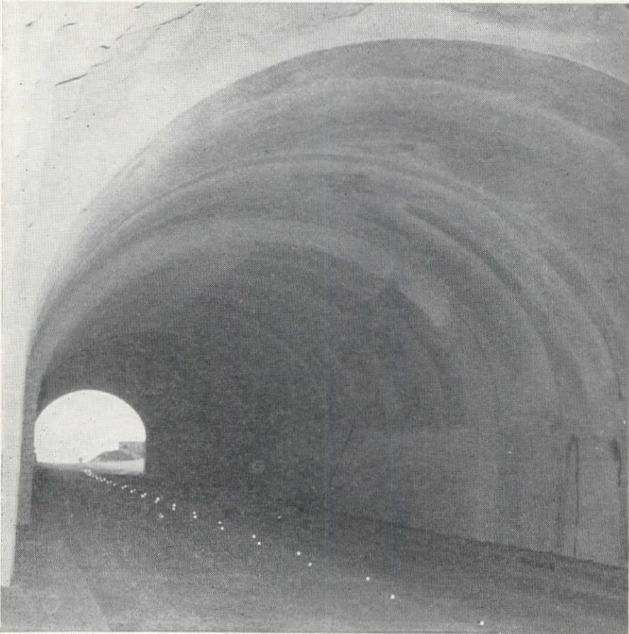
TOP—View of west portal. Jutting limestone ridge obstructed optimum alignment.
