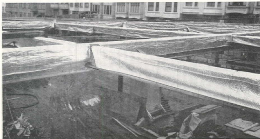
ALUMINUM PAINT, aluminum foil and wet burlap are being used to prevent high temperatures from causing strains in the steel network at the east approach.
