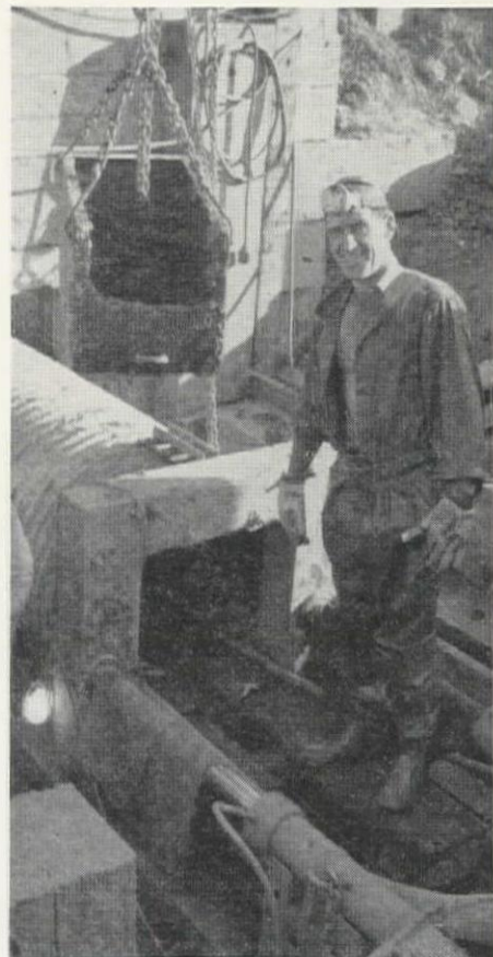
DIRT BUGGY in background was used to elevate muck from working pit. The working pit was excavated just long enough to handle the 20-ft. lengths of pipe.
