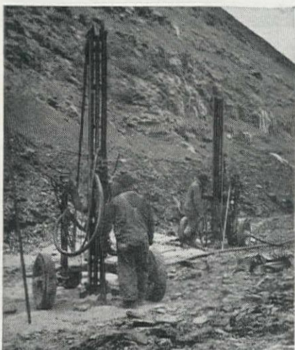
Wagon drills are used for 2½ and 3 in. diameter holes on slopes of the cut. Crews space holes on a 6 x 8 ft. pattern, drilling holes to depths varying up to 18 ft.
