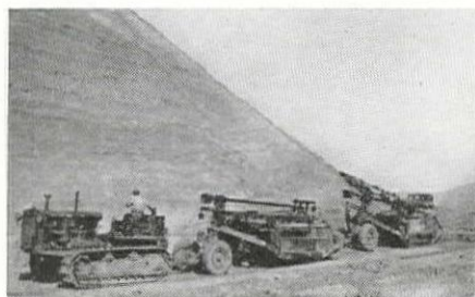
Two LeTourneau 12-yd. Scrapers Used for Making Overhaul.
