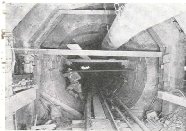
Gunite Lining in Tunnel Near East Portal at Thomas Shaft. Precise Measurement of Diameter Is Being Made by Engineer.
