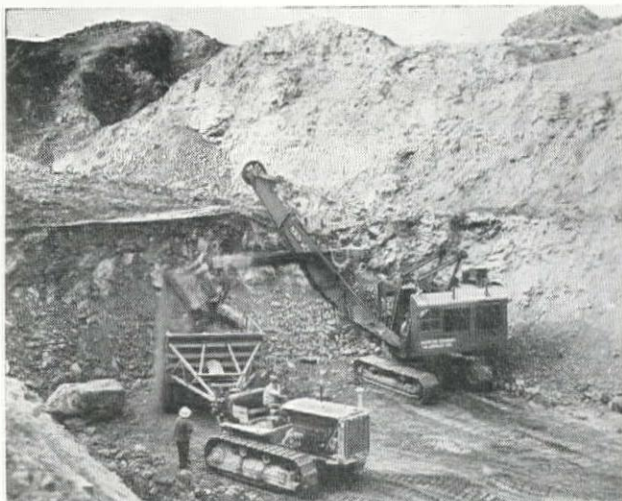
A Tractor Drawn 25-Yd. LeTourneau Wagon and 2-Yd. Northwest Shovel Are Used in the Rock Work on Griffith's Contract.
