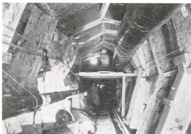
Tunnel Section in Heavy Ground Near Indian Creek Shaft. Note Crushed Condition of Roof Timbers.
