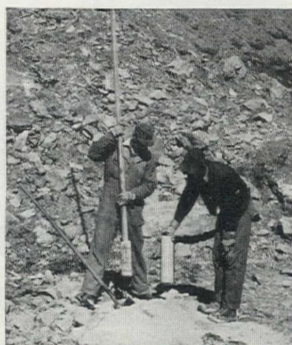
Holes at the center of the cut are loaded with Du Pont "Red Cross Extra" 40%—widely used in blasting operations of this type. It is dependable . . . has considerable water resistance.
