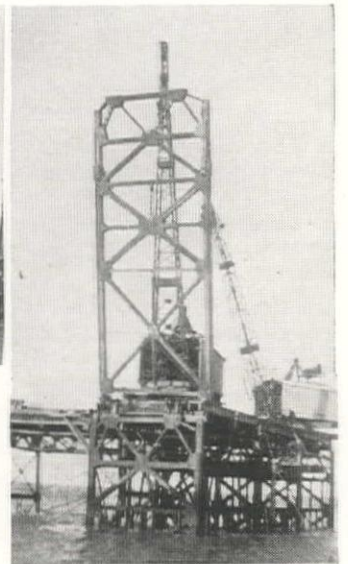
(Upper) Lowering Bottom Section Of AS Unit On Guide Tower, October 25, 1933. Note Jaw Castings And Wooden Blocking To Facilitate Aligning. Three Such Sections Were On Guide Tower At The Time Of Accident One Week Later.
