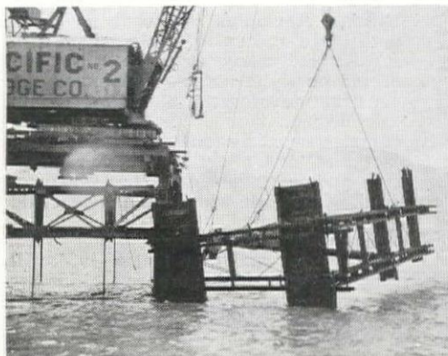
Base Form Being Lowered With Whirley Derrick, June, 1934.
