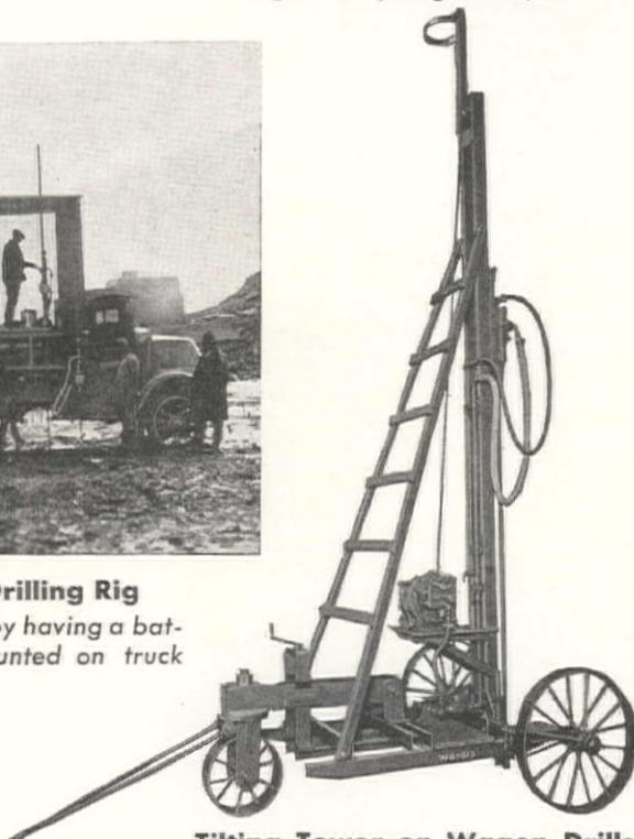
Tilting Tower on Wagon Drills Rapid adjustment to vertical position gets machine at work more quickly
