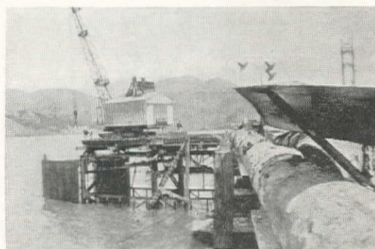
Whirley Derrick Lowering Unit 2CLS, May, 1934. Note Guide Beams Projecting Above Water.
