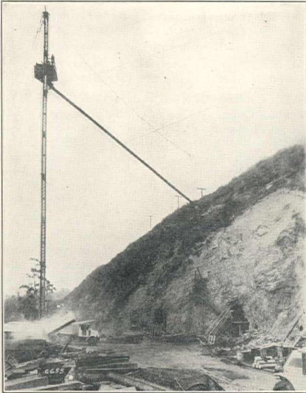
H. W. Rohl & Co. Placing Concrete with Smith-Insley Plant on Figueroa St. Tunnel, Los Angeles
