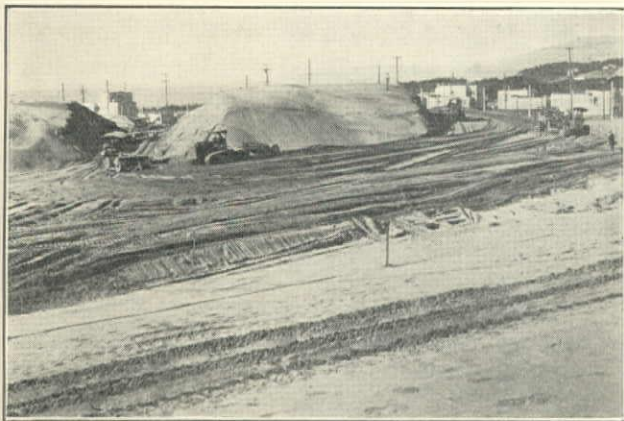
California Construction Co. Grading Sunset Boulevard, San Francisco, with Caterpillar-Drawn Ateco Scrapers and Guy Loaders
