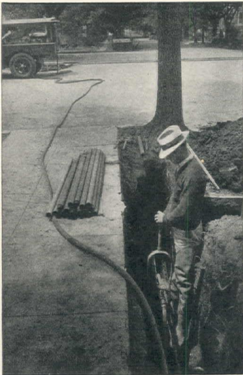
Hydrauger in use—boring under a double street and railroad—a distance of more than 100 feet. This remarkable new tool bores under thoroughfares, sidewalks, buildings, gardens—to lay pipe, condulets, drains and sewers—avoiding pavement-cutting almost entirely.
