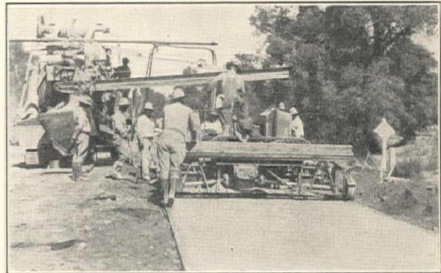
Sander Pearson Laying Concrete with Rex Paver and Lakewood Tampers in San Diego County Between Viejas Creek and Pine Valley
