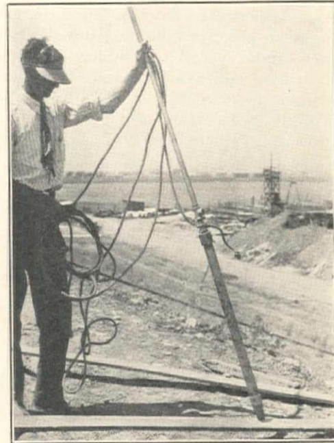
Bottom Sampler for Determining Distribution of Bentonite Seal
