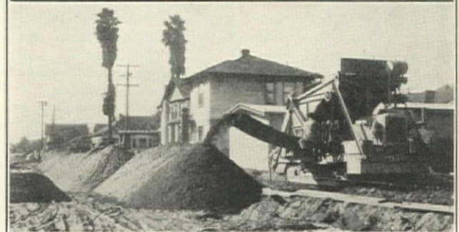
(Upper) Griffith Co. Placing Asphaltic Concrete on Eighth St., Los Angeles, Austin Tandem Roller in Foreground. (Lower) Griffith Co. Excavating with Parsons Trencher on South Broadway, Los Angeles
