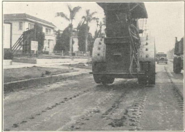
W. F. Crawford Uses Spiked Roller to Perforate Old Asphalt Pavement on Sunset Boulevard, Los Angeles
