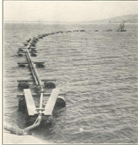
Floating Pipe-Line for Bentonite Suspension with Operating Barge at End
