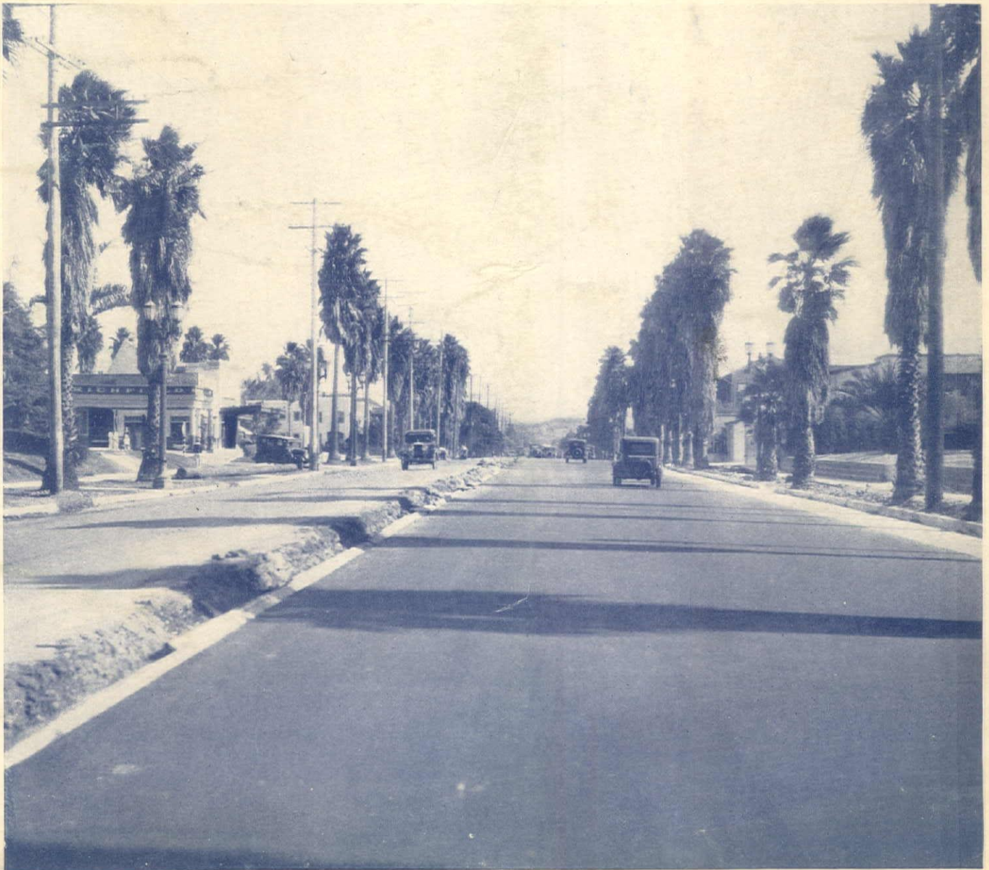
REPAVING OF SUNSET BOULEVARD, LOS ANGELES, EAST FROM HOBART BOULEVARD, SHOWING EXTENT TO WHICH STREET CROWN HAS BEEN LOWERED TO REDUCE CROSS SLOPE; W. F. CRAWFORD, CONTRACTOR
