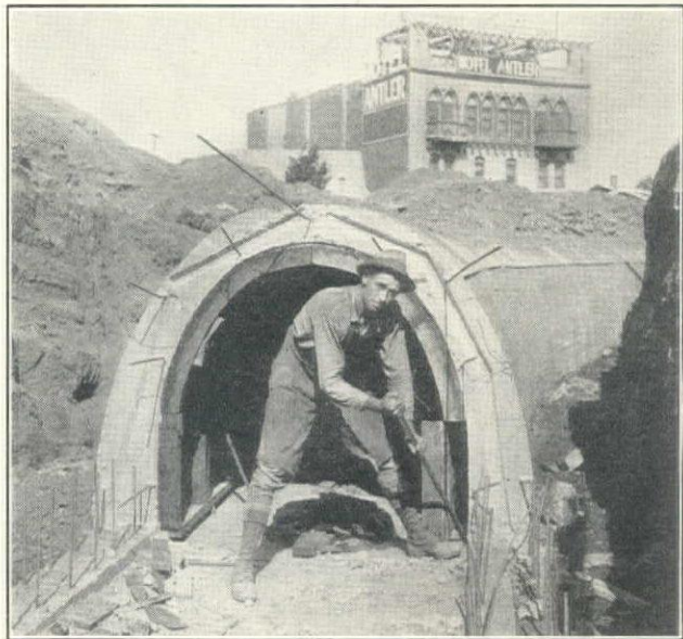
Constructing Semi-Elliptical Concrete Storm Water Drain for Outfall Between Surge Tank and Ocean
