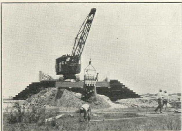
P&H 20-ton Dragline Making Fill on which to Leave West Central Avenue Bridge
