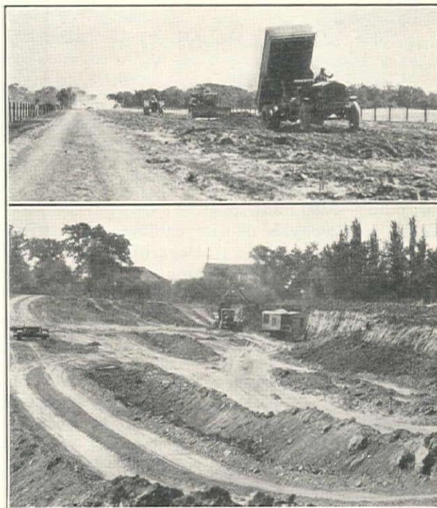
(Upper) Larsen Bros. Grading Between French Camp and Stockton, San Joaquin County, for California Division of Highways. Kleiber 5-ton Truck Dumping in Front of Ateco Bulldozer; Fordson Roller in Background. (Lower) 1 1/4-yd. Brownhoist Shovel in Borrow Pit on Larsen Bros. Contract
