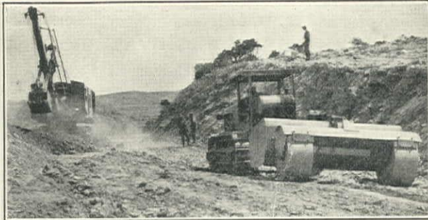
Nevada Rock & Sand Co. Using 1-yd. Northwest Shovel and 2-yd. Ateco Scraper with Caterpillar '60' on White Horse Pass, Elko-Deeth Contract, Nevada Department of Highways, Elko County
