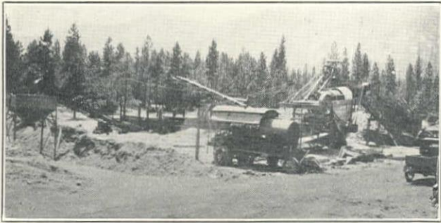
Crushing Plant on Isbell Construction Co. Contract for Sections C and D of Quincy-Beckwith Highway, Plumas National Forest, California
