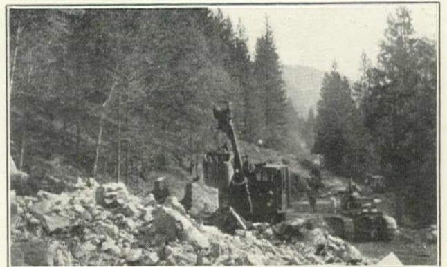
Finnell Co. Working in Rock Cut on Bureau of Public Roads Contract, Riverton-Kyburg Project, Placerville-Lake Tahoe Road, Eldorado National Forest, California. Osgood 1¼-yd. Shovel and Caterpillar '60' in Foreground
