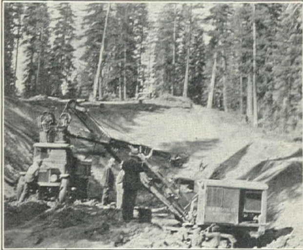
W. A. Bechtel Co., Subcontractor on Northern California Extension of Western Pacific Railroad, Digging in with Northwest 1½-yd. Gas Shovel at Portal for Tunnel. Shovel Loading 5-yd. Sterling Truck
