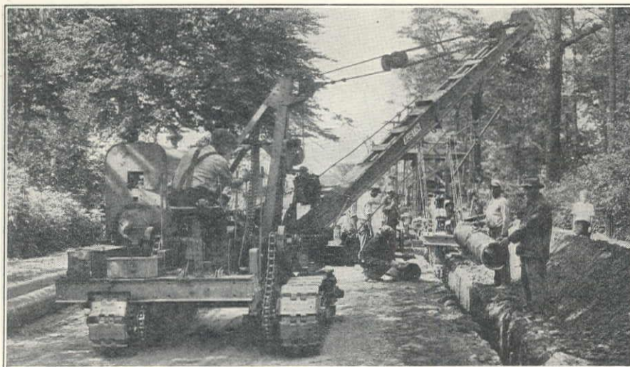
Indianapolis Water Company—laying bell and spigot water mains with Leadite Joints.
