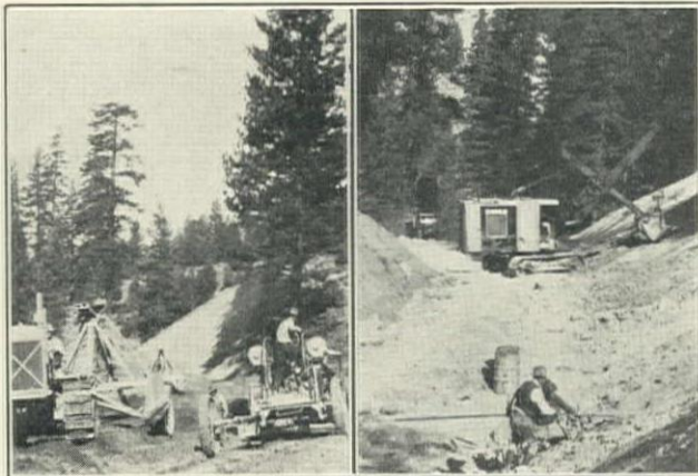
(Left) Trimming Slope with Backstopper Attached to 12-ft. Blade, Chas. Harlowe, Jr., Contract for Blairsdell-Delleker Section, Quincy-Beckwith Highway, Plumas National Forest. Caterpillar '60' and Le Tourneau Scraper Passing Blade. (Right) Bucyrus-Erie 1¼-yd. Gas-Air Shovel on Harlowe Contract
