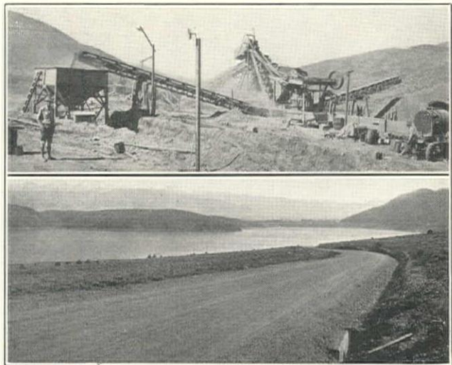
(Upper) Isbell Construction Co. Plant for Surfacing Topaz Highway in Mono National Forest, Nevada. (Lower) Finished Gravel Surfacing on Topaz Highway, Looking Toward Topaz Lake
