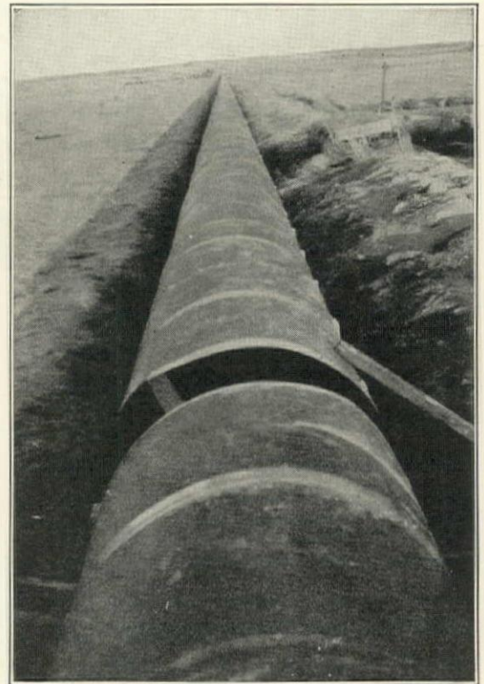
S TRETCHING off into the distant plain is this Armco INGOT IRON syphon installed by the Bigwood Canal Company at Gooding, Idaho. The Western Engineering Company of Seattle, Washington, fabricated the 78" line which is 3600 feet in length made of 300 tons of \frac{3}{8} " Armco INGOT IRON plates. The Syphon serves approximately 7700 acres of land under the Bigwood project.
