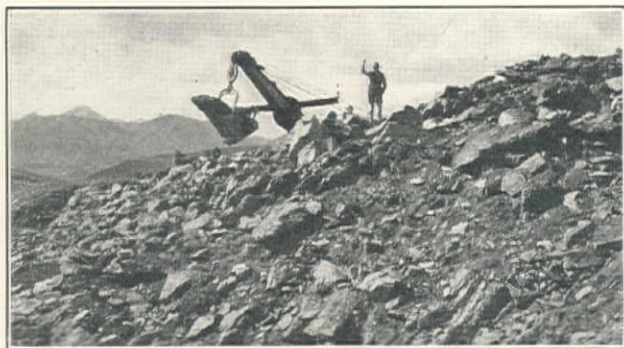
W. A. Colt & Sons 1 1/4-yd. Thew-Lorain Shovel in Rock Cut on Section B of Fall River Project, Rocky Mountain National Park, Colorado, Bureau of Public Roads Contract
