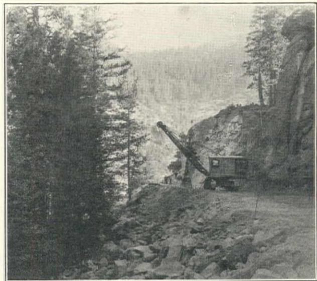
Welsh & Murdock Building Pioneer Road Around Rock Cut on Elevenmile-Grouse Creek Section of Wawona Road, Yosemite National Park, for Bureau of Public Roads
