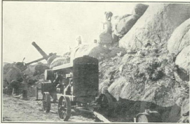
Dimmitt & Taylor Grading Rock Cut on Laguna Highway in Cleveland National Forest, California, Bureau of Public Roads Contract. Ingersoll-Rand Compressor in Foreground
