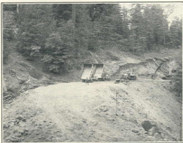
George Pollock Co. \frac{1}{4} -yd. P&H and Fleet of 9-yd. Sterling Trucks Grading Oakhurst Highway in Sierra National Forest, California, Bureau of Public Roads Contract
