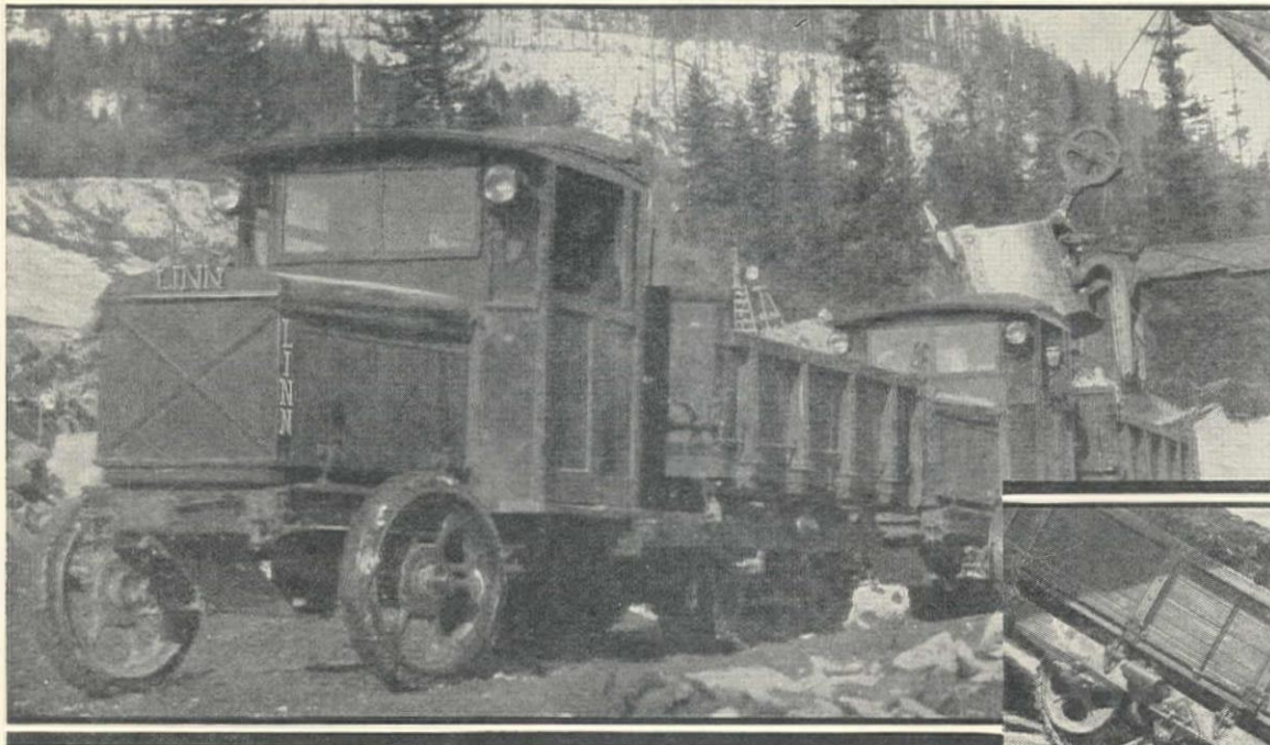
One of a fleet of four Linns purchased by the Phoenix Utility Company for construction work on the Ariel hydroelectric project. The Ariel Dam on Lewis River, Washington, will be 200 feet high and 1,295 feet long. The Linns on this job are equipped with high speed reverse.
