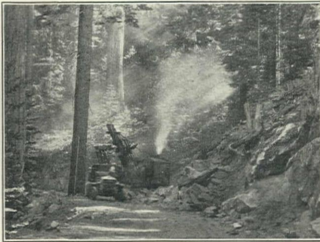
A. J. & J. L. Fairbanks 1-yd. P&H Shovel Loading 5-yd. Sterling Truck on Hospital Rock-Giant Forest Section of the Generals Highway, Sequoia National Park, California, Bureau of Public Roads Contract
