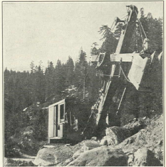
Isbell Construction Co. 1½-yd. Northwest Shovel in Rock Cut on Lake Tahoe Highway, Tahoe National Forest, Nevada, Bureau of Public Roads Contract
