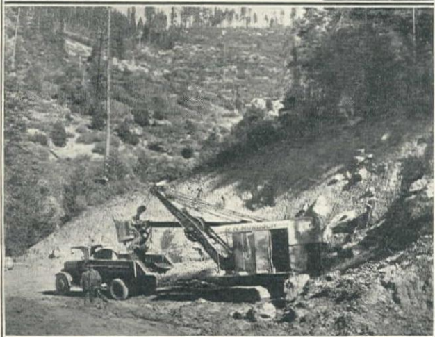
(Upper) George Pollock Co. Grading Mariposa Grove Section, Wawona Road, Yosemite National Park, with Caterpillar '60' and 7½-yd. Le Tourneau Gondola Scraper. (Lower) Welsh & Murdock ¾-yd. Thew-Lorain Shovel Removing Slide on Elevenmile-Grouse Creek Section, Wawona Road, Yosemite National Park
