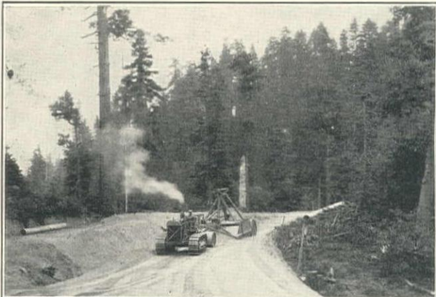
Welsh & Murdock Building Pioneer Road Around Rock Cut on Elevenmile-Grouse Creek Section of Wawona Road, Yosemite National Park, for Bureau of Public Roads
