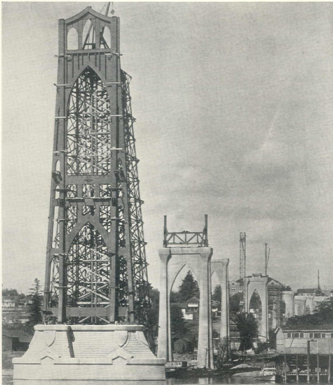
ERECTING MAIN TOWER PIER, ST. JOHNS SUSPENSION BRIDGE, WILLAMETTE RIVER, PORTLAND. TIMBER ERECTION TOWER 100 FT. SQUARE ON BASE, NEARLY 300 FT. HIGH, CONTAINS FOUR HUNDRED THOUSAND F.B.M. AND MOUNTS 60-TON STIFF-LEG DERRICK. J. H. POMEROY & CO. ERECTORS; ROBINSON & STEINMAN CONSULTING ENGINEERS FOR MULTNOMAH COUNTY
