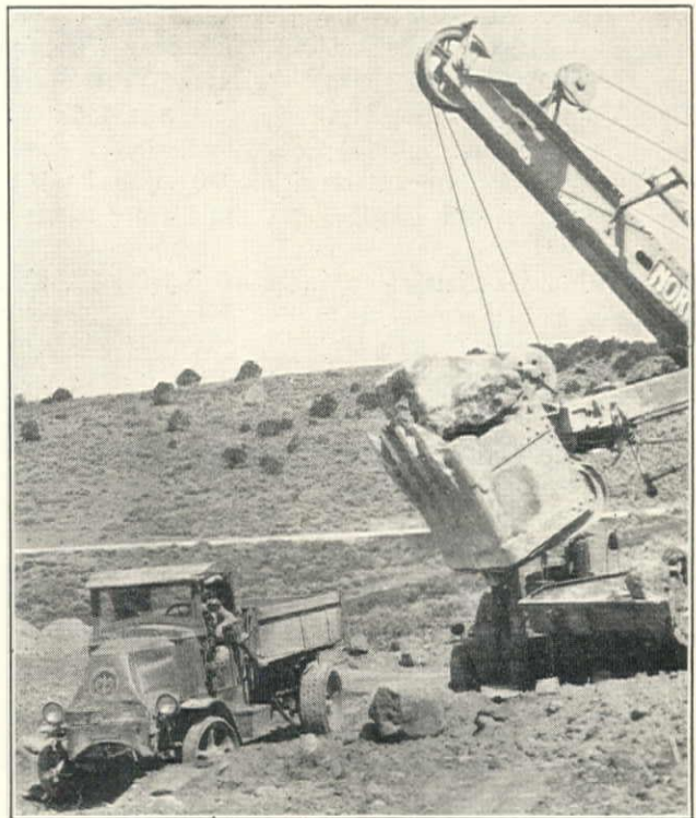
Nevada Rock & Sand Co. 1-yd. Northwest Shovel Loading 6-yd. Mack Truck on Section of Nevada State Highway Between Elko and Deeth
