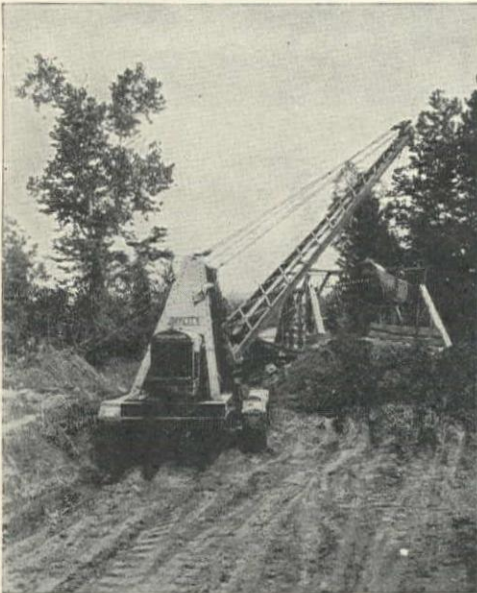
McCormick-Deering Power is operating this shovel, engaged in building approaches to the bridge shown.
