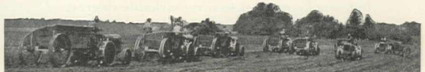
A fleet of McCormick-Deering Industrial Tractors and dump trailers moving dirt quickly and at low cost on a new road in Missouri.
