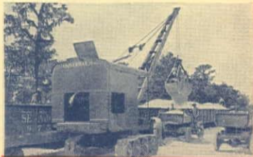
Universal 35, 1/2 yd. machine mounted on 2-Speed Center Drive Crawler.
