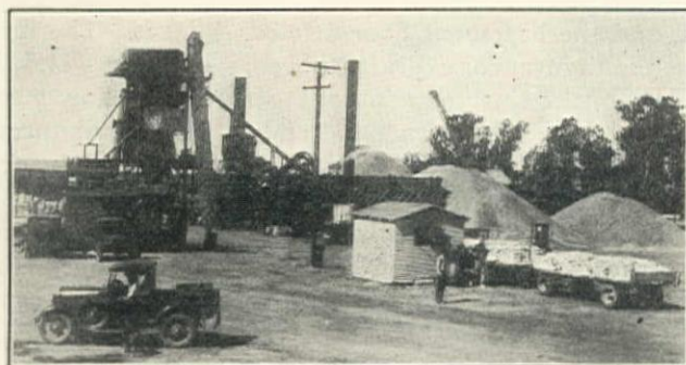
Geiger 4000-lb. Asphalt Plant on Alfacs Siding at Center of Pixley-Tipton Paving Contract of California Construction Co. Northwest Crane with 1-yd. Owens Rehandling Bucket on Stockpile in Right Background
