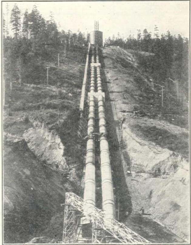
Larner Differential Surge Tank and Twin Penstock for Cushman No. 2 Plant
