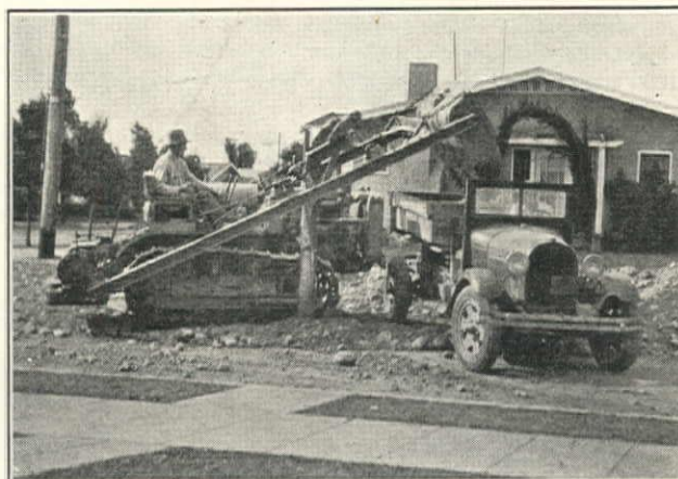
Caterpillar '30' Equipped with Loader on Schedule A, Otay Reservoir-San Diego Second Main Pipe-Line
