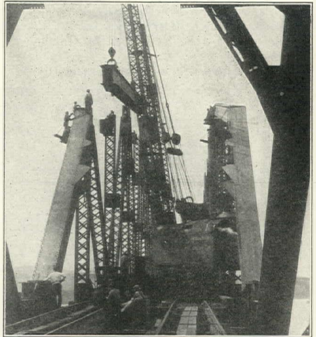
American Bridge Co. Erection Crew Placing Top Chord for Span No. 14
