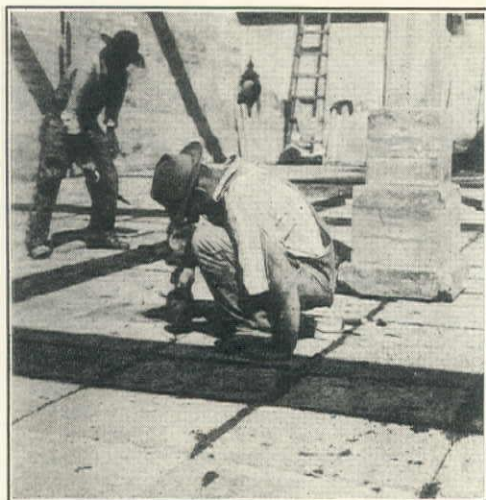
Pouring Portland Cement Grout in Joints Between Porous Concrete Slabs, Watsonville Filtration Plant, Grant L. Miner, Jr., Contractor
