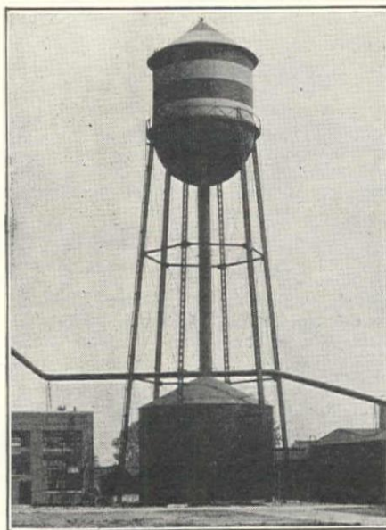
This 200,000-gallon PDM Elevated Tank on a 100-foot tower gives reliable fire protection to the Fisher Body Corporation plant at Seattle, Wash. Ground suction tank is also 200,000-gallon capacity.
