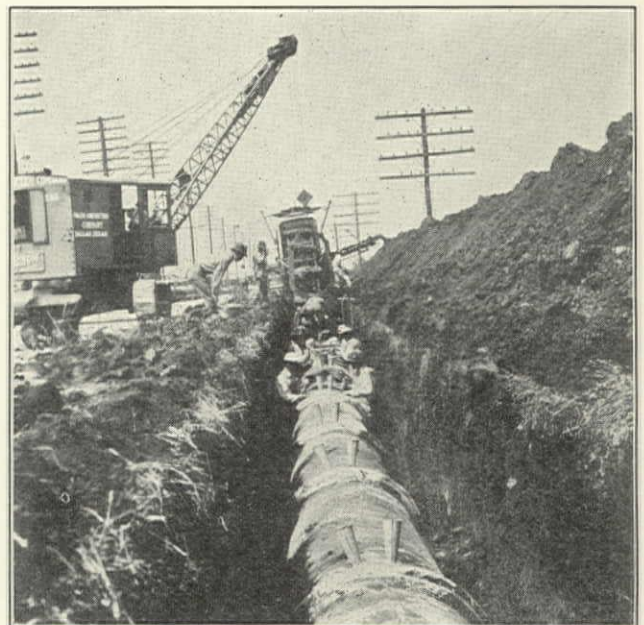
Northwest Crane Laying 36-in. U. S. deLavaud Pipe at Dallas; Leadite Joints Used; Austin Ditcher in Background
