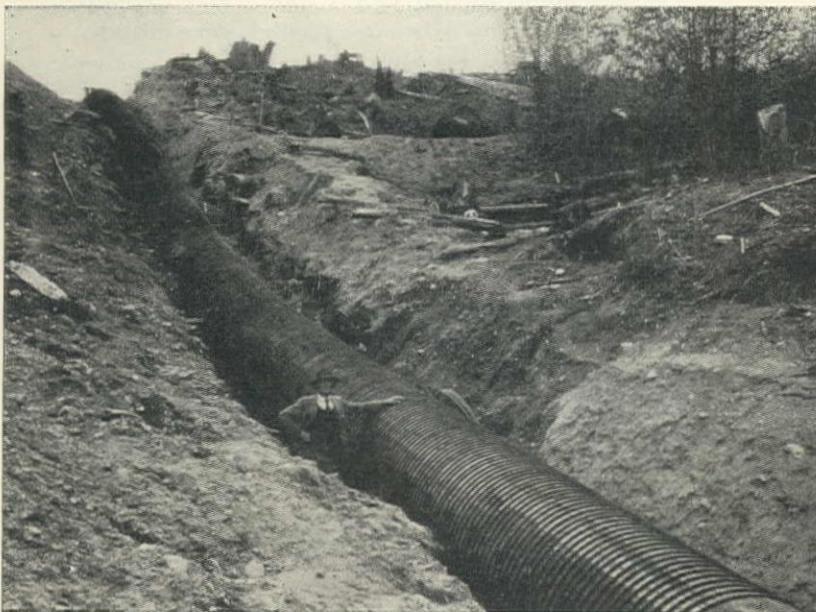
Illustration shows a portion of new Everett water supply line. This line is full of difficult curves, contours and grades, but all obstacles were successfully overcome with Federal Wood Pipe.
