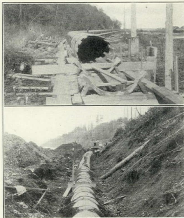
Redwood-Stave Pipe-Line on Trestle and Concrete Pipe-Line in Trench, Elwha River Water Supply
