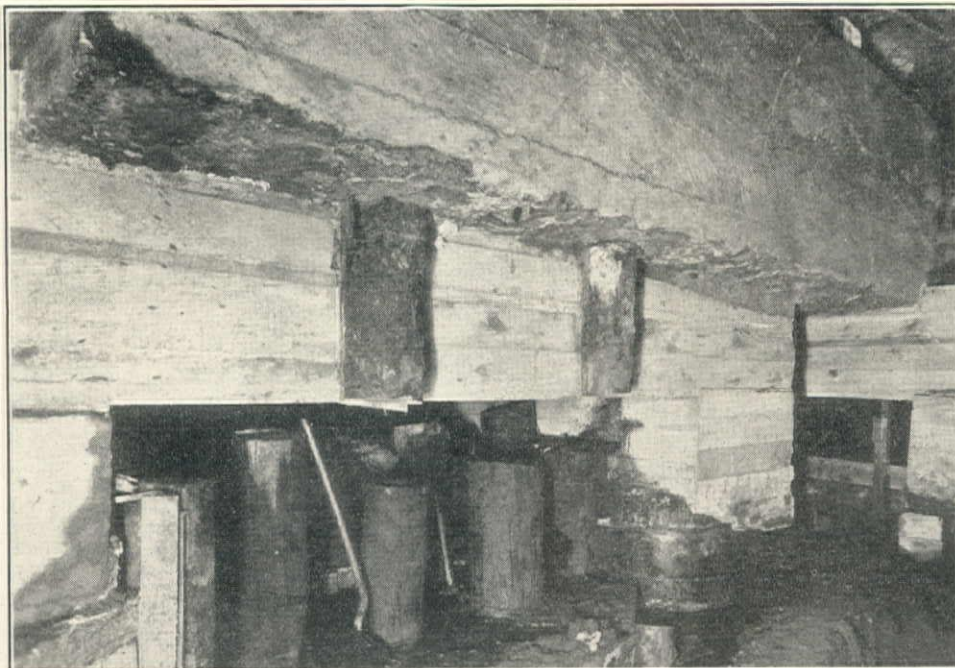
FIG. 7. UNDERPINNING COMPLETED. COMBINED FOOTING SUPPORTS WALL COLUMN AND INTERIOR COLUMN
