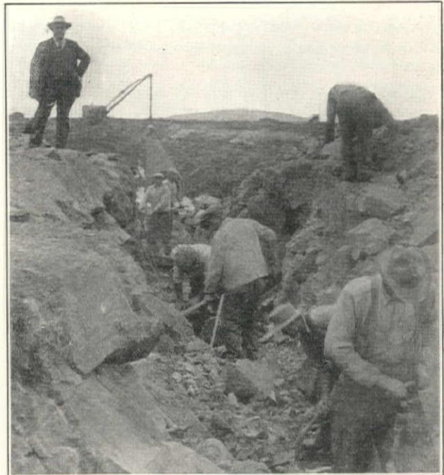
Excavating Trench for North Intercepting Sewer Near S.P. Railroad, Through Sandstone and Bluestone
