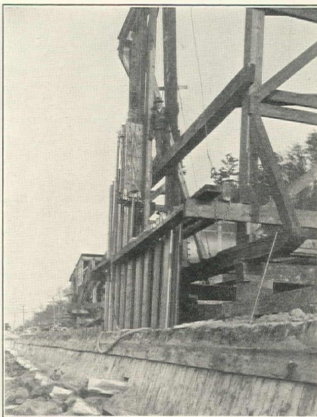
Driving Steel Sheet Piling with McKiernan-Terry Hammer Behind Old Wooden Seawall, Alki Point, Seattle
