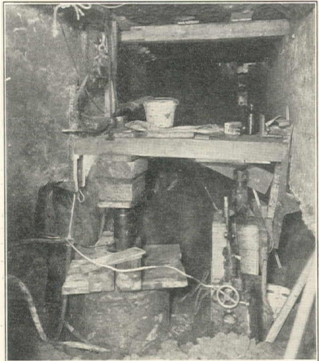
Fig. 8. Hydraulic Jack Forcing Steel Caisson Into Position
