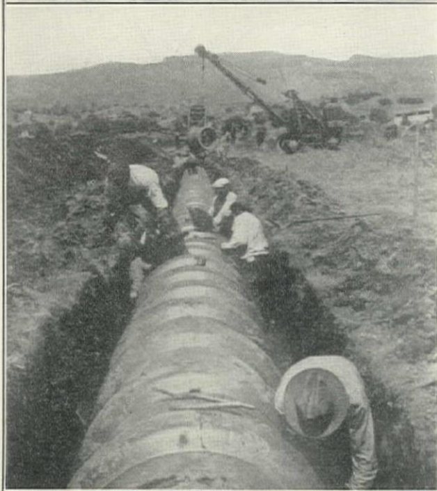
(Upper) P&H \frac{3}{4} -yd. Dragline Excavating Trench for North Intercepting Sewer. (Lower) Laying 36-in. Gladding, McBean & Co. Vitrified Clay Pipe Sewer on North Interceptor East of S.P. Mainline Tracks
