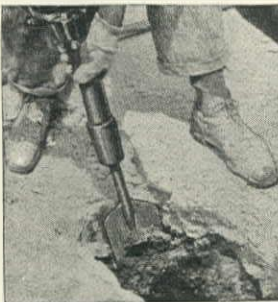
Ability of Spader to dig narrow trench saves pavement replacement costs.
