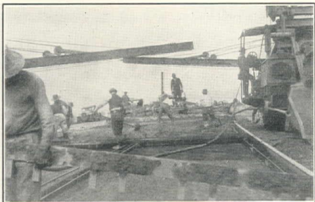
Placing Carey Rubber Joint for Expansion Filler
