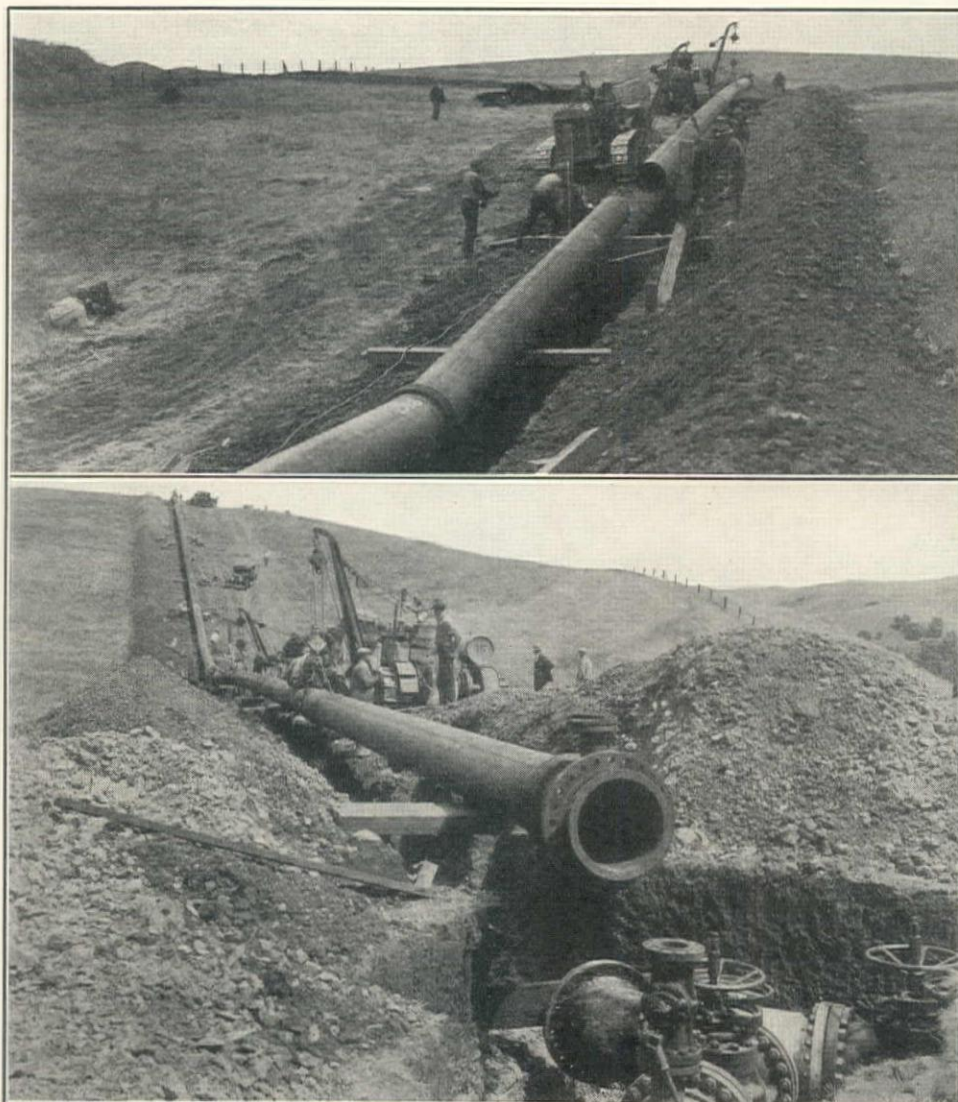
(UPPER) TWO CATERPILLAR '60S' WITH BECHTEL & PALMER BOOMS JOCKEYING PIPE STRING PRELIMINARY TO BELL HOLE WELDING. SMITH WRINKLE BELLY JOINT IN FOREGROUND. (LOWER) PLACING LAST SECTION OF PIPE IN NATURAL GAS LINE NEAR MARTINEZ, VALVE ASSEMBLY FOR WYE BRANCH IN FOREGROUND
