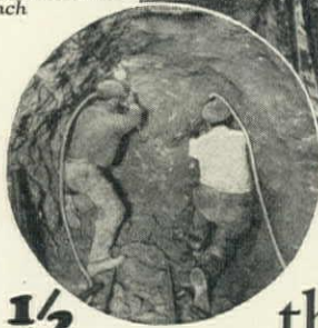
At Left—Bull point Spaders drive sewer tunnel rapidly in dry clay.
