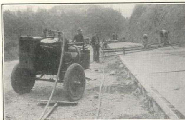
I. L. Young Construction Co. Applying 'Hunt Process' for Curing Pavement on the Canyon Road
