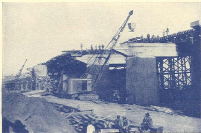
P & H Model 400 placing concrete on Commerce Street viaduct job.
