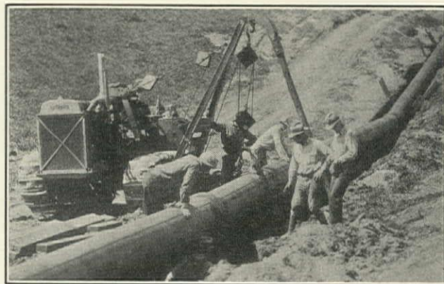
Caterpillar '60' with Bechtel & Palmer Boom and Rope Sling Lowering Welded Pipe into Trench. Note Use of Removable Telescopic Tripod Leg with Side Boom
