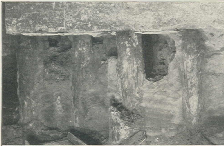
FIG. 1. DRY-ROTTED AND BROKEN PILES BENEATH OLD FOOTINGS OF SAN FRANCISCO OFFICE BUILDING
